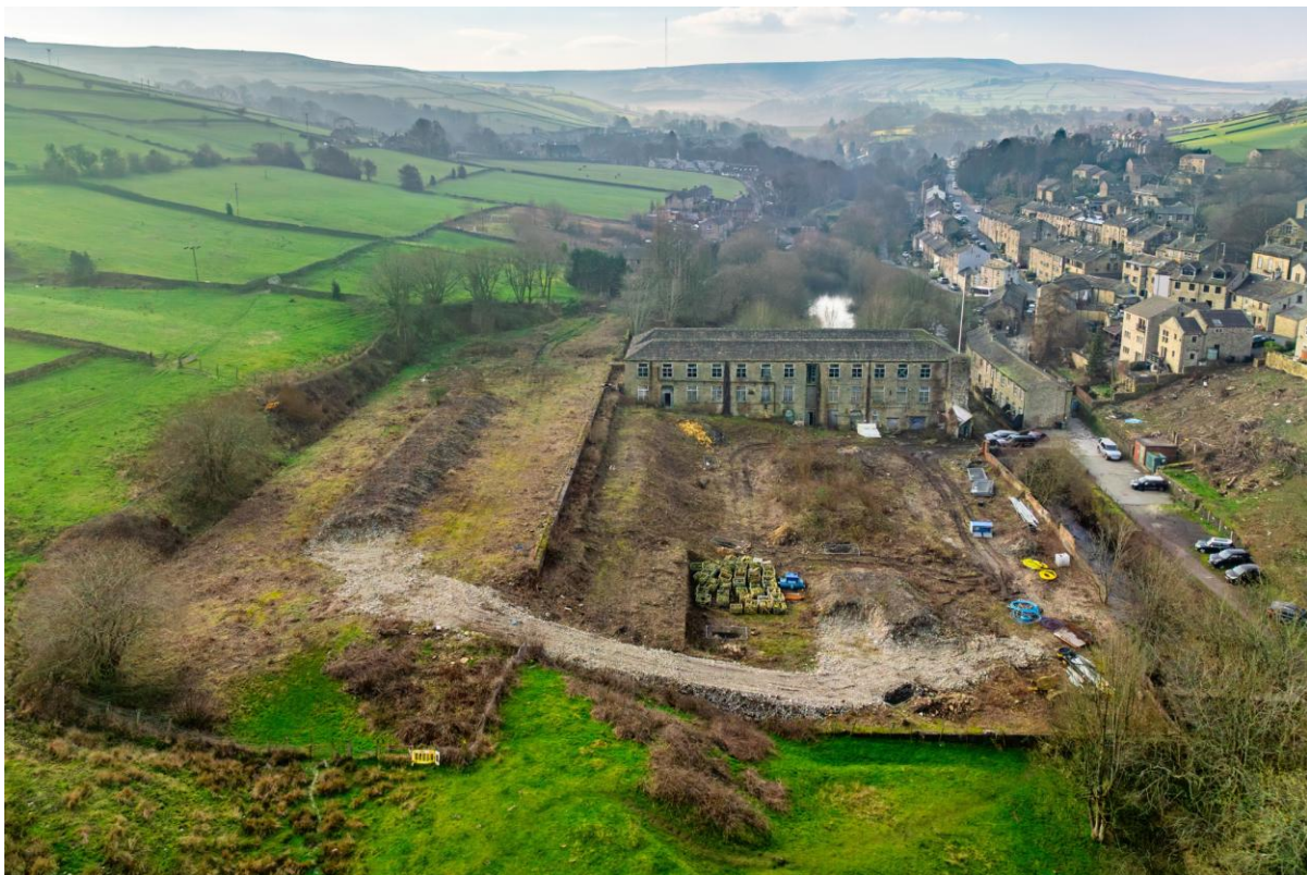
Site following demolition of the former industrial buildings, before the current redevelopment works.
