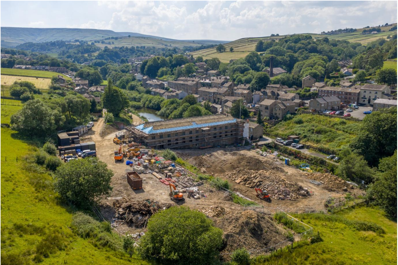
Current redevelopment works with the retained mill remaining as the principal historic building on the site.
