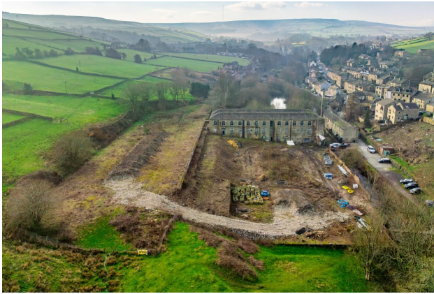
Site following demolition of the former industrial buildings, with the retained mill at the centre.
