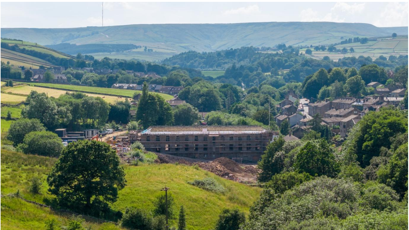
View toward the retained mill from the northern landscape. The amended northern plots have been designed with this relationship in mind.
