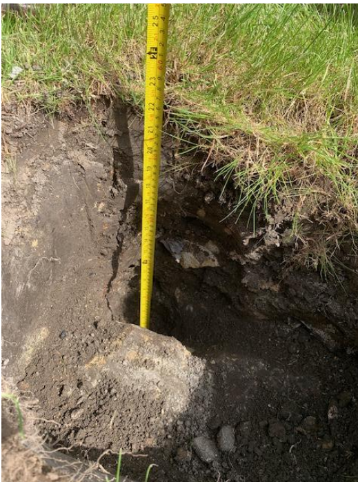
Excavation in garden 4/6
