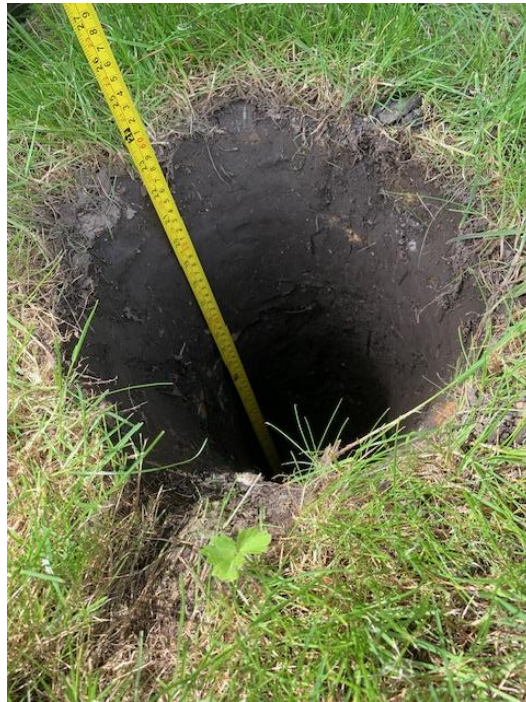
600 mm depth of excavation
