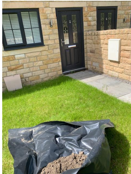
Material excavated from garden 8/10
