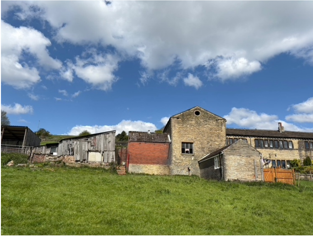
South east elevation / external building
