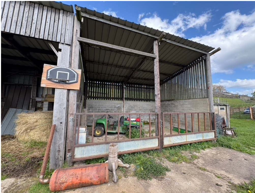
End bays of agricultural structures (to be demolished)
