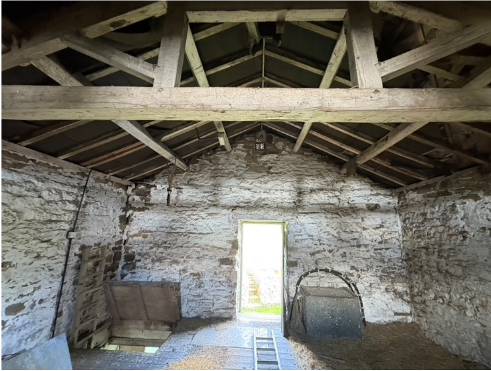
Internal photo at first floor towards north west
