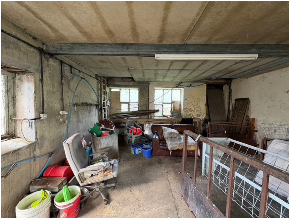
Internal photo at ground floor towards north west
