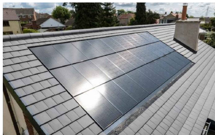
Recessed Solar Panels Scale NTS
