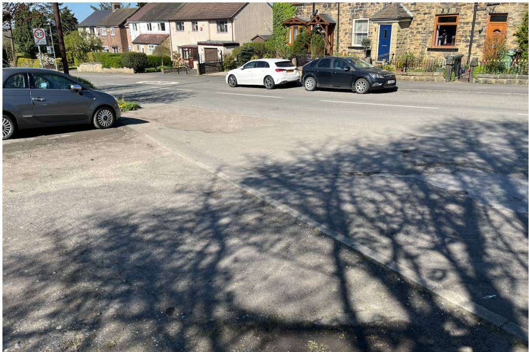
Figure 2 Photograph of existing drainage channel position
