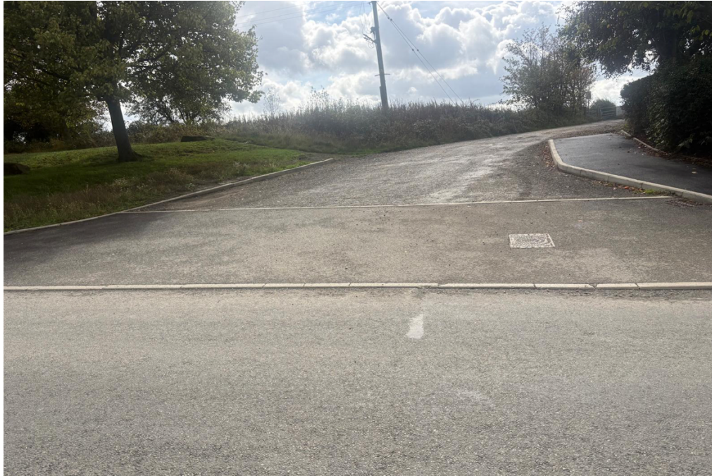
Figure 5 Photograph initial access improvement works (looking southeast)
