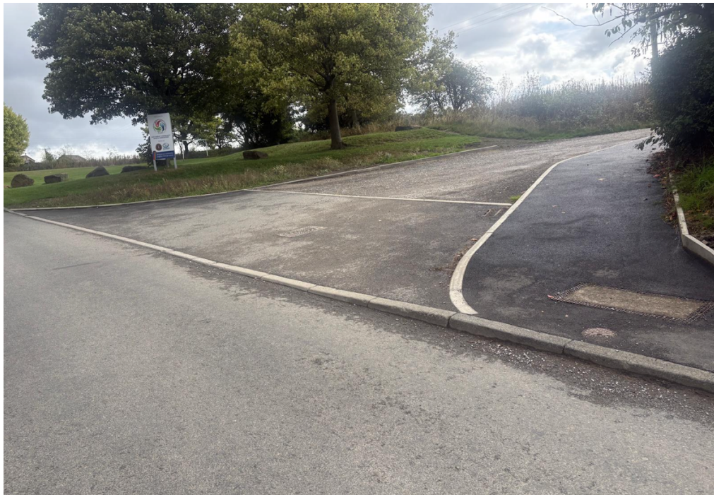
Figure 6 Photograph initial access improvement scheme (looking east)
