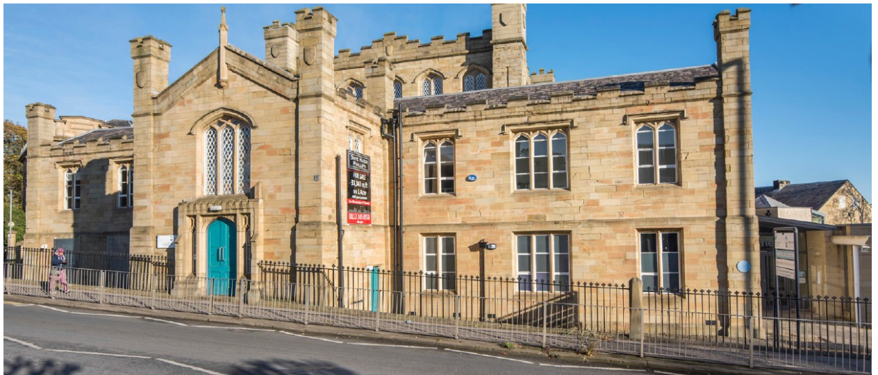
Current view from New North Road (with The Link Building to the right).
