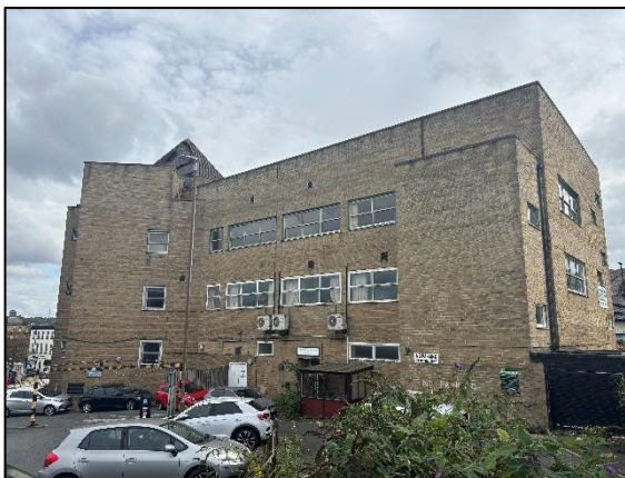
Buildings B1 and car park (u1b5 u1b 804)
