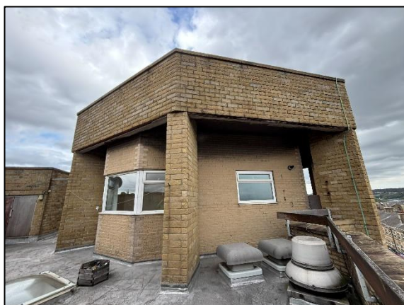
Eastern elevation of residential dwelling
