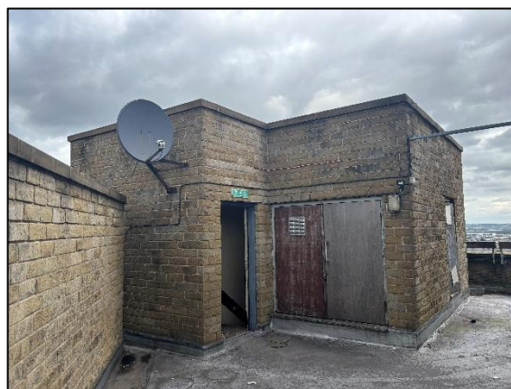
Storage building and stairs
