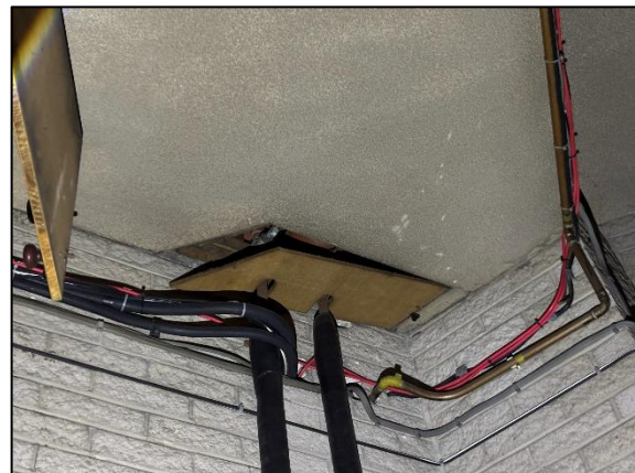
Small gap from lifted board adjacent to butterflies
