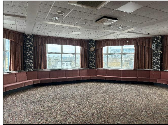
Second floor interior of B1
