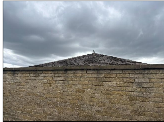
Roof tiles of main hipped roof
