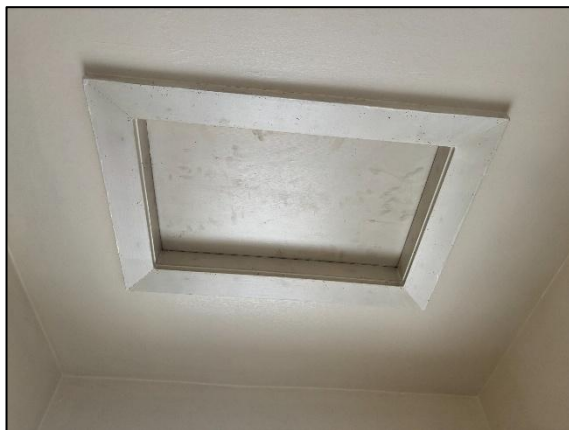
Inaccessible loft hatch leading to loft 1
