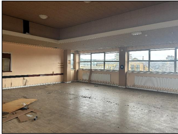
Third floor interior of B1
