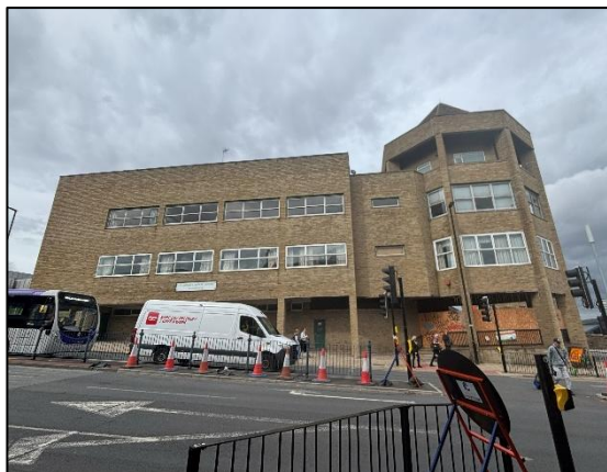
Building B1 (u1b5)
