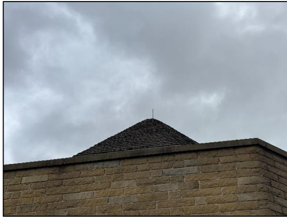
Roof tiles of residential dwelling
