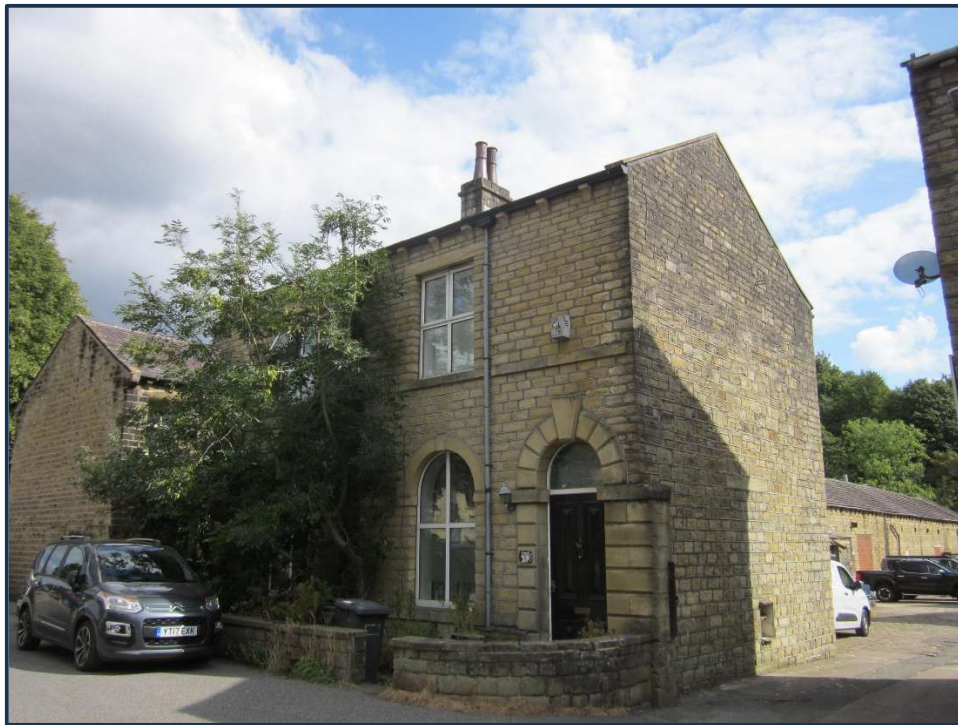
Photograph 5. 4 and 5 Commercial Mill Cottages (looking South West)
