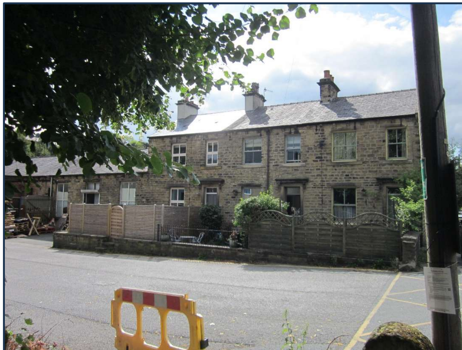
Photograph 4. 1 – 3 Commercial Mill Cottages (looking South West)
