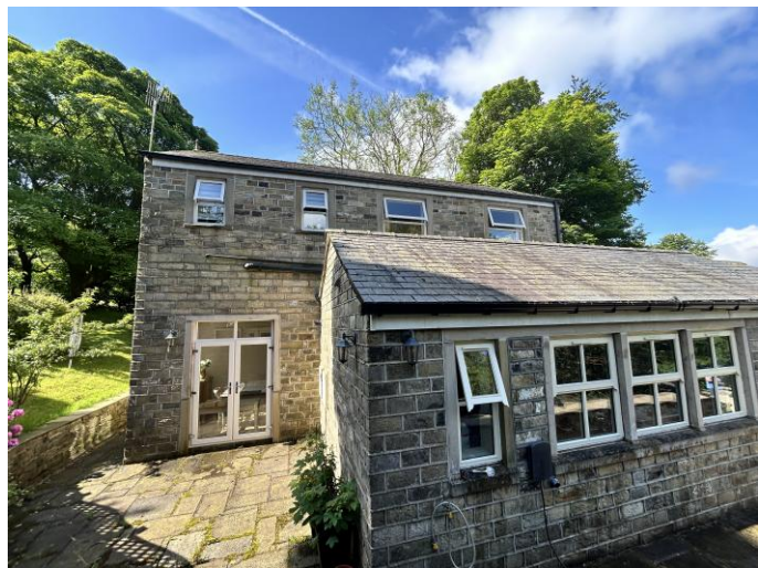
North facing façade [site visit]
