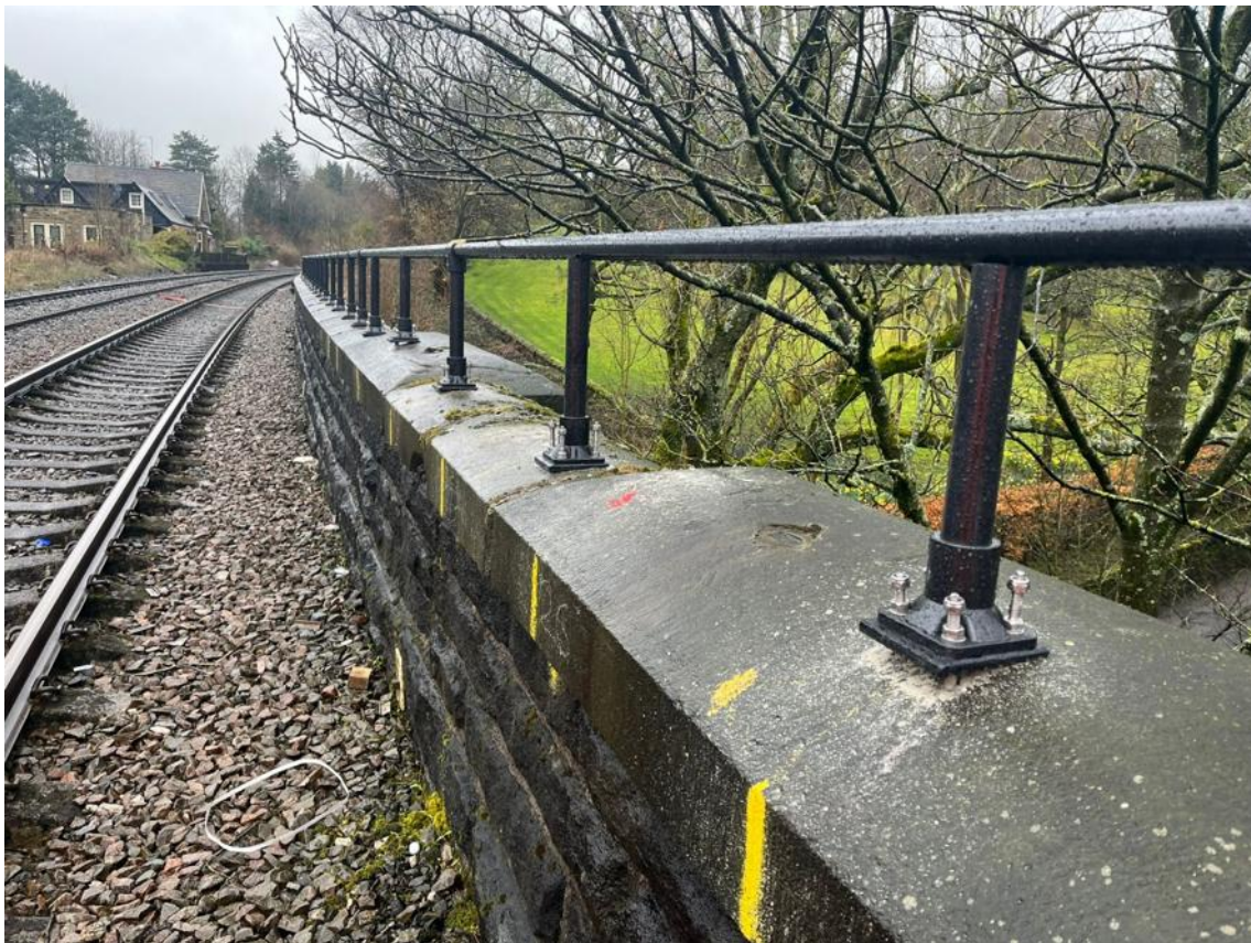
Figure 1 - Indicative image of new black GRP handrail.
