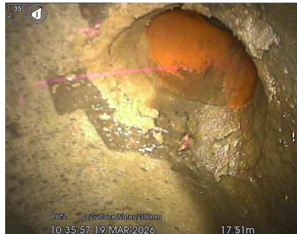
4, 00:01:38, 17.12 m Junction at 3 o'clock, 100mm dia
