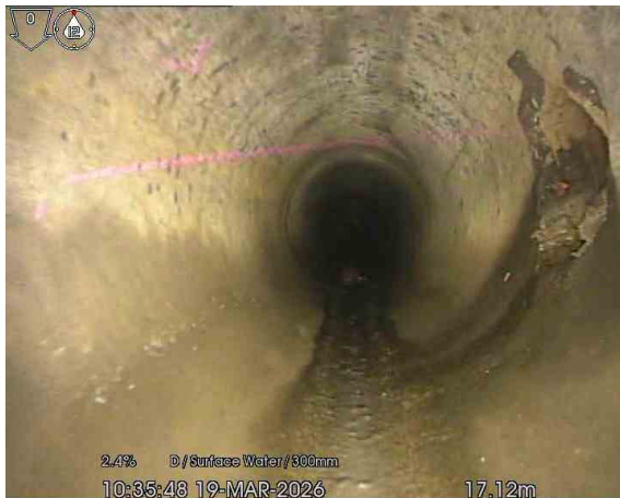
3, 00:01:38, 17.12 m Junction at 3 o'clock, 100mm dia
