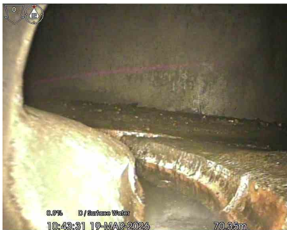
1, 00:05:24, 70.35 m General photograph taken at this point, PIPE ENTERING CHAMBER
