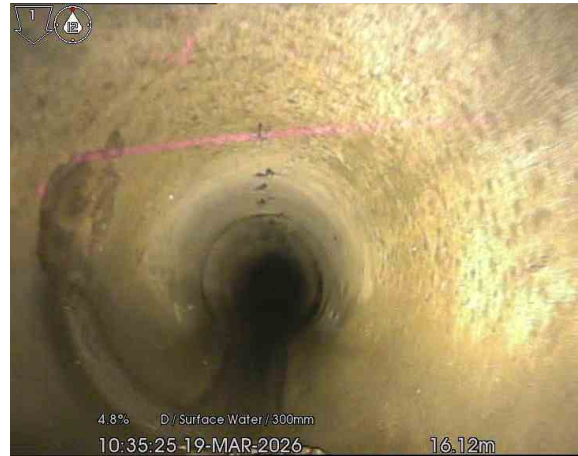
2, 00:01:15, 16.12 m Junction at 9 o'clock, 100mm dia
