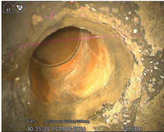
1, 00:01:15, 16.12 m Junction at 9 o'clock, 100mm dia
