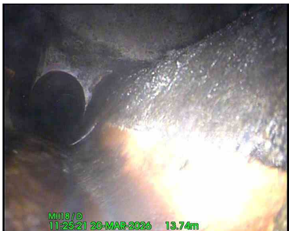
1, 00:01:06, 13.74 m Finish node, manhole, reference: OS8X
