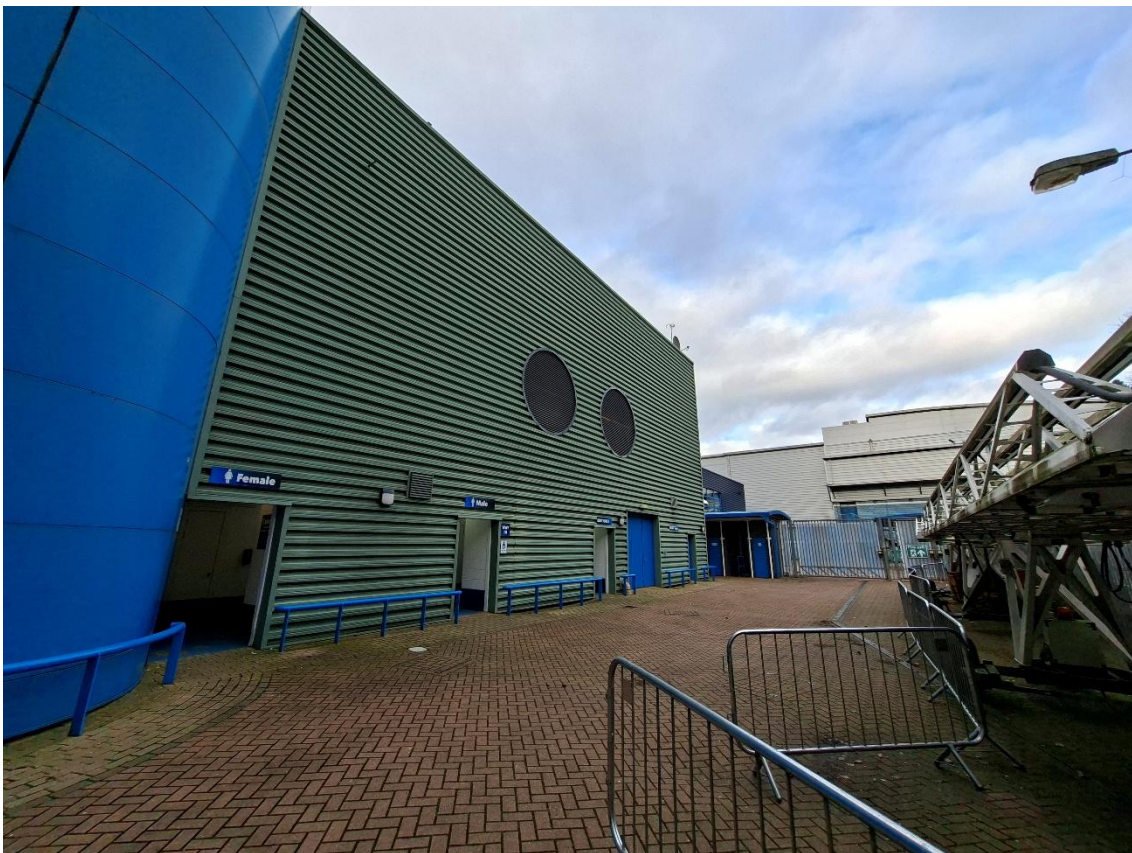
4. Looking north at the southern elevation of the leisure / office structure.
