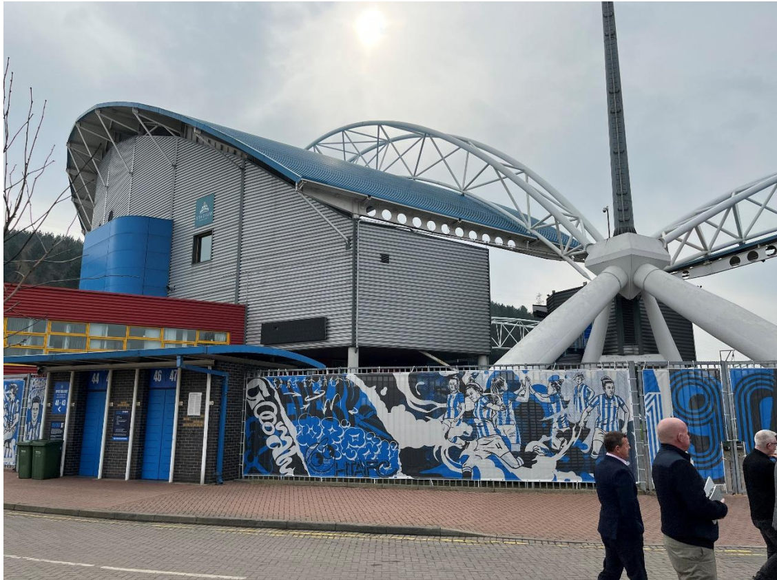
1. Looking south at the northern elevation of the North Stand.
