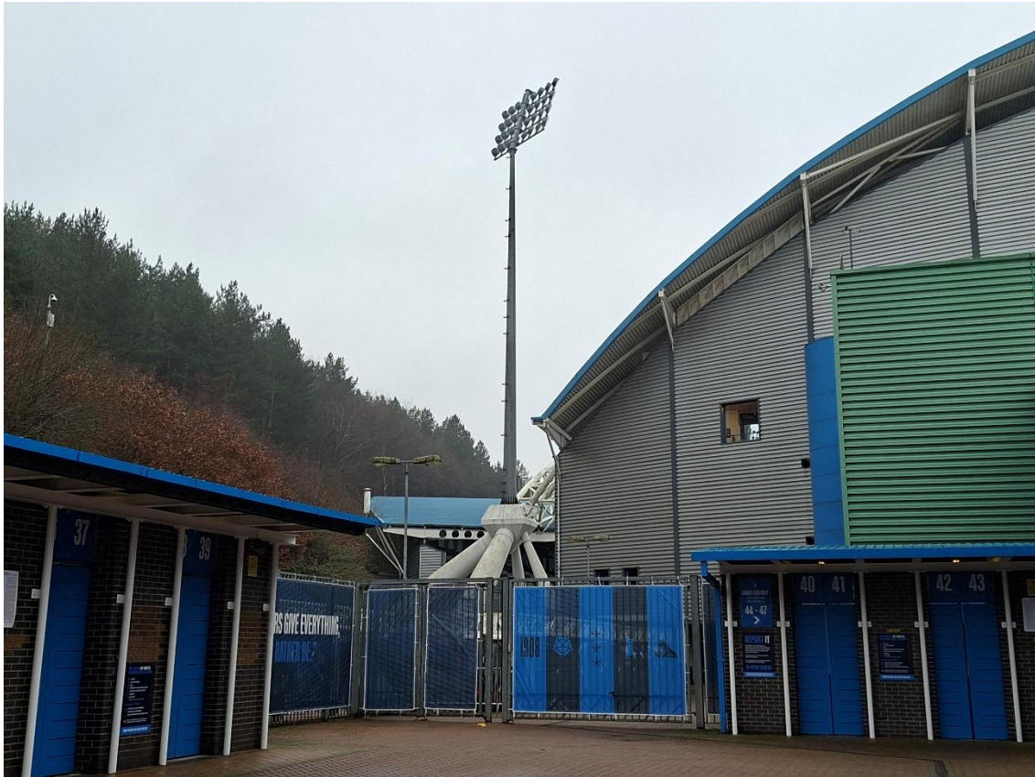
3. Looking south west at the south of the North Stand and leisure / office structure.
