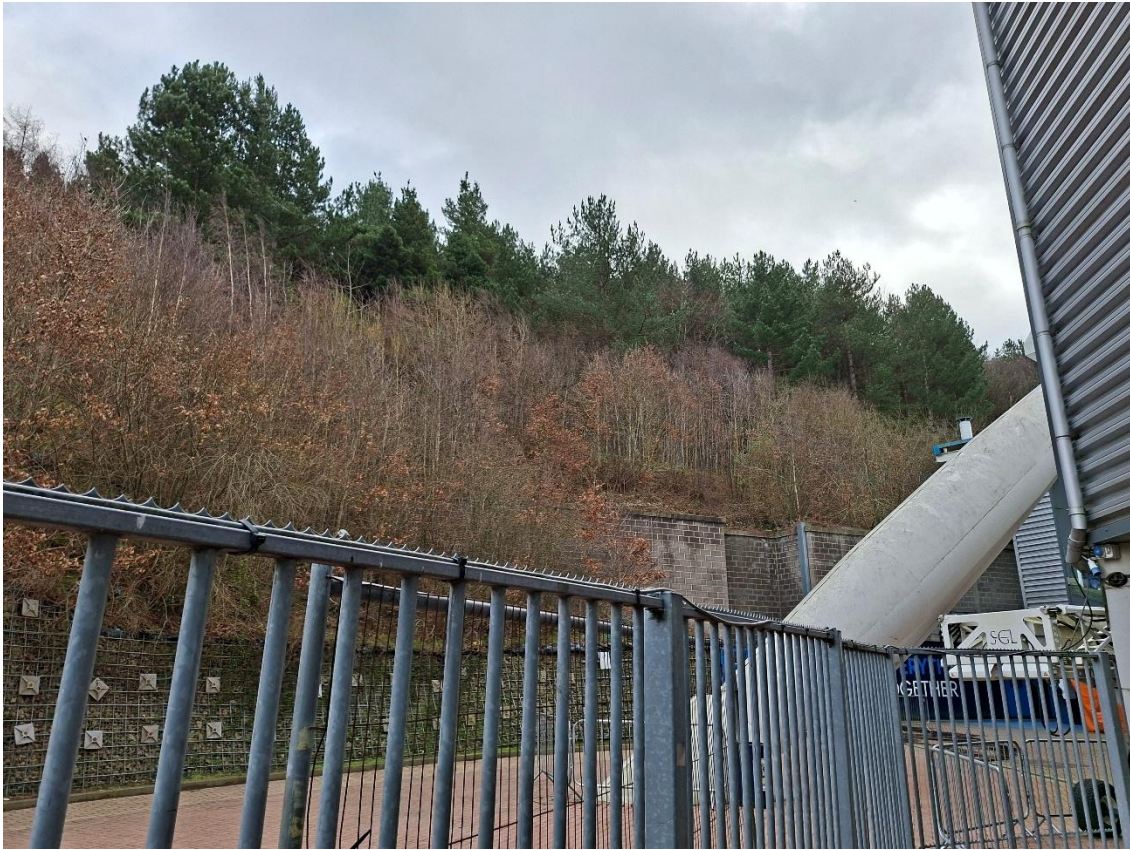
5. Embankment to the east of the site.
