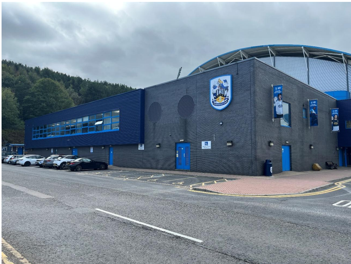
2. Looking south at the north and east elevations of the leisure / office structure.
