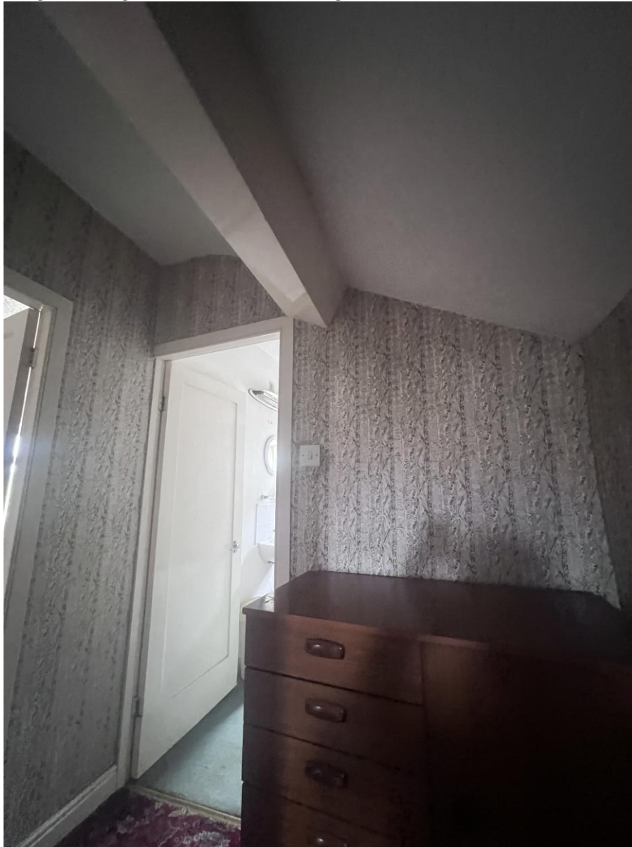
Image showing internal headroom along rear wall (1.76m)
