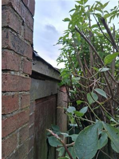
Plate 21 - View of Building 2
