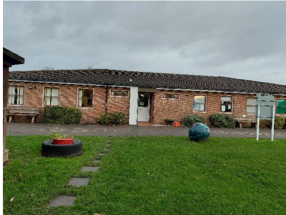
Plate 14 – Southern aspect of Building EFAA
