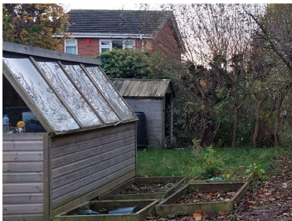
Plate 23 – View of Building 5 and 6.
