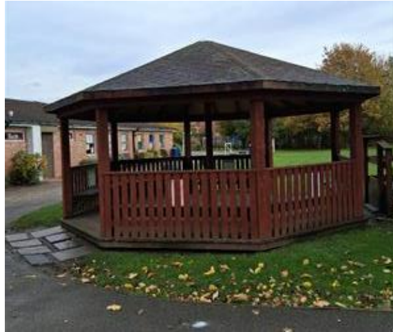
Plate 20 – View of Building 1.
