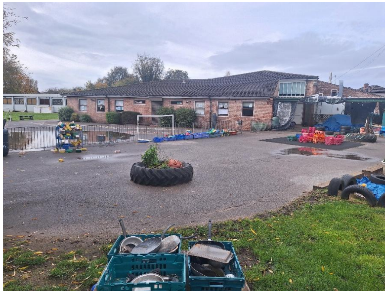
Plate 4 – Example of area of developed land sealed surface within the site boundary.
