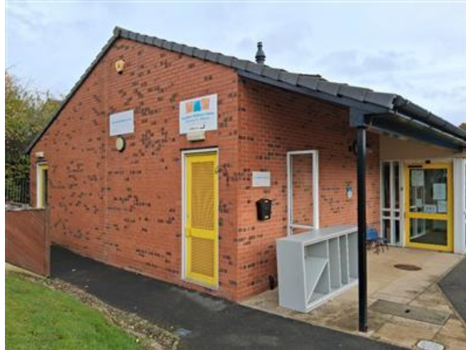
Plate 17 – Southern and eastern aspect of Surestart Children's Centre
