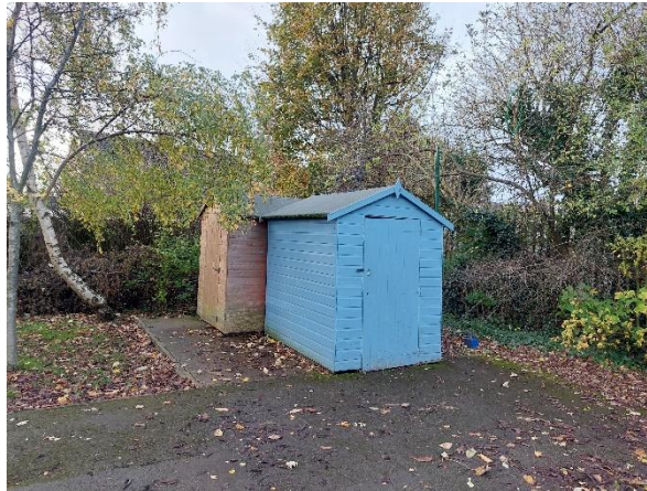
Plate 22 – View of Building 3 and 4
