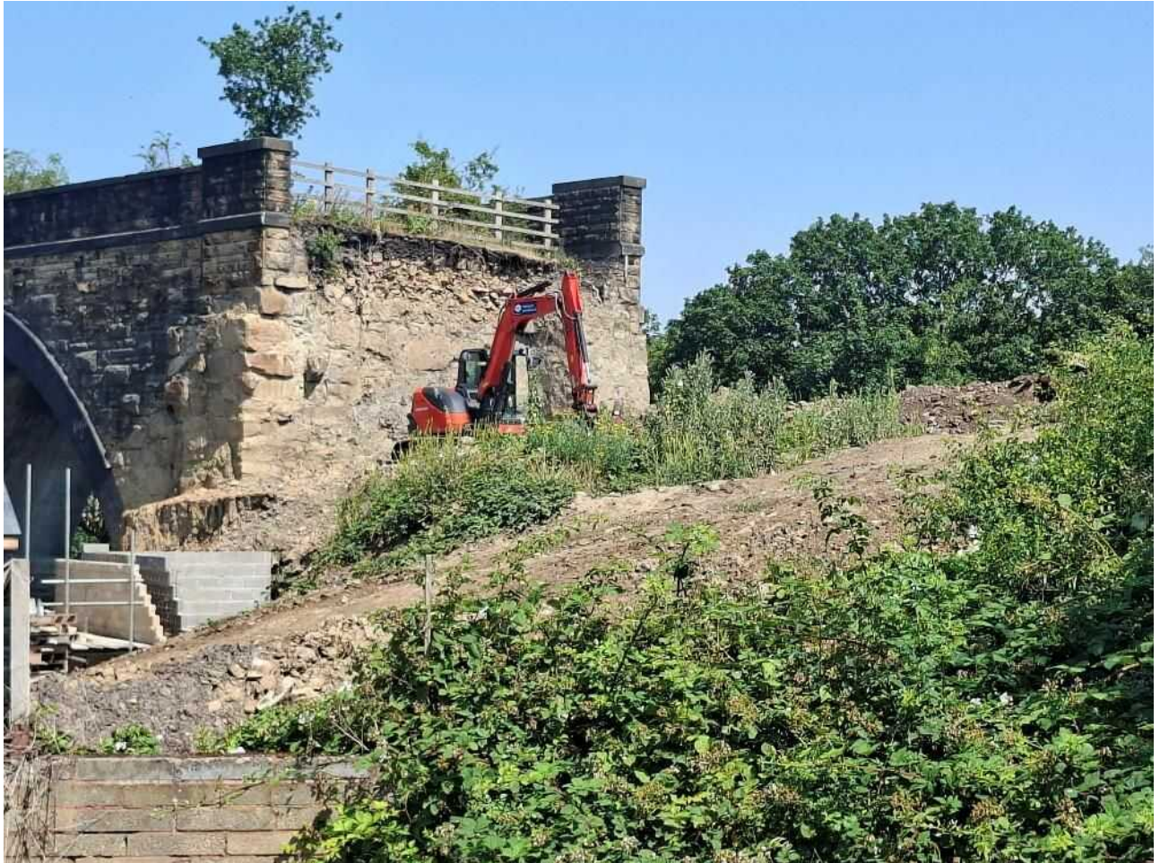
Photograph 2 – View north-west of the Site towards former railway bridge and associated groundworks, that was a continuation of the raise railway line that ran near the Site's north-western boundary – illustrating the nature of the material recently excavated from the embankment (rock fill) present along the temporary access slope.
