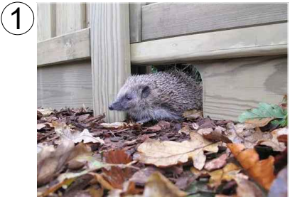
Hedgehog Holes 13cm x 13cm holes cut into the base of fencing panels.
