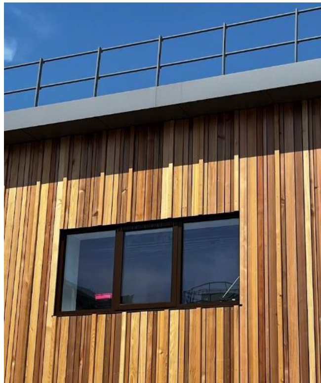
Cedar Cladding currently being installed on the recladding of a storage shed else where on the Longley site. Used here in conjunction with aluminium windows, aluminium ppc eaves cladding and aluminium roof handrail, all as proposed on the proposed development
