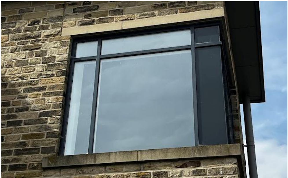
Aluminium Curtain Walling and Windows Smarts Architectural Aluminium Alitherm 700 series with double glaze sealed units to achieve a ‘U’ value of 1.6w/m2k.
