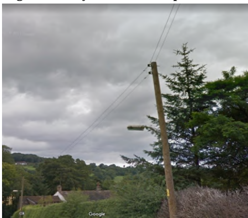
Figure 5 & 6 Open wire LV cable replaced with design successor Aerial Bunch Conductor
