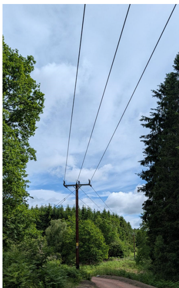
Figure 2 – 100mm Alloy conductors -proposed replacement
