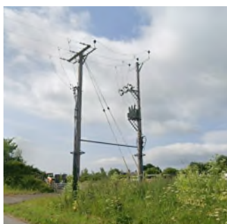
Figure 3 – Lay Pole terminal pole
