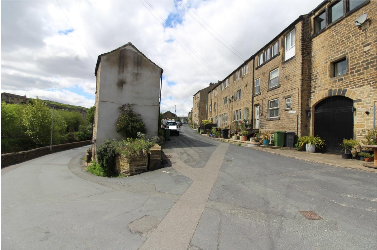
Plate 7 – View along Old Road / Ford Gate
