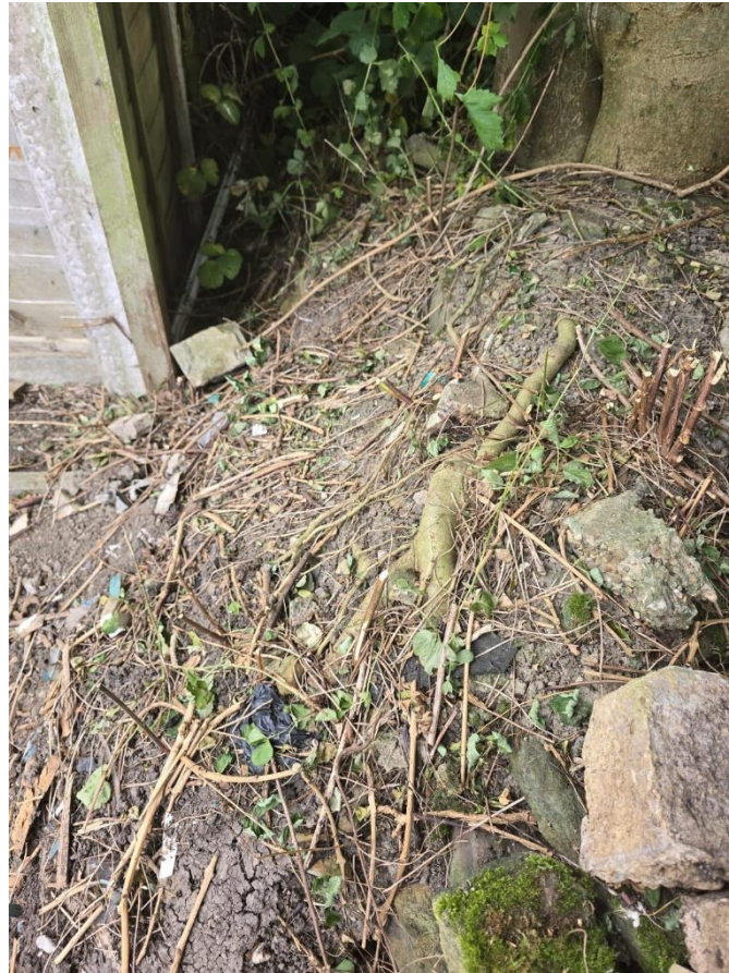
Image 6 - Showing tree roots overgrowing the dry-stone wall and subsiding over / impacting fence location
