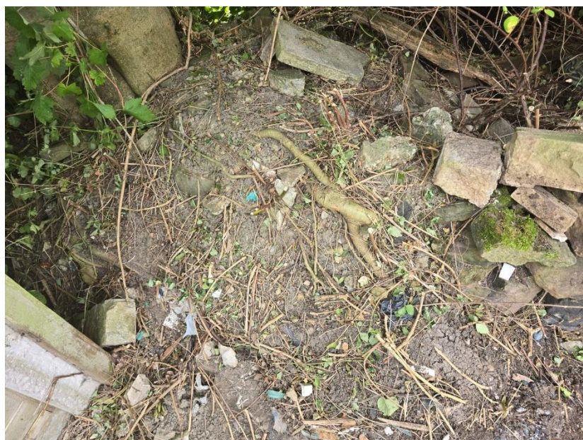
Image 6 - Showing tree roots overgrowing the dry-stone wall and subsiding over / impacting fence location
