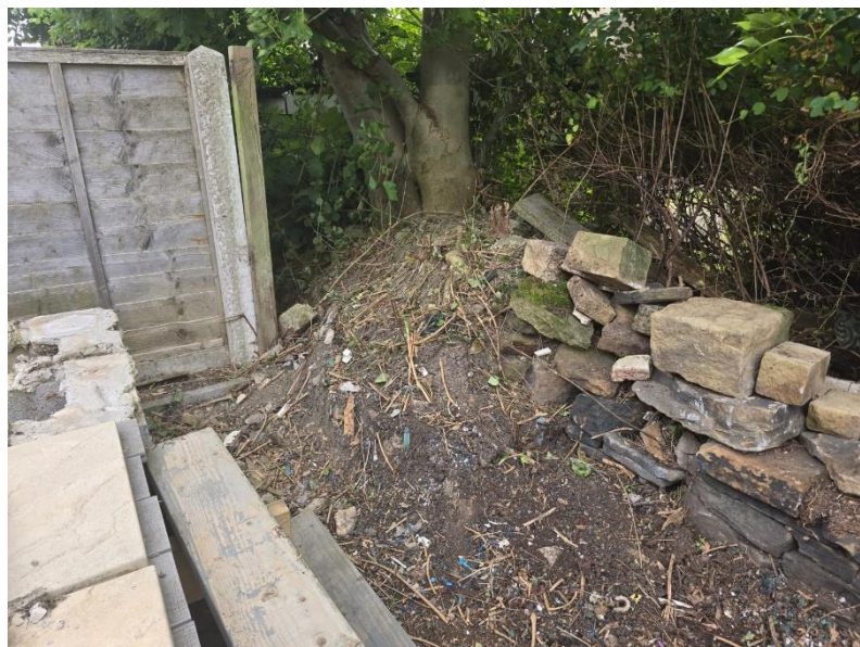
Image 4 - Showing tree roots overgrowing the dry-stone wall and subsiding over / impacting fence location
