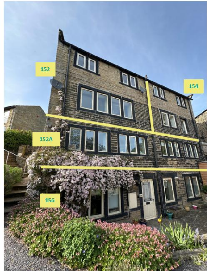
Rear of property, showing split of units
