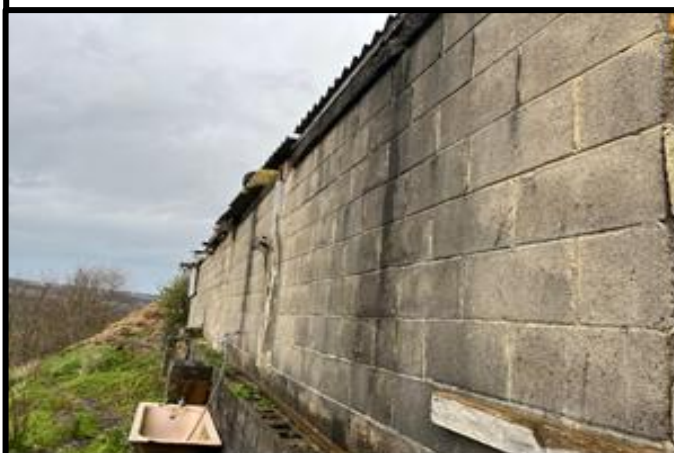
Photograph 5. View of stable from behind.
