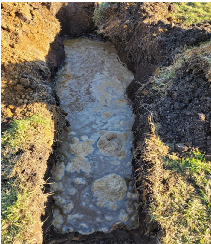
Typical soakaway test
