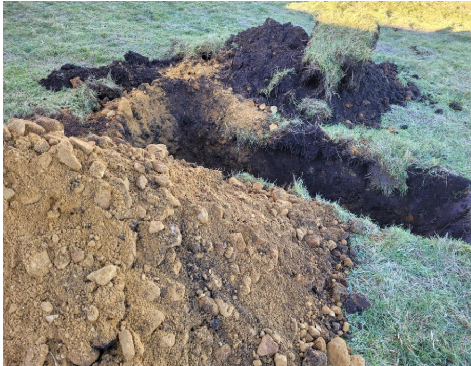
Typical arisings from trial pits
