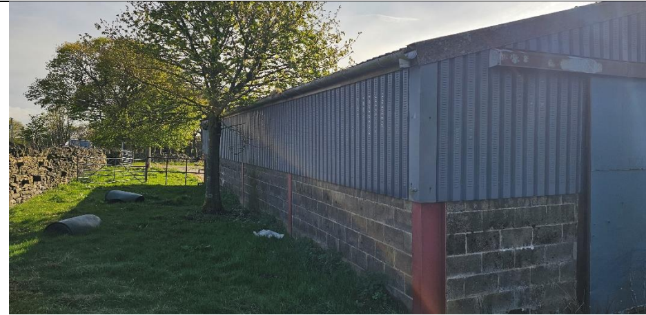
Photograph 11: Northern aspect of Building 1.
