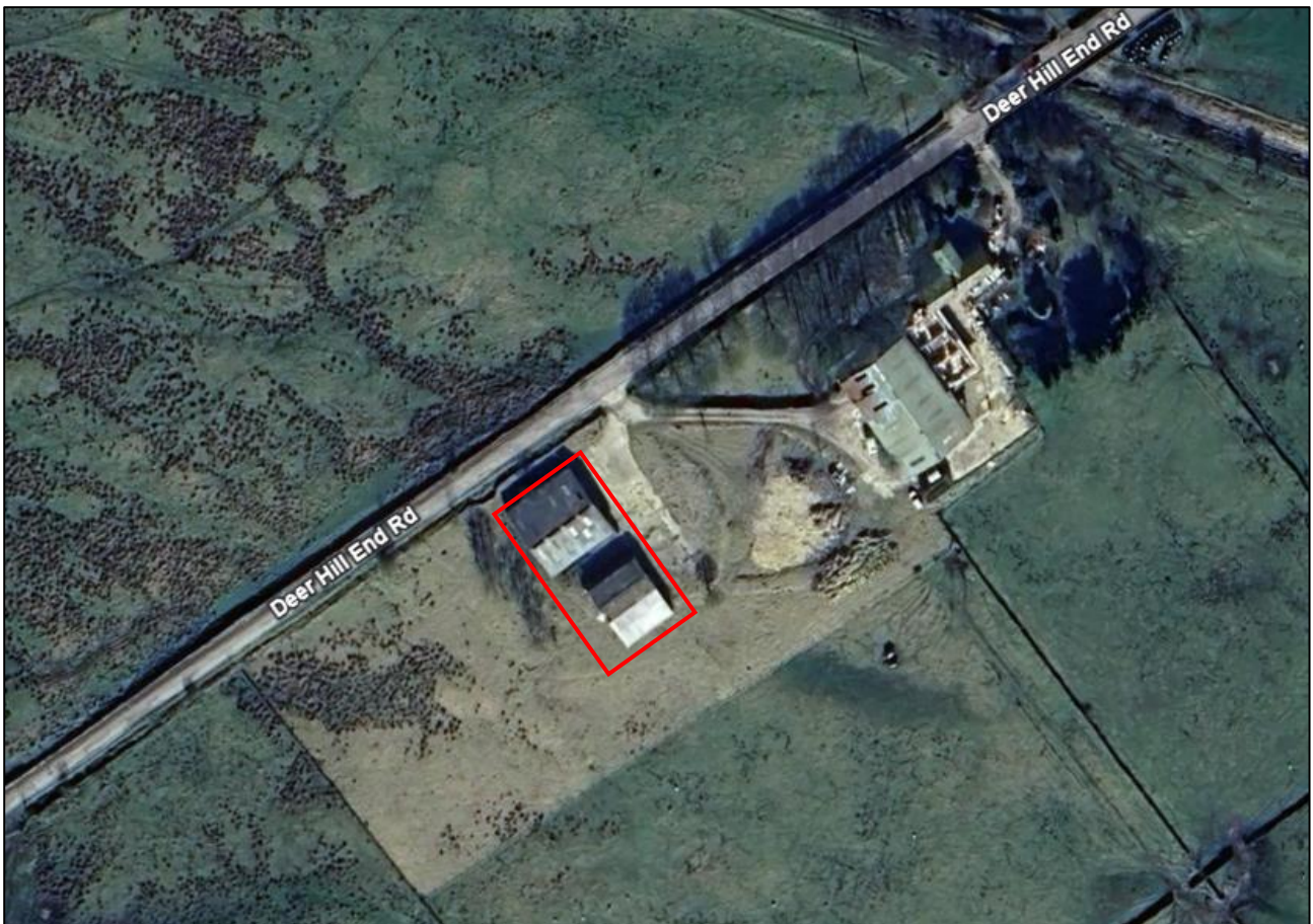
Figure 1.1 – Two agricultural buildings inspected as part of the survey.
