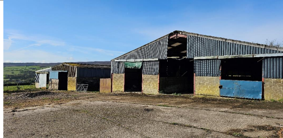
Photograph 1: Overview of the buildings northeastern aspect.
