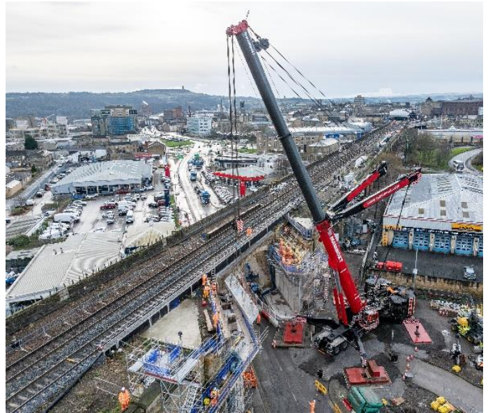
Figure 10: TransPennine Route Upgrade works in Huddersfield
