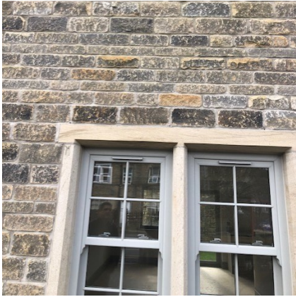
COURSED 'TUMBLED & DYED' NATURAL STONE WITH ASHLAR HEADS, CILLS AND MULLION
