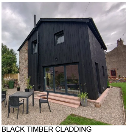
BLACK TIMBER CLADDING
