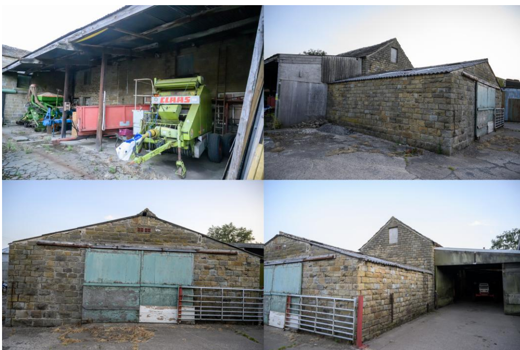
Photo 2. Main barn general views
