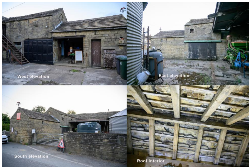
Photo 1: General view of the section of barn running south
