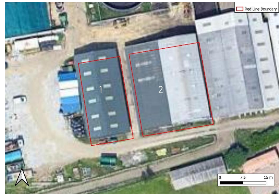
Figure 1 The surveyed building - red line.
