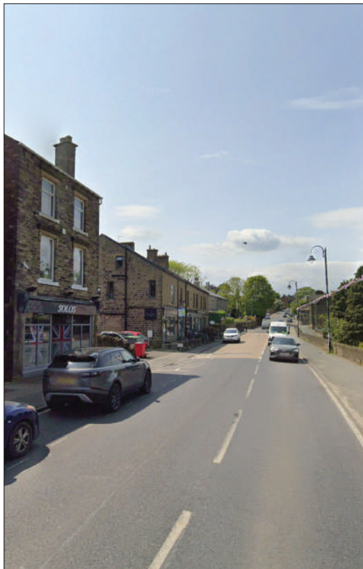
View towards access along Commercial Road
