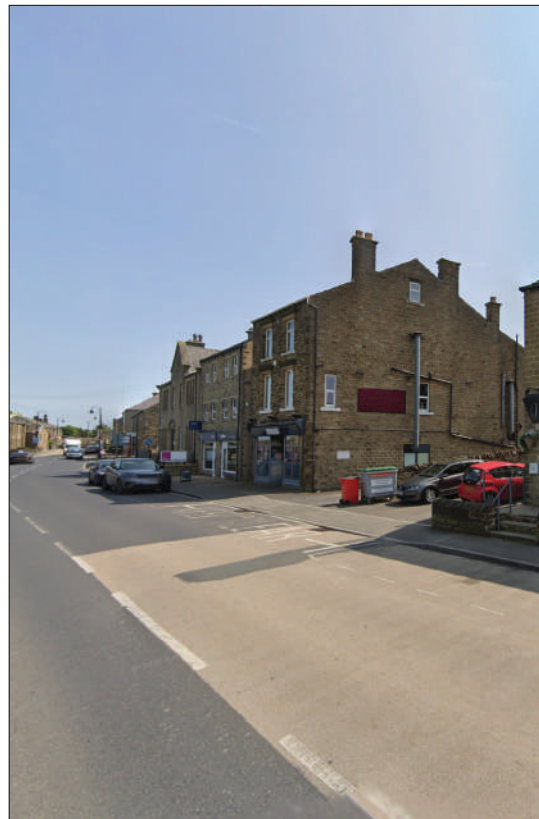
View towards access along Commercial Road
