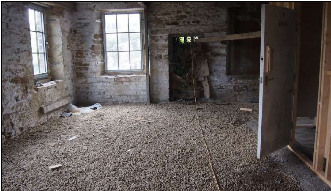
Plate 18: Interior view showing wall surface condition and internal floor space (Bankgate Mill (81).JPG, AHP).
