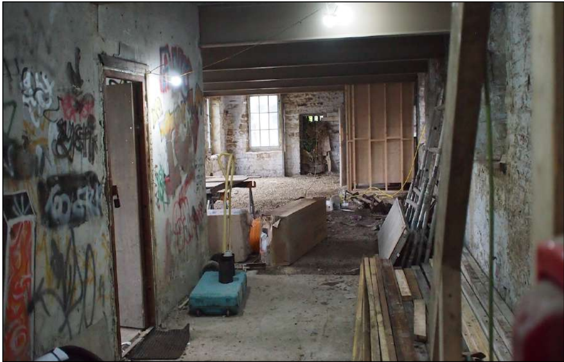
Plate 23: Interior view showing corridor or circulation space (Bankgate Mill (102).JPG, AHP).
