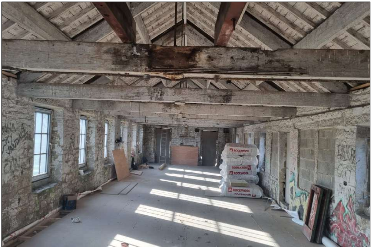
Plate 28: Third floor interior showing roof trusses and open floor space (17.jpeg, Client).
