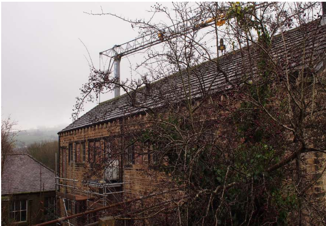
Plate 4: External view of the principal elevation showing multiple rows of window openings (Bankgate Mill (121)).JPG, AHP).
