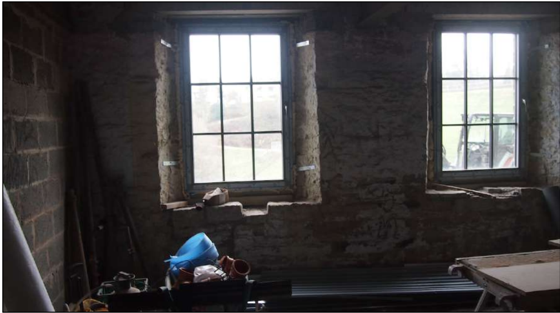
Plate 17: Interior view showing window bays along the external wall (Bankgate Mill (79).JPG, AHP).
