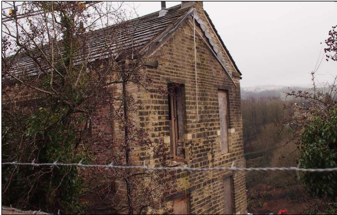
Plate 3: External view of the mill showing the gable elevation and surrounding context (Bankgate Mill (120)).JPG, AHP).
