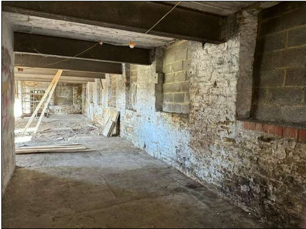
Plate 13: Ground floor interior showing masonry wall and structural beam (23.jpeg, Client).
