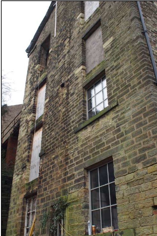
Plate 6: External close-up showing masonry wall construction and window openings (Bankgate Mill (123).JPG, AHP).
