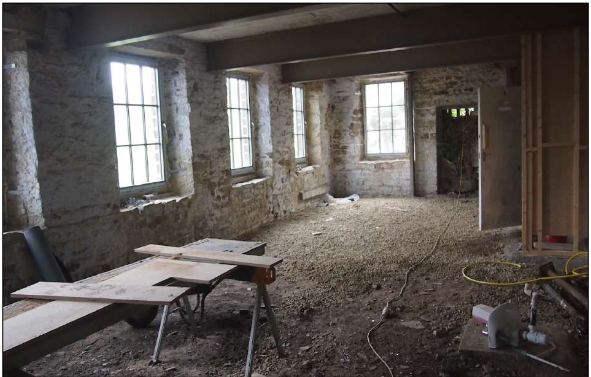
Plate 16: Interior view showing open floor space and window openings (Bankgate Mill (78).JPG, AHP).
