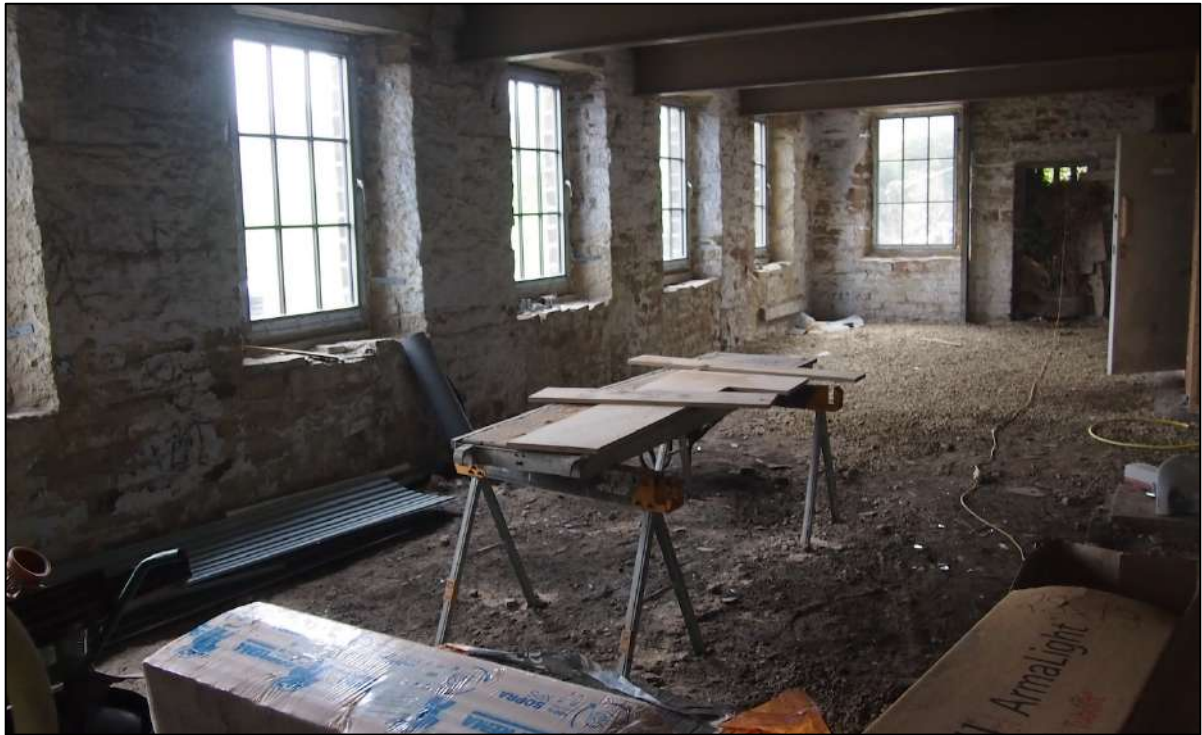
Plate 15: Interior view showing open room and structural walls (Bankgate Mill (76).JPG, AHP).
