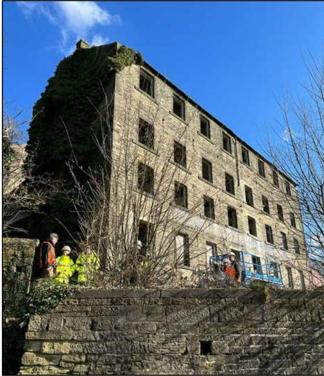
Plate 7: External view of the front elevation from below the retaining wall (25.jpeg, Client).
