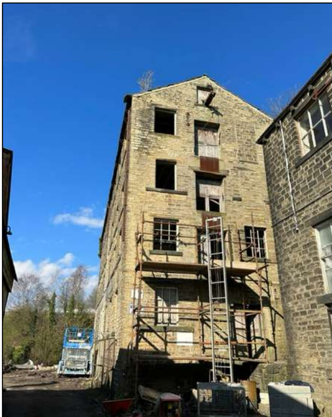
Plate 8: External view of the gable elevation showing scaffolding during works (31.jpeg, Client).
