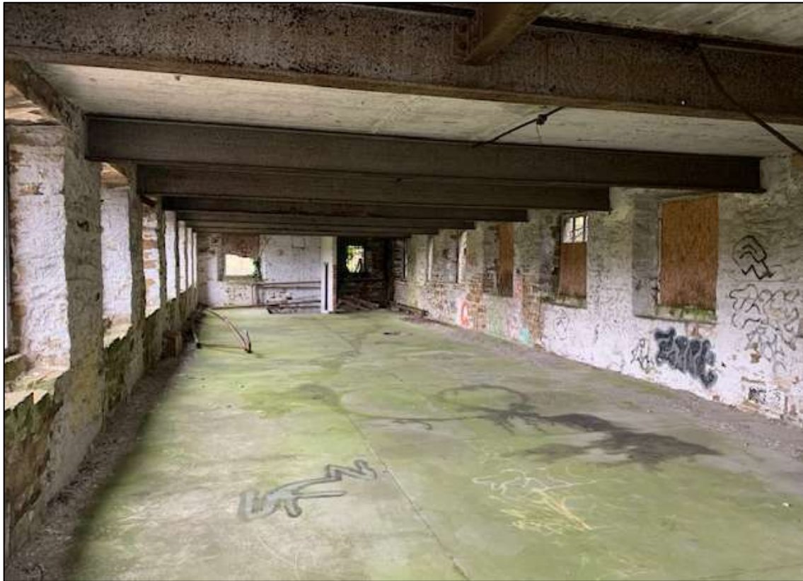
Plate 11: Ground floor interior long view across open floor space (4.jpeg, Client).
