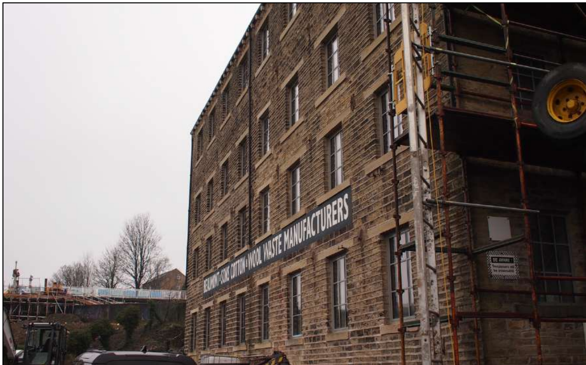
Plate 2: External oblique view of the mill building (Bankgate Mill (101).JPG, AHP).
