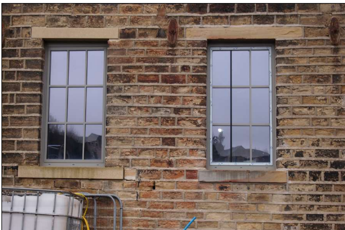
Plate 10: External detail of stone masonry wall and modern window openings (Bankgate Mill (90).JPG, AHP).
