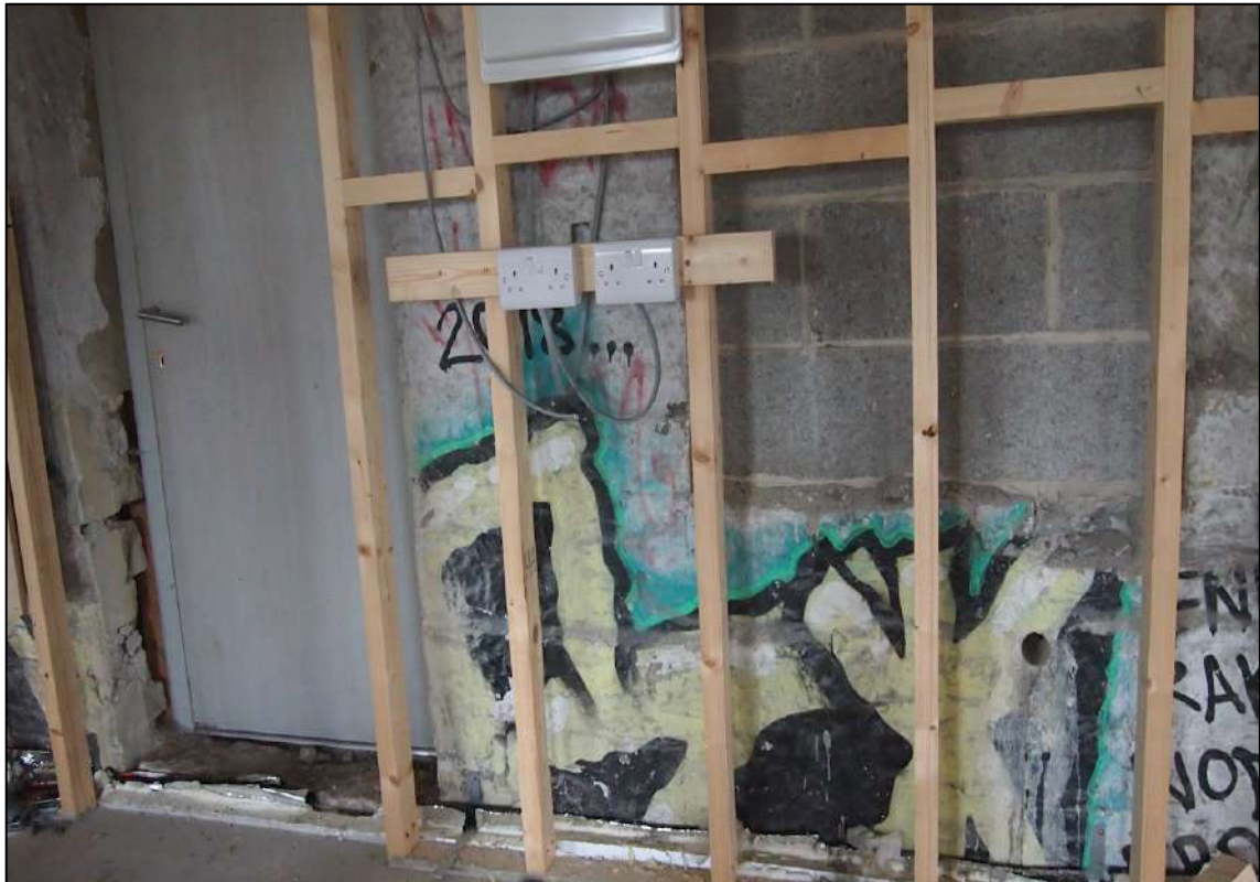
Plate 25: Interior detail showing graffiti behind the modern partitions (Bankgate Mill (10).JPG, AHP).
