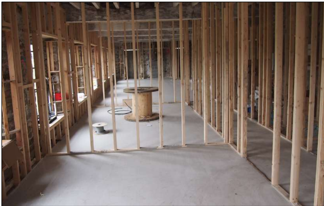
Plate 14: Interior view along open floor space with partition framing (Bankgate Mill (41).JPG, AHP).
