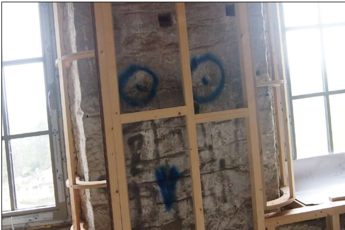
Plate 26: Interior detail showing modern framed opening within an external wall (Bankgate Mill (11).JPG, AHP).
