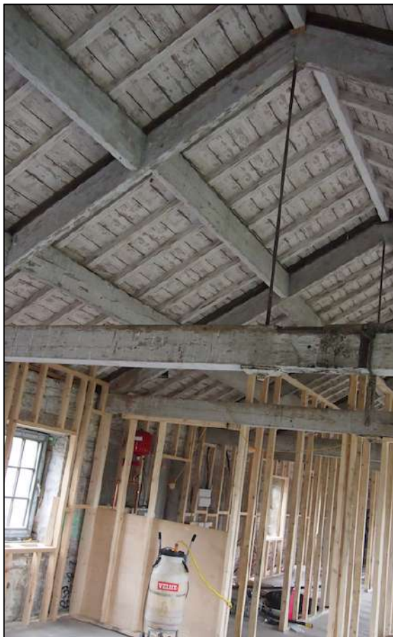
Plate 24: Interior view showing roof trusses and timber structural members (Bankgate Mill (6).JPG, AHP).
