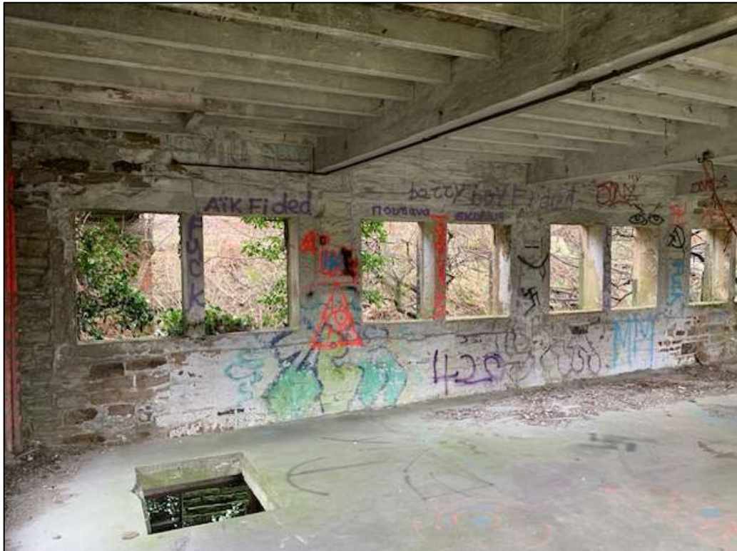
Plate 19: Interior view showing graffiti, access point and wall surfaces (10.jpeg, Client).
