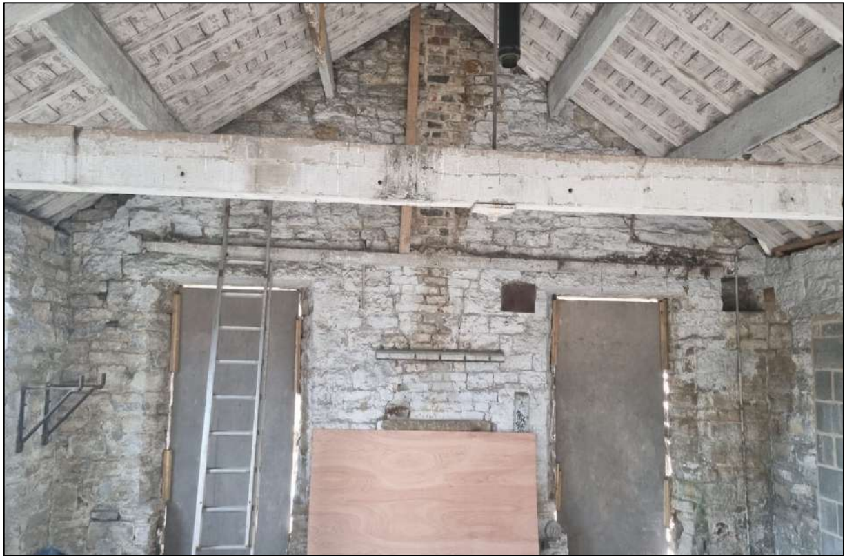
Plate 29: Third floor interior showing roof structure and gable wall (21.jpeg, Client).
