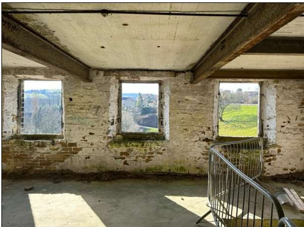
Plate 20: Interior view showing window openings (24.jpeg, Client).
