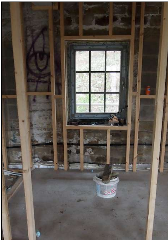
Plate 22: Interior detail showing modern framed opening within an internal partition (Bankgate Mill (42).JPG, AHP).
