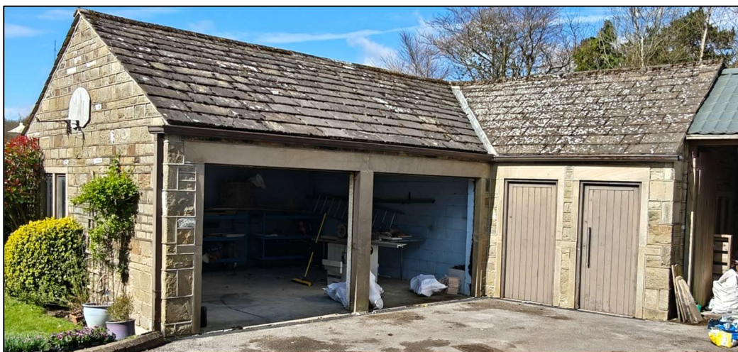
View of existing garage / store – pointing in excellent conditions and no gaps for bats to enter.
