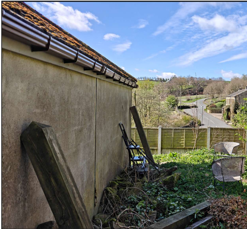
View of existing garage / store rear – again, no gaps for bats to enter.
