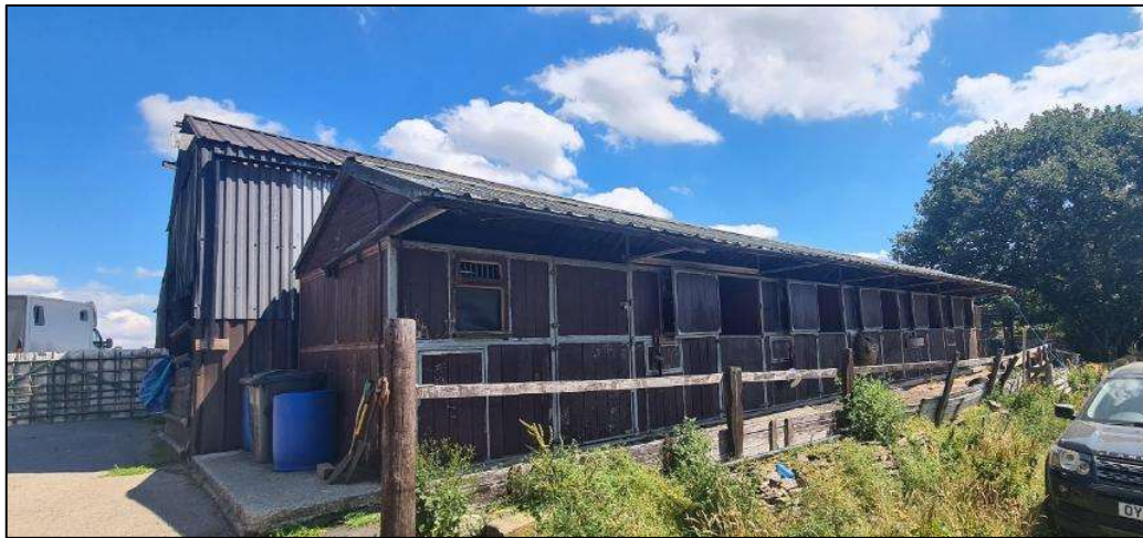
Plate 15. Building B viewed from the southwest
