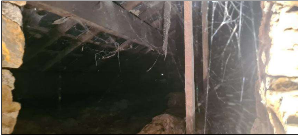
Plate 14. The interior of the roof showing the large timber purlin and rafters as well as heavy cobwebs
