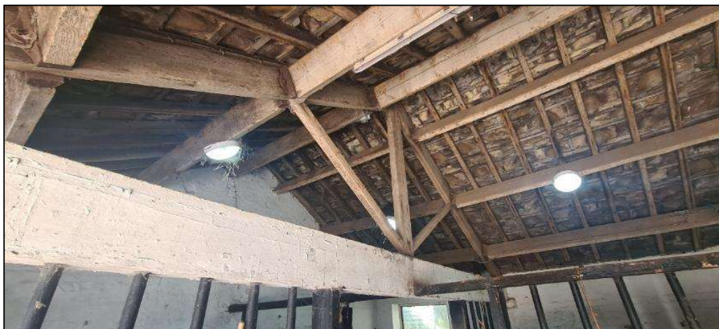
Plate 19. The underside of the roof at the northern end of the building.
