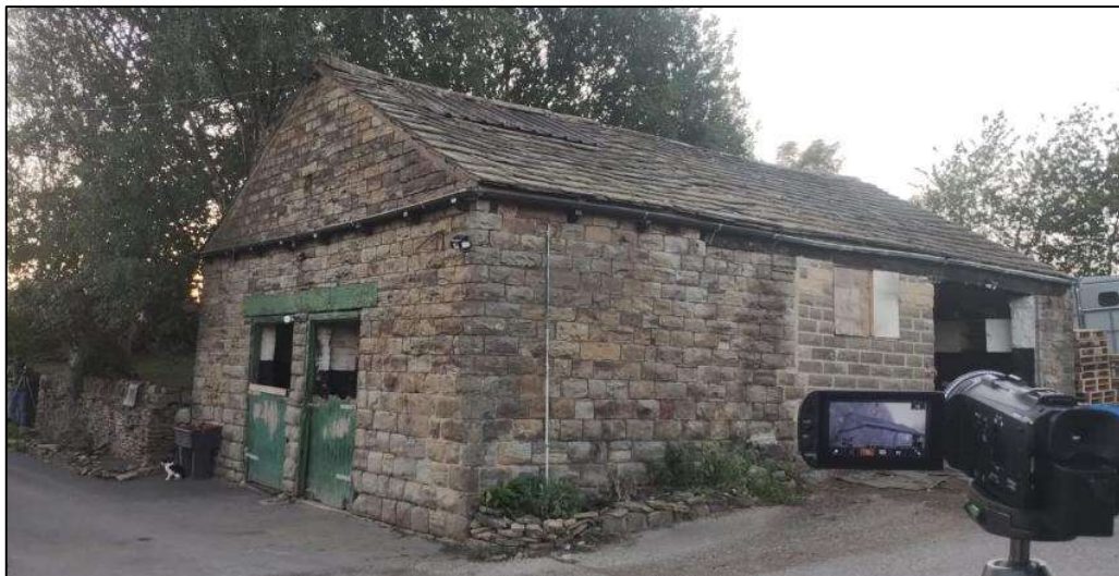
Plate 18. Building C viewed from the southeast
