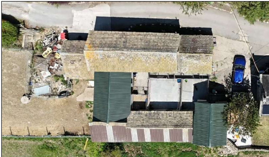
Plate 23. The roof of Building D
