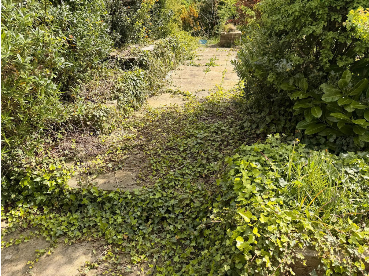
Plate 8: Narrow Access Constraints – View of restrictive pathways between the dwelling and garden walls that fail to accommodate 1500mm turning circles.
