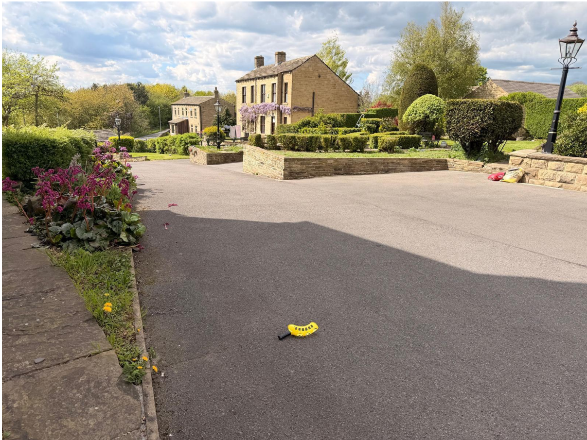
Plate 2: Primary Site Gradient – Illustrating the steep, descending driveway which presents a severe fall risk for Blue Badge holders with restricted mobility.
