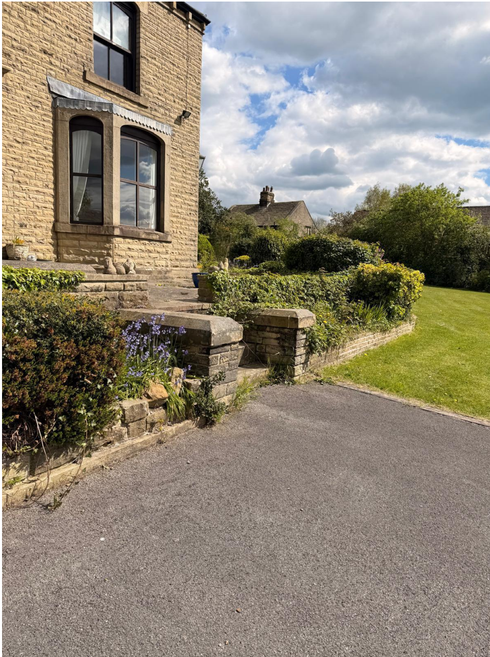
Plate 3: Vertical Access Barrier – Close-up of multi-level stone steps leading to the terrace, demonstrating the "accessibility gap" between the dwelling and the garden.
