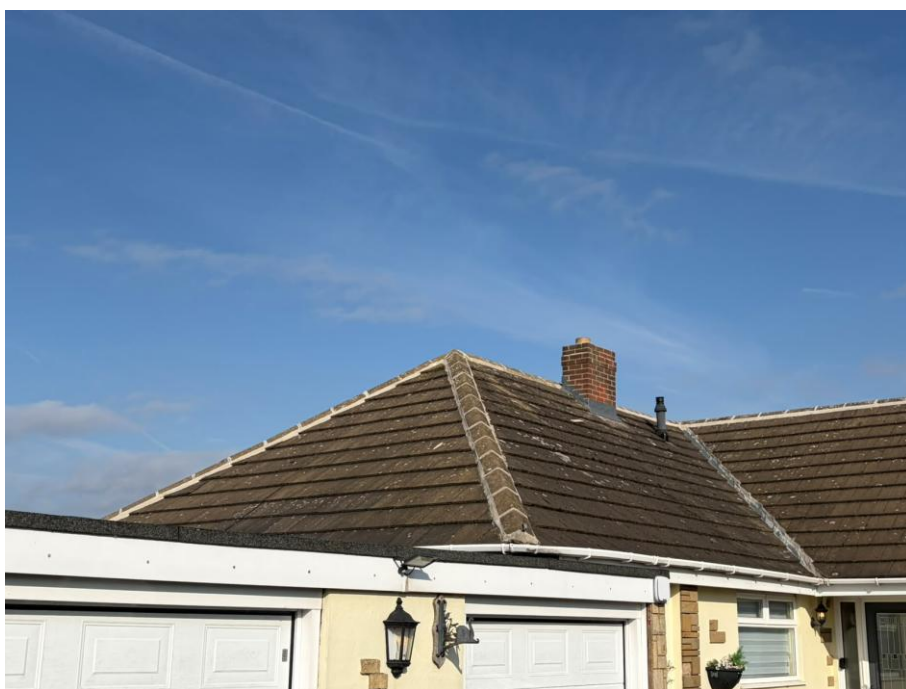
Figure 8 The southeastern aspect of the roof of B1
