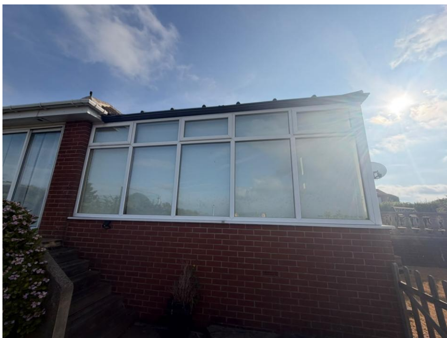
Figure 9 The western aspect of B1
