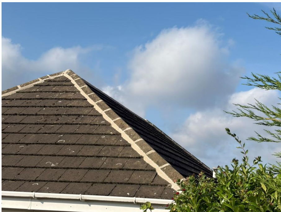
Figure 5 The roof of B1, viewed from Woodlands Road, looking west
