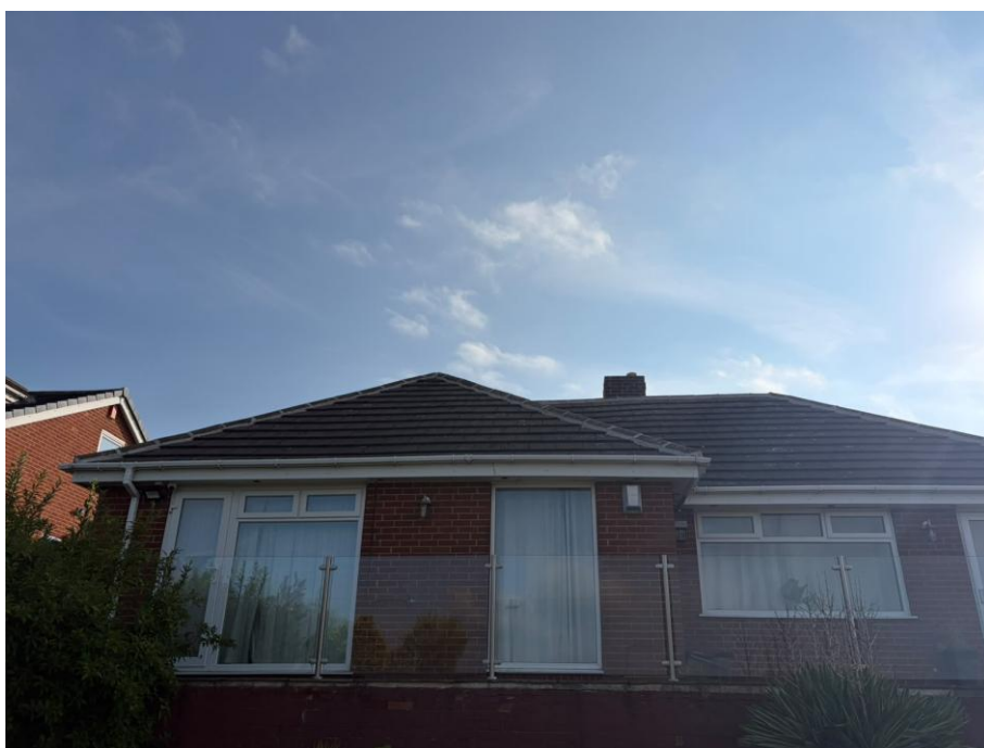
Figure 10 The western aspect of B1
