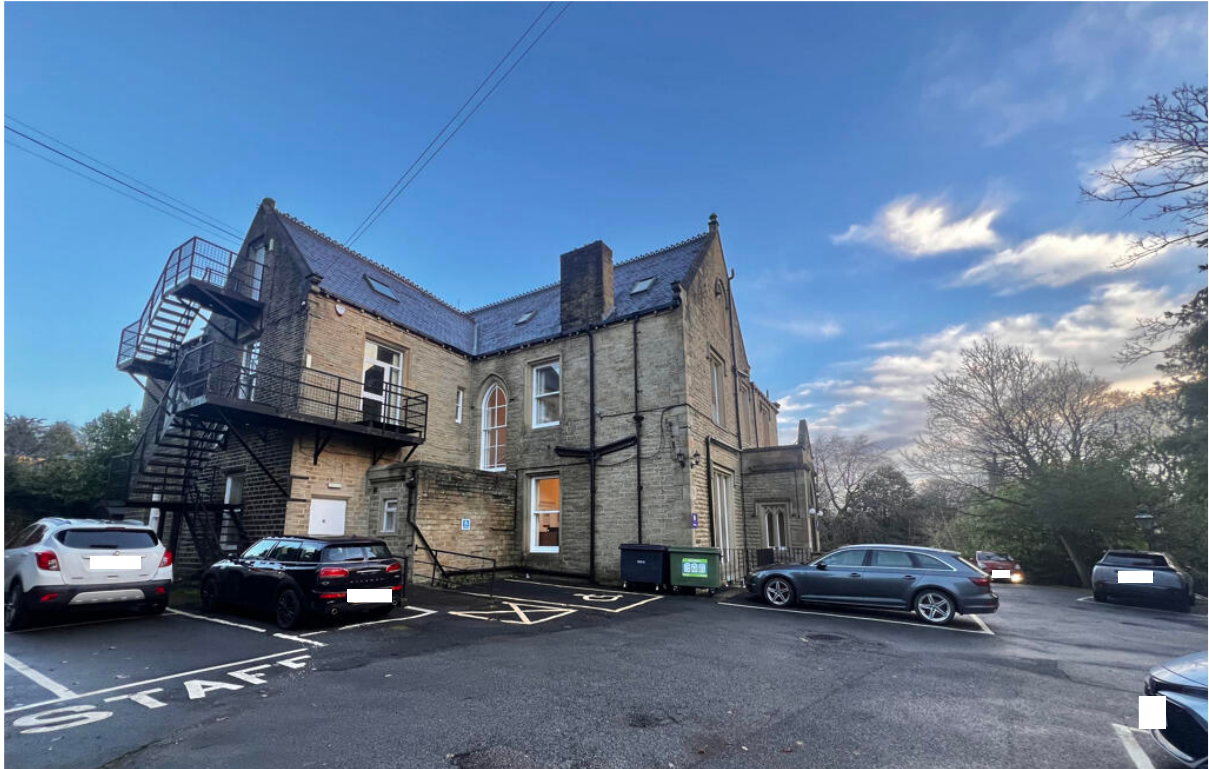
Photo 3. Side and rear elevations
