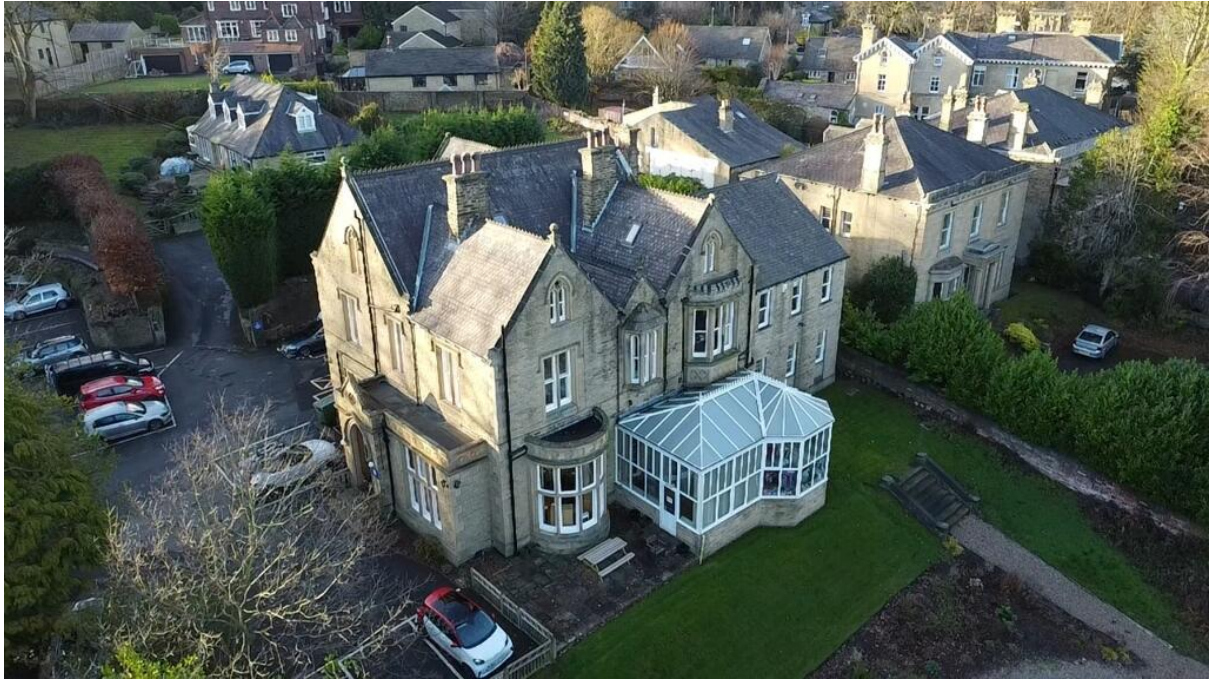
Photo 1. Aerial of garden facing elevation showing conservatory proposed for removal
