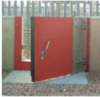
Figure 3. Concrete walls and flood gates
