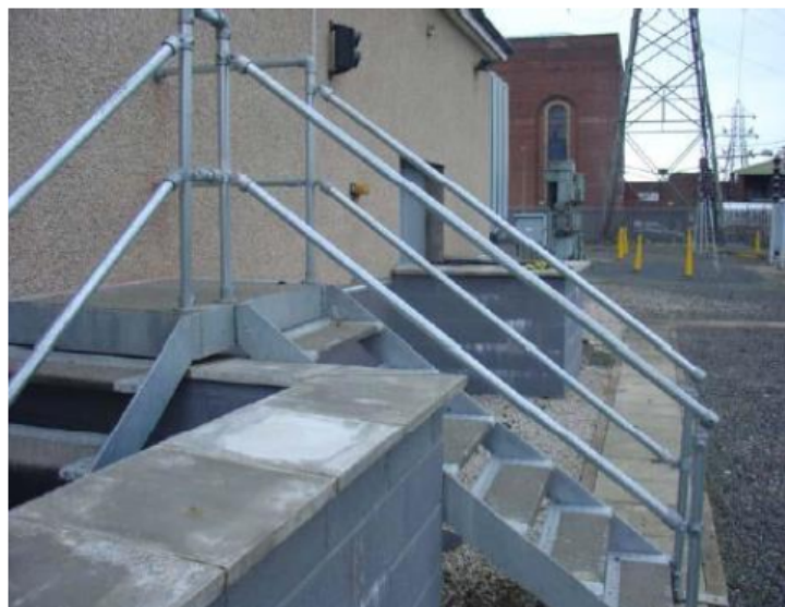
Figure 5. Access to Substation entrance (ENA ETR138 Annex 1)
