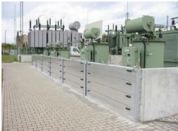
Figure 4. removable flood panels (ENA ETR138 Annex 1)
