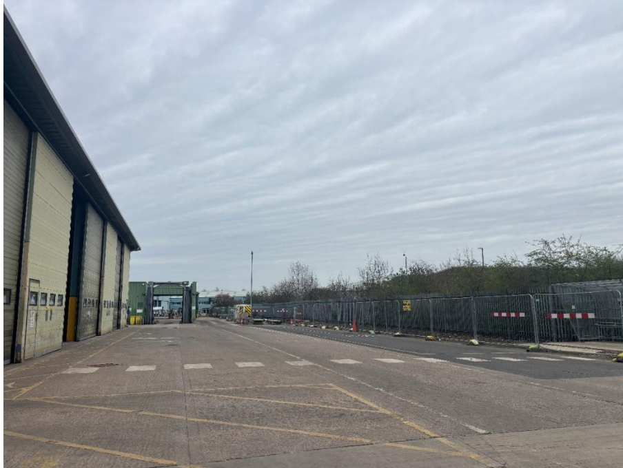
Figure 5. View of the hardstanding access and car parking area on site (March 2026).
