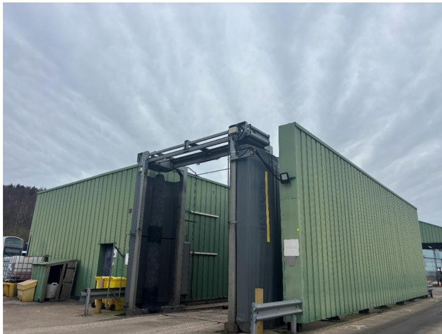
Figure 9. Bus wash station with negligible bat potential (March 2026).
