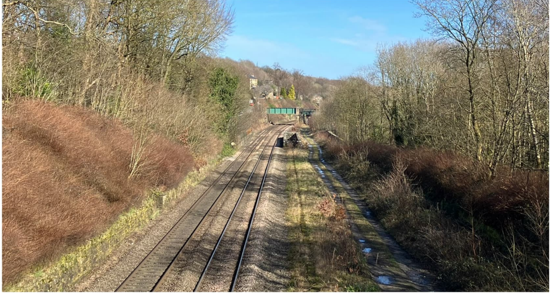
Figure 11: Golcar viaducts' decks and parapets from Lockwood footbridge, with Britannia Road bridge at rear, looking north east. Tracks pass over MVL3/69.
