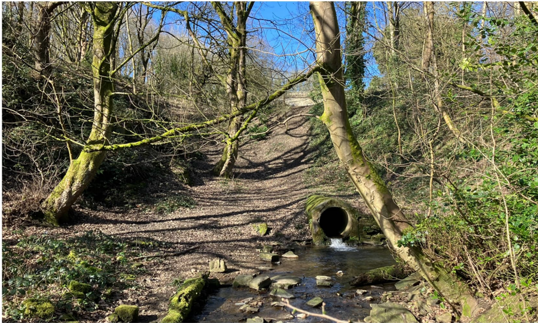
Figure 9: The top of the viaduct parapet from the riverside path.
