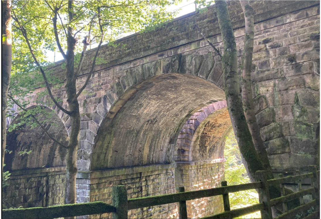
Figure 15: North elevation of Golcar new viaduct MVL3/69 central arches from footpath.
