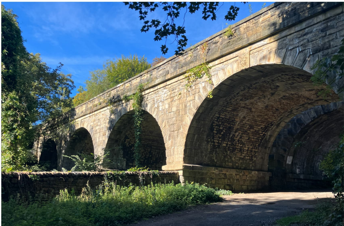
Figure 14: South elevation of the original viaduct MVL3/70 from farm track.
