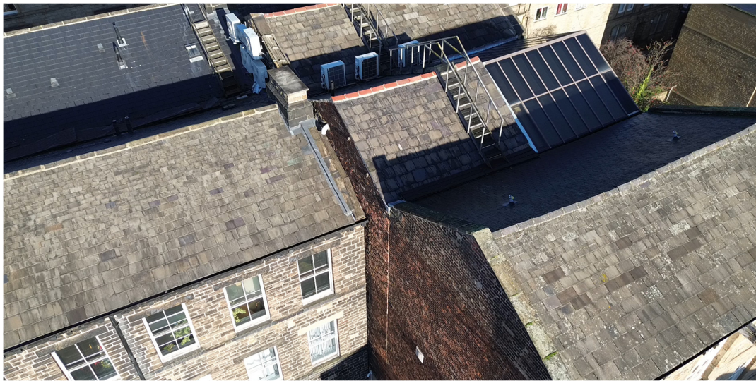
Figure 7 – The existing roofs of 23/21 Bond street. Note the modern glazing.
