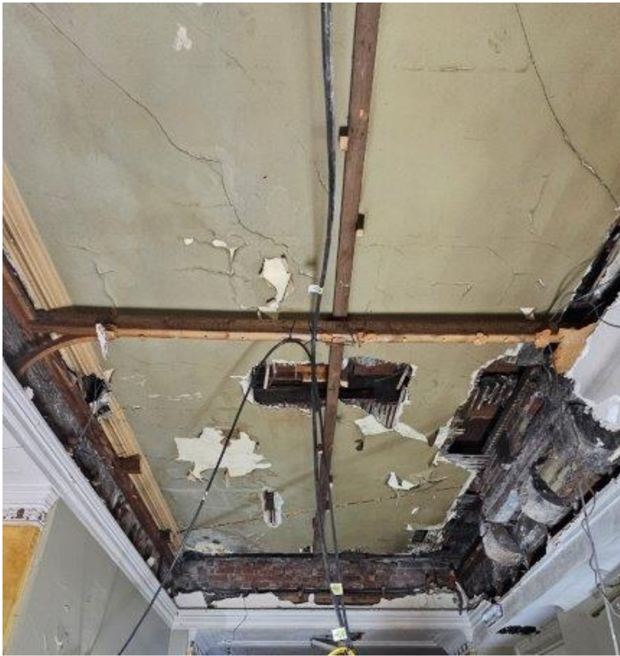
26.04.16 - 20260416_100920 – Ground Floor Context (Room 047) – Concealed ceiling exposed
