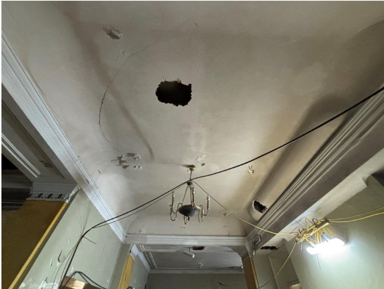
IMG_4416 – 1 st floor (U/S) as viewed from Ground floor (Room 047).
