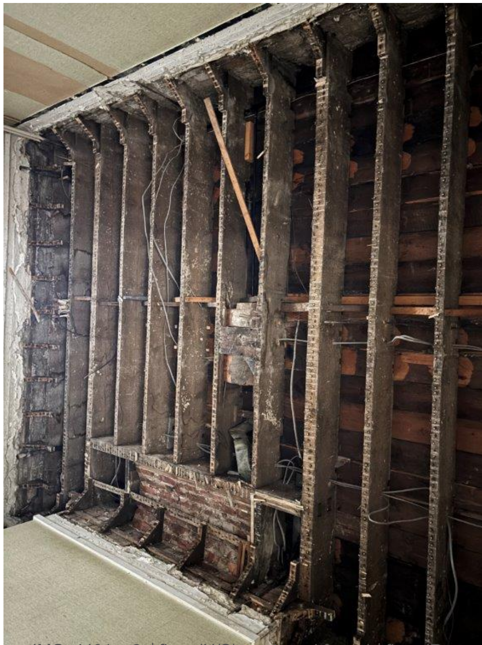
IMG_4401 – 2 nd floor (U/S) as viewed from 1 st floor (Room 095).
