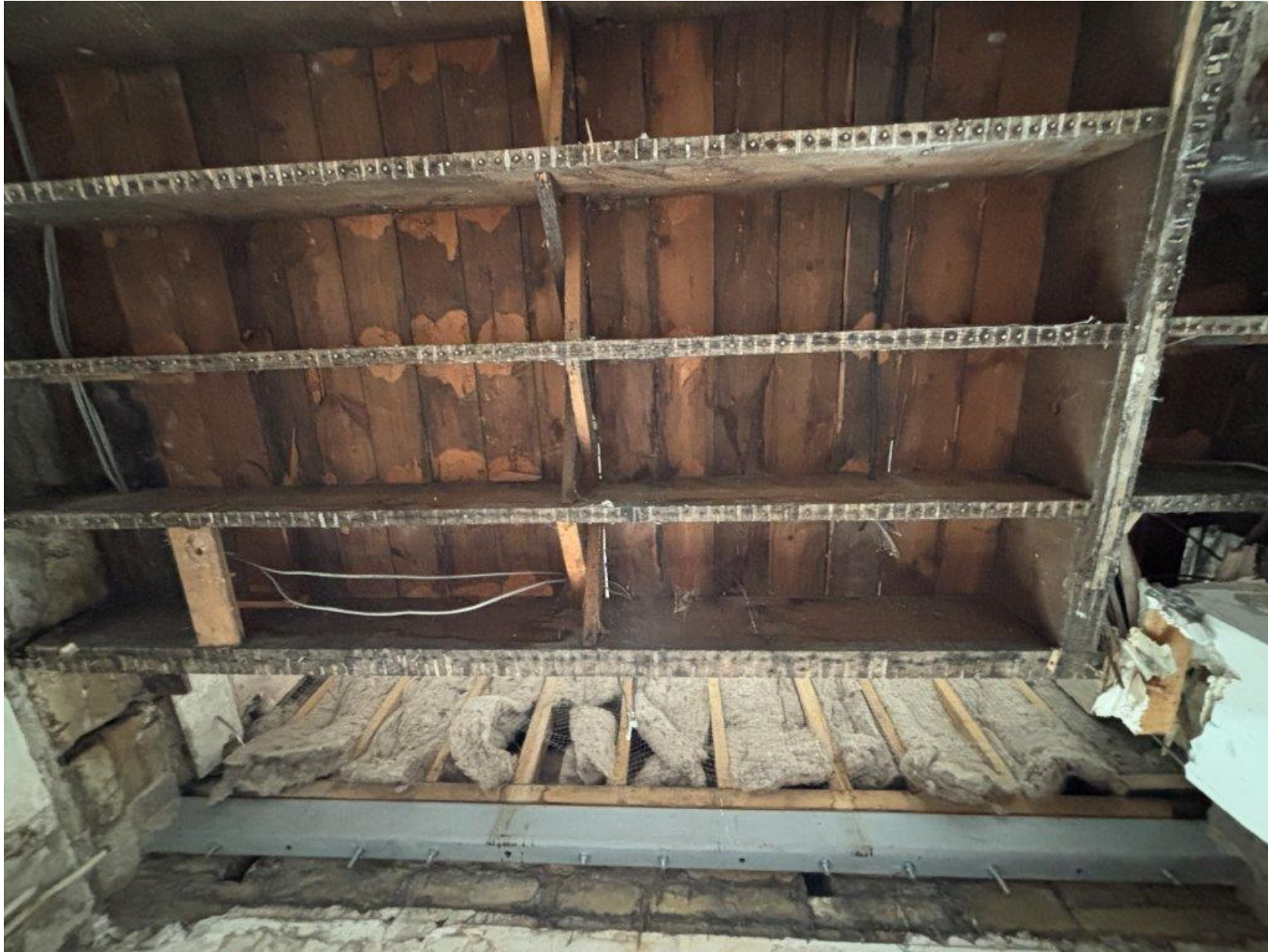
IMG_4393 - 4 th floor (U/S) as viewed from 3 rd floor (Room 181)
