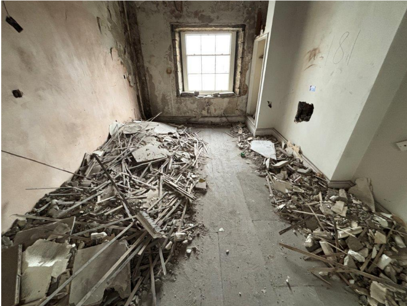
IMG_4395 – 3 rd floor context (Room 181)
