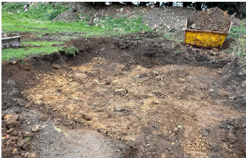
Excavation area showing evidence of made ground
