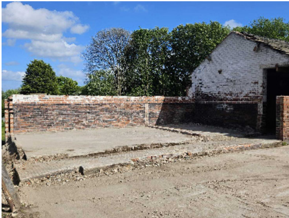
18/5/2026 - View of demolished outbuilding facing west
