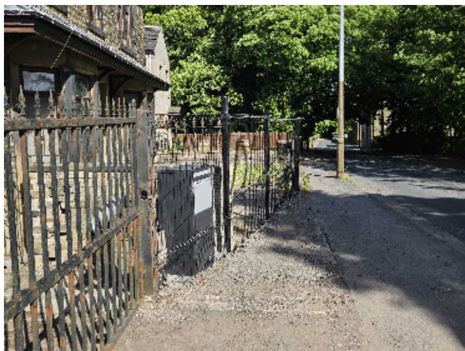
18/5/2026 - Demolished walling and realigned railings to new VS looking west along Whitechapel Road
