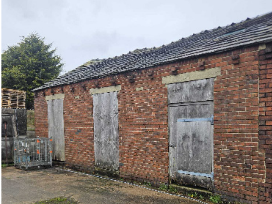
18/5/2026 - View of the end terraced outbuilding facing west pre-demolition
