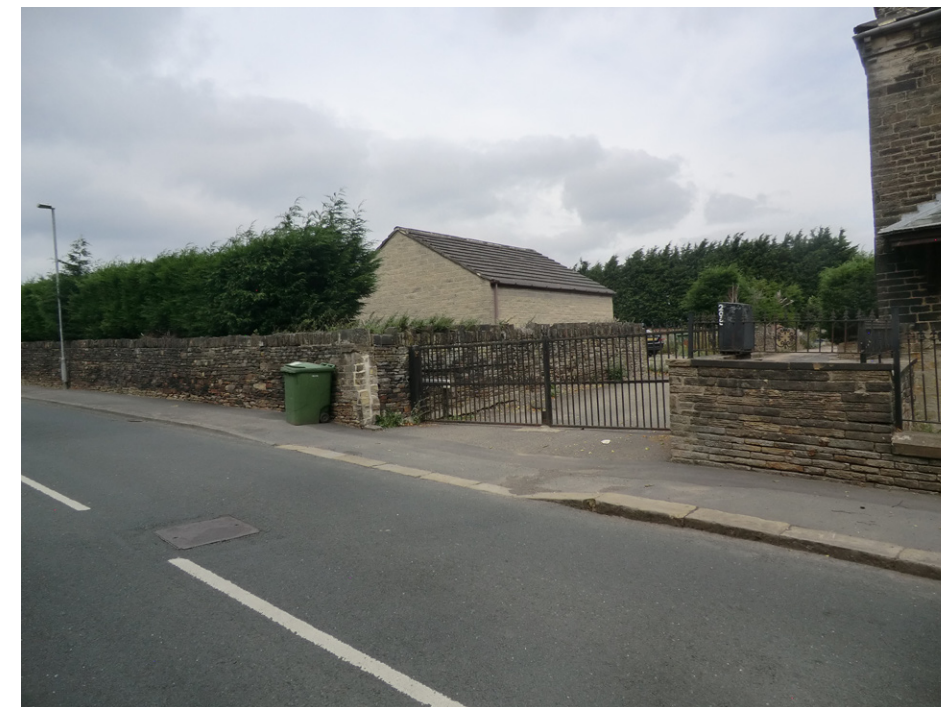
22/8/2018 - View of the existing access looking west along Whitechapel Road
