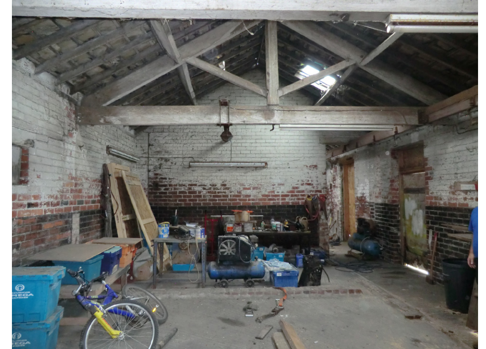
22/8/2018 - Internal image of the outbuilding pre-demolition
