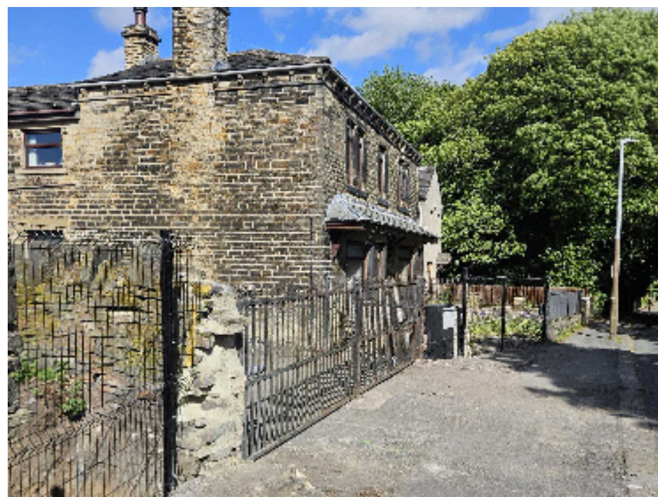
18/5/2026 - Section of stone walling demolished and realigned railings to new VS looking east along Whitechapel Road.
