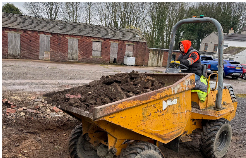
Contaminated material being removed to skip on site
