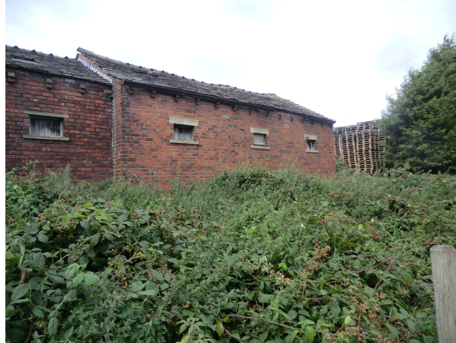
22/8/2018 - View of the end terraced outbuilding facing east pre-demolition
