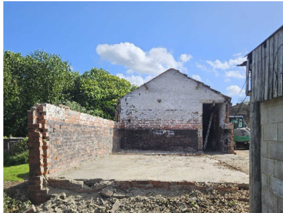
18/5/2026 - View of demolished outbuilding facing north
