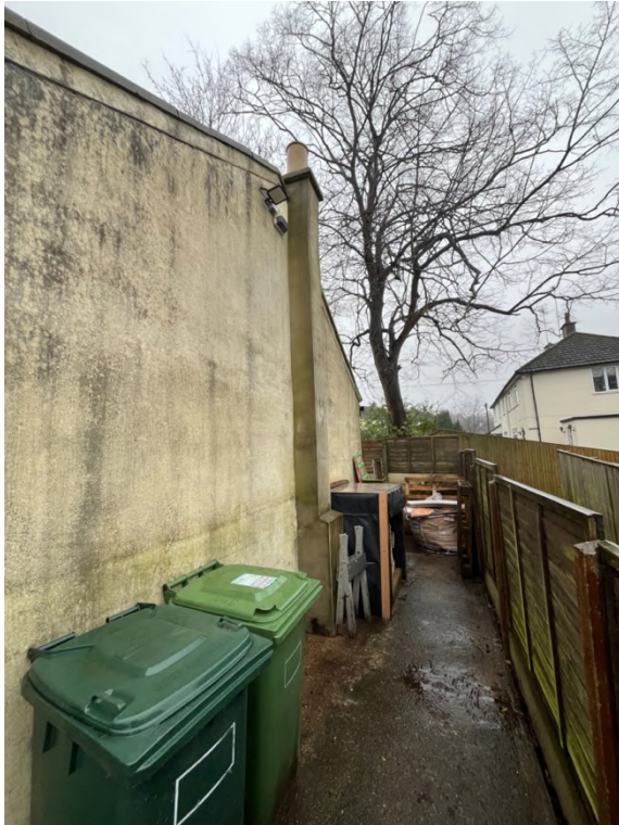
Figure 11: Existing bin store, visible from Fleminghouse Lane
