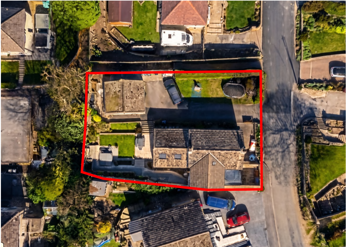
Figure 3: Aerial view of site as existing
