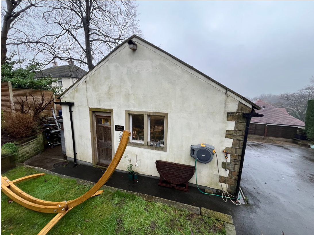
Figure 9: Existing pedestrian entrance to garage
