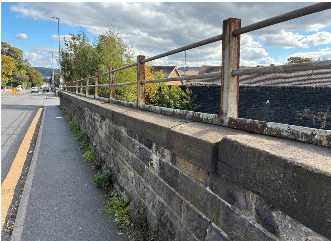
Figure 11: Deck looking south, west parapet and handrail with bottom rail.
