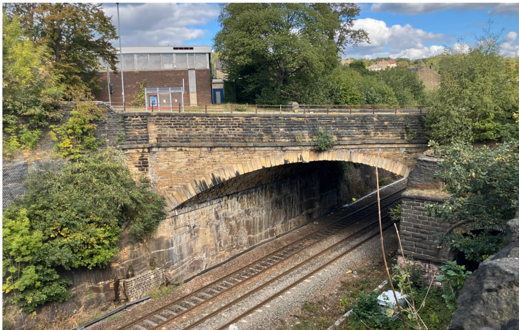
Figure 9: West elevation of Paddock Bridge with later tunnel to right
