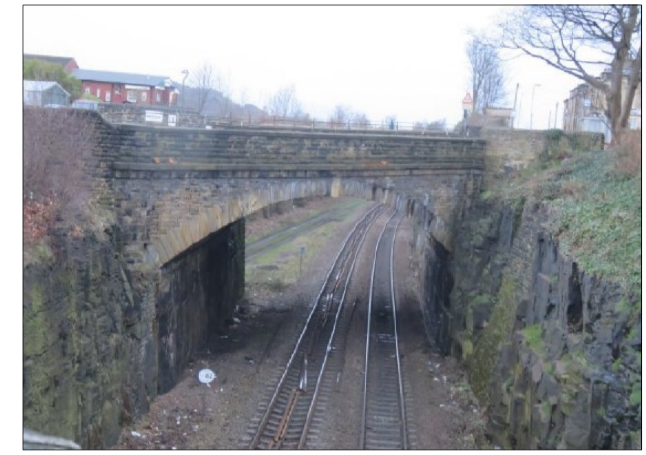
Photo 1 (Looking South West) Scale N.T.S
