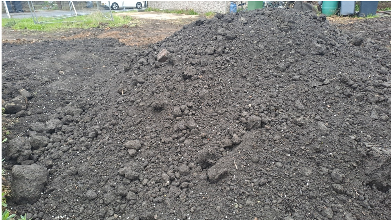
28.04.26 Stockpile of topsoil brought on to site (front of image). Placed already in the background.
