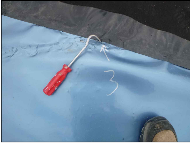
A Minor gap in perimeter joint, 25/04/2025
