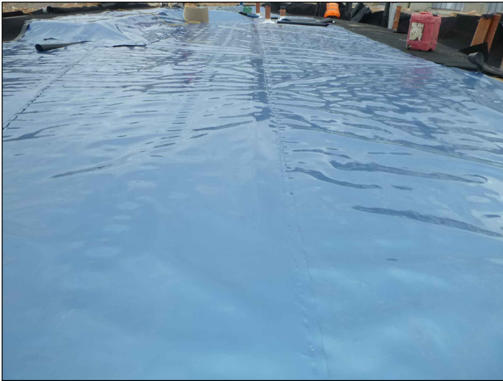
A | Extrusion welded membrane joins, 25/04/2025
