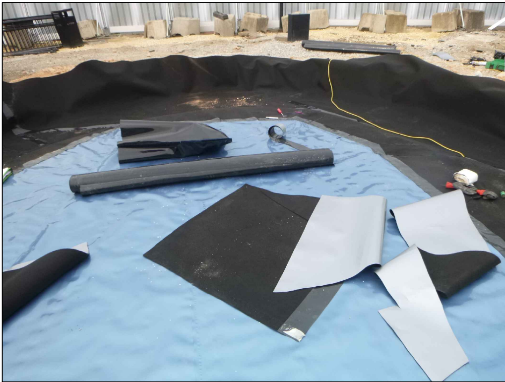
A Completed Titanbond perimeter installation, 28/04/2025
