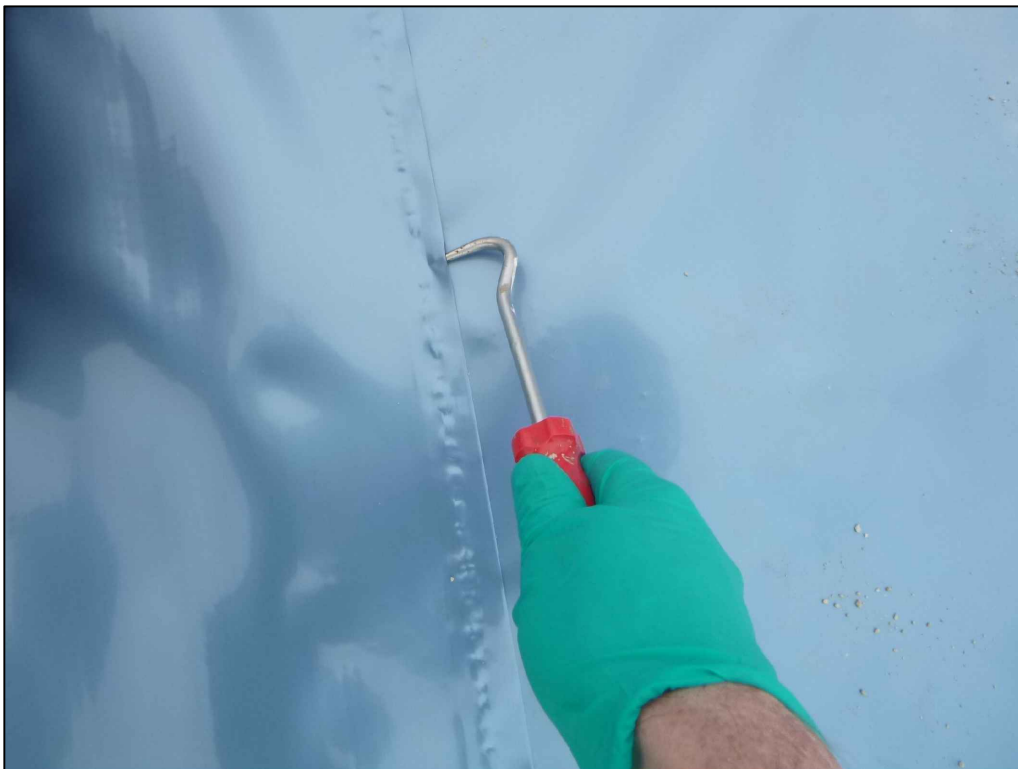
B | Testing an extrusion welded joint, 25/04/2025
