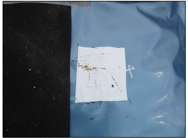
D Patch used to repair defect shown in C, 25/04/025
