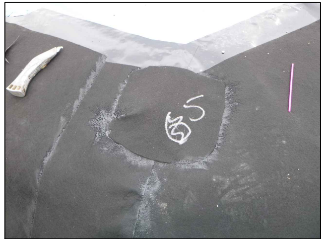
F Patch used to repair defect shown in E, 28/04/025
