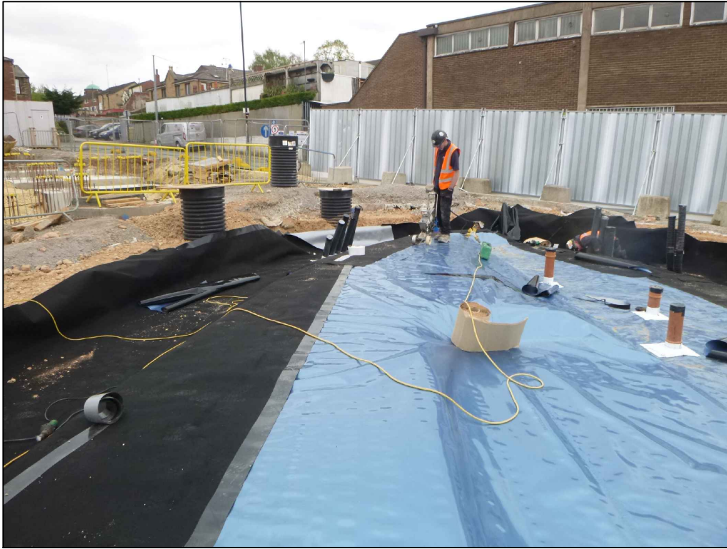
A General view of site during installation, 25/04/2025
