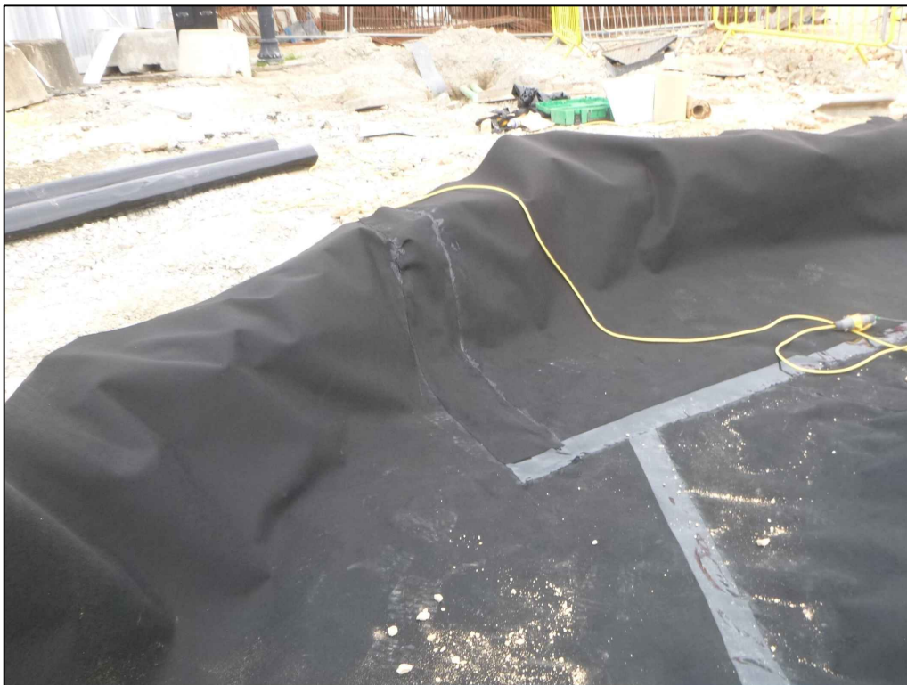
B Perimeter join covered with Titanbond strip, 28/04/2025
