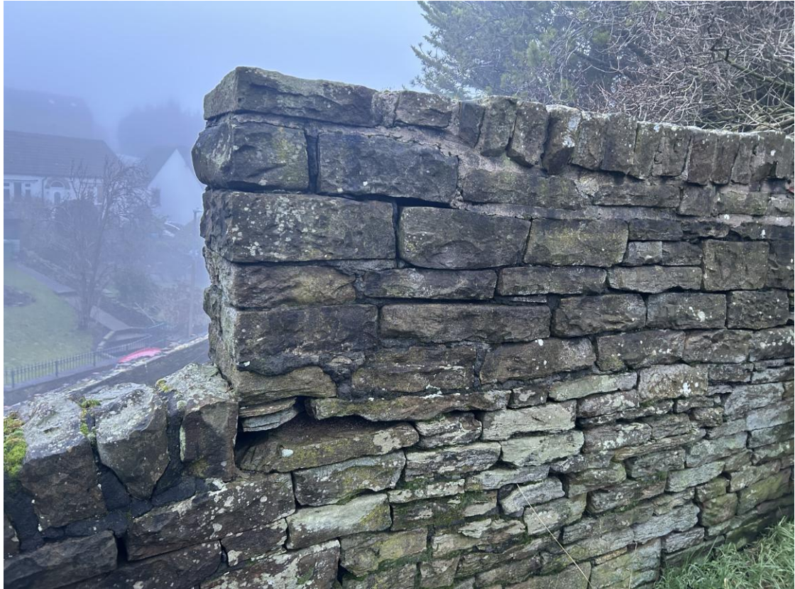
Photo B/R/25T – Wall B, Rear Face, ~CH 24.5m (Upper Parapet – Top Section)
