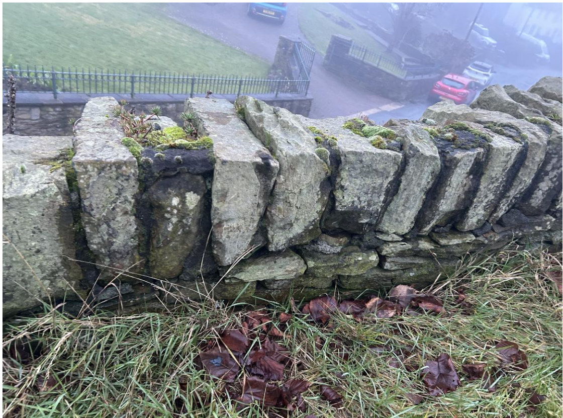
Photo B/R/6 – Wall B, Rear Face, ~CH 11.8m (Upper Parapet)
