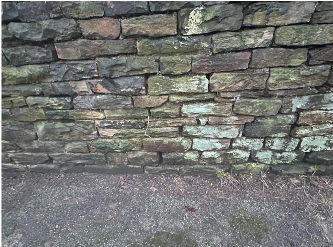
Photo E/F/3B – Wall A, Front Face, ~CH 1.0m (Lower Section)
