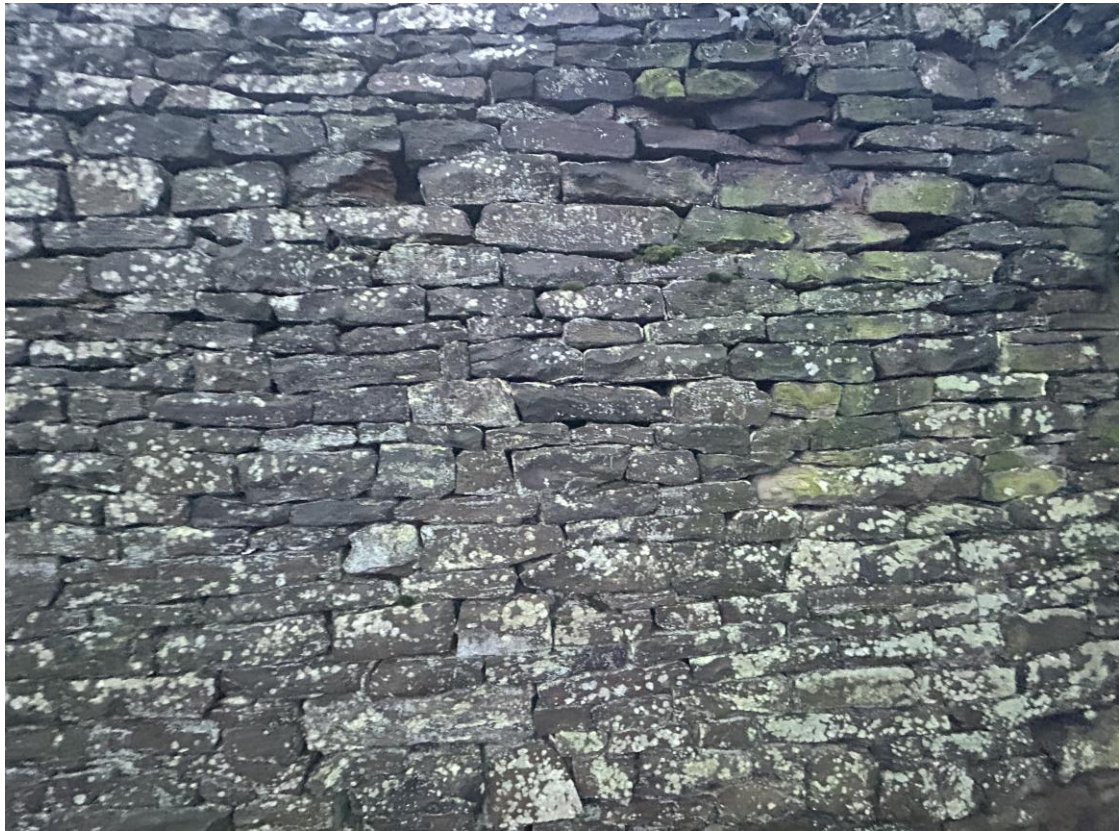
Photo B/F/4M – Wall B, Front Face, ~CH 8.5m (Middle Section)
