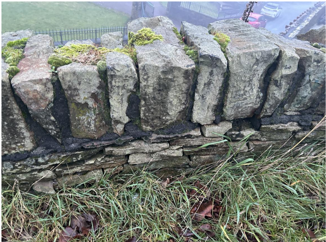
Photo B/R/10 – Wall B, Rear Face, ~CH 14.5m (Upper Parapet)
