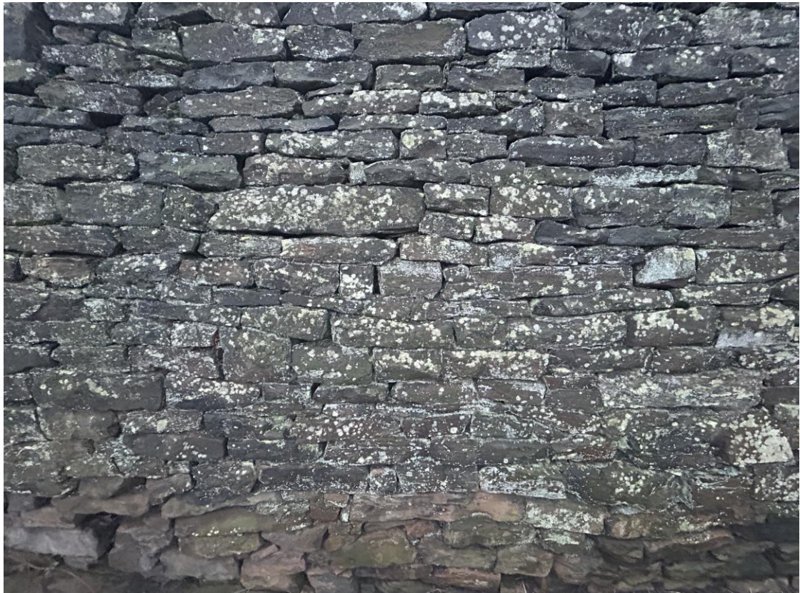
Photo B/F/5L – Wall B, Front Face, ~CH 10.2m (Lower Section)
