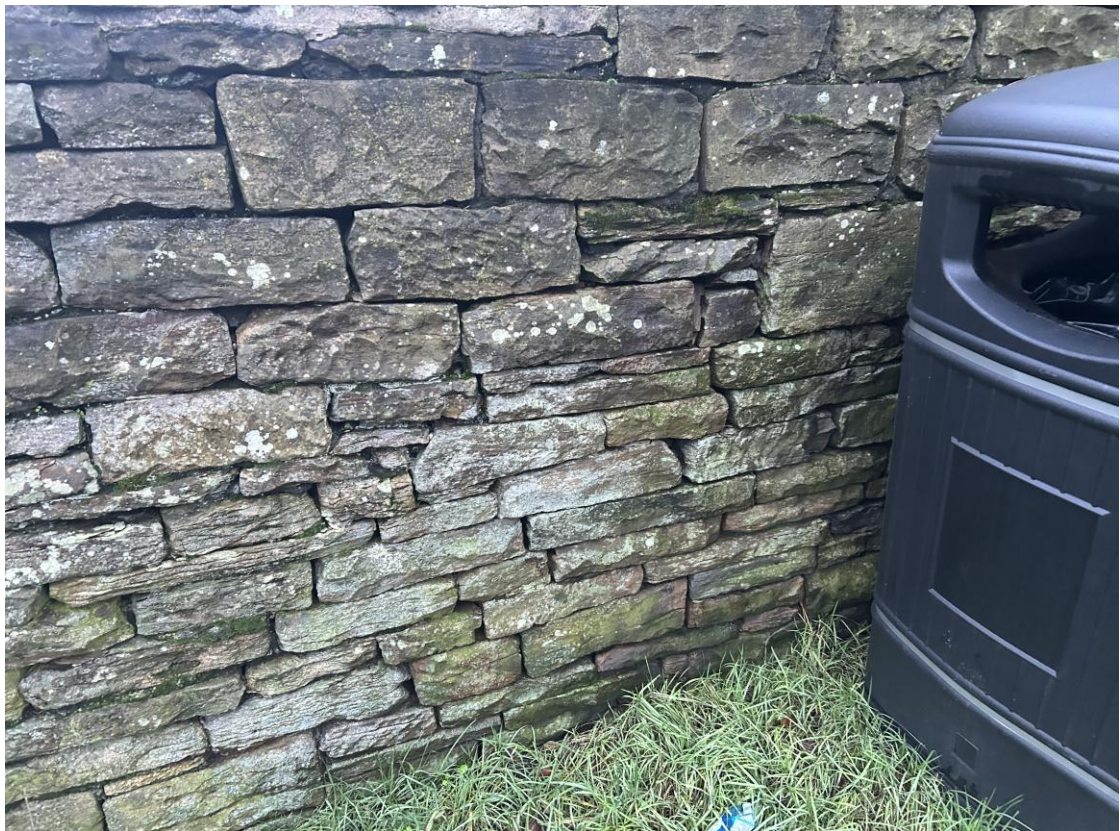
Photo B/R/26B – Wall B, Rear Face, ~CH 25.8m (Upper Parapet – Lower Section)
