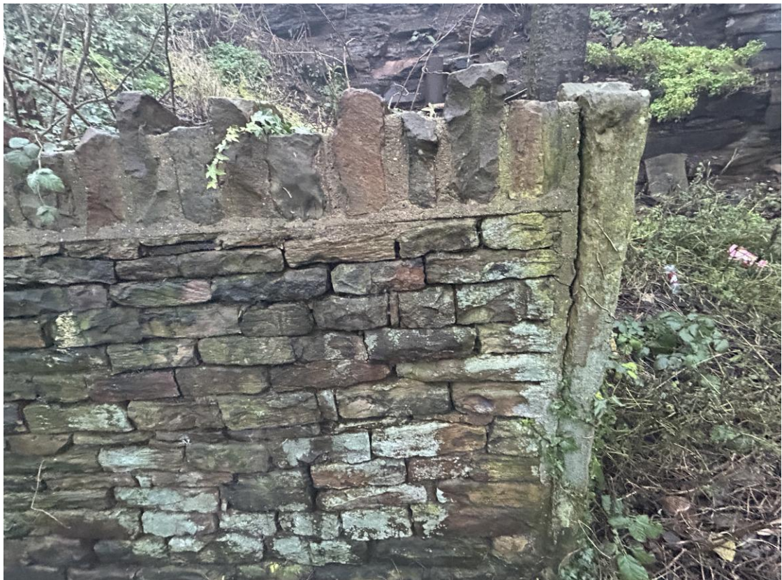
Photo B/F/2T – Wall A, Front Face, CH 0.0m (Upper Section)
