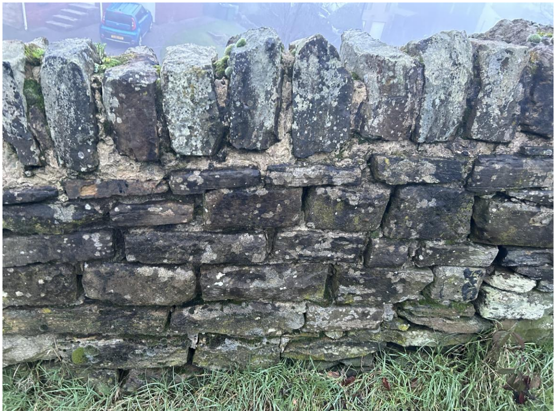
Photo B/R/22 – Wall B, Rear Face, ~CH 22.5m (Upper Parapet)
