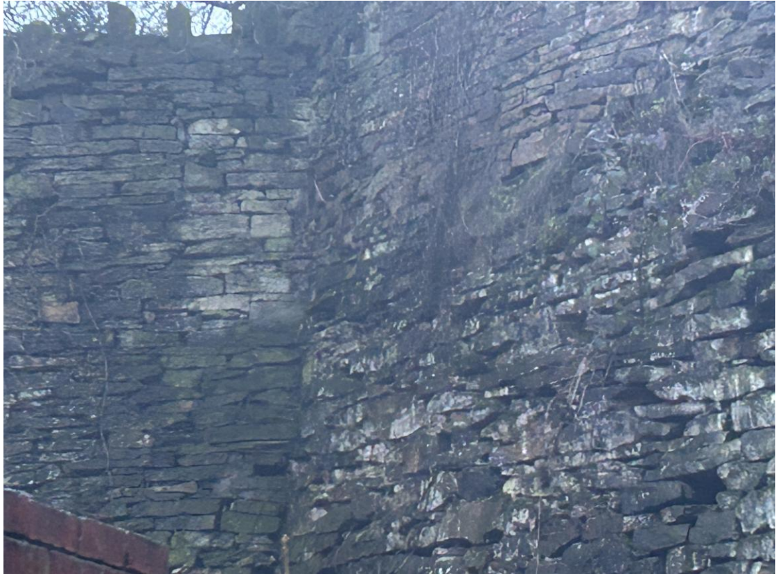
Photo B/F/14M – Wall B, Front Face, ~CH 27.0m (Middle Section)
