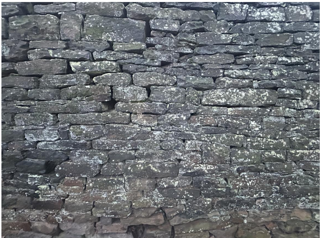
Photo B/F/6B – Wall B, Front Face, ~CH 11.5m (Lower Section)
