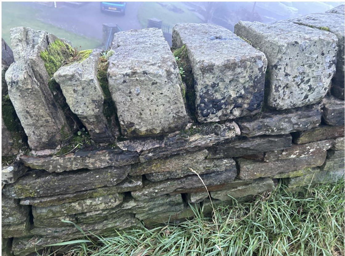
Photo B/R/16 – Wall B, Rear Face, ~CH 18.5m (Upper Parapet)
