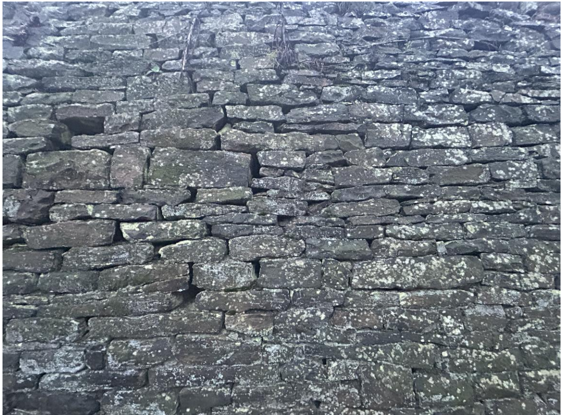
Photo B/F/6M – Wall B, Front Face, ~CH 11.5m (Middle Section)
