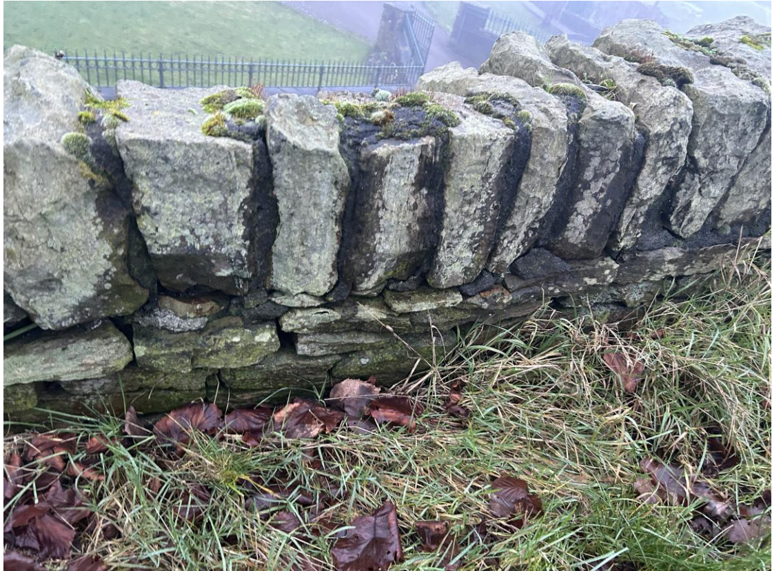
Photo B/R/7 – Wall B, Rear Face, ~CH 12.5m (Upper Parapet)
