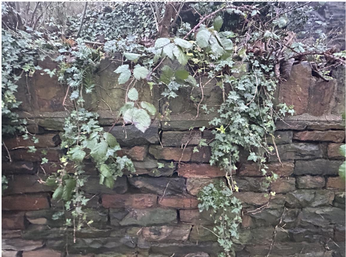
Photo J/F/6T – Wall A, Front Face, ~CH 4.0m (Upper Section)
