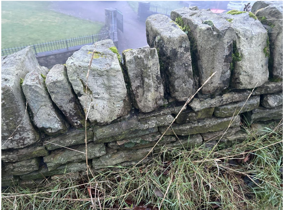
Photo B/R/13 – Wall B, Rear Face, ~CH 16.5m (Upper Parapet)
