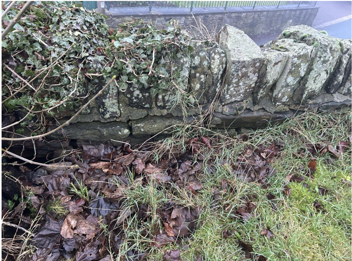
Photo B/R/1 – Wall B, Rear Face, ~CH 8.5m (Upper Parapet)
