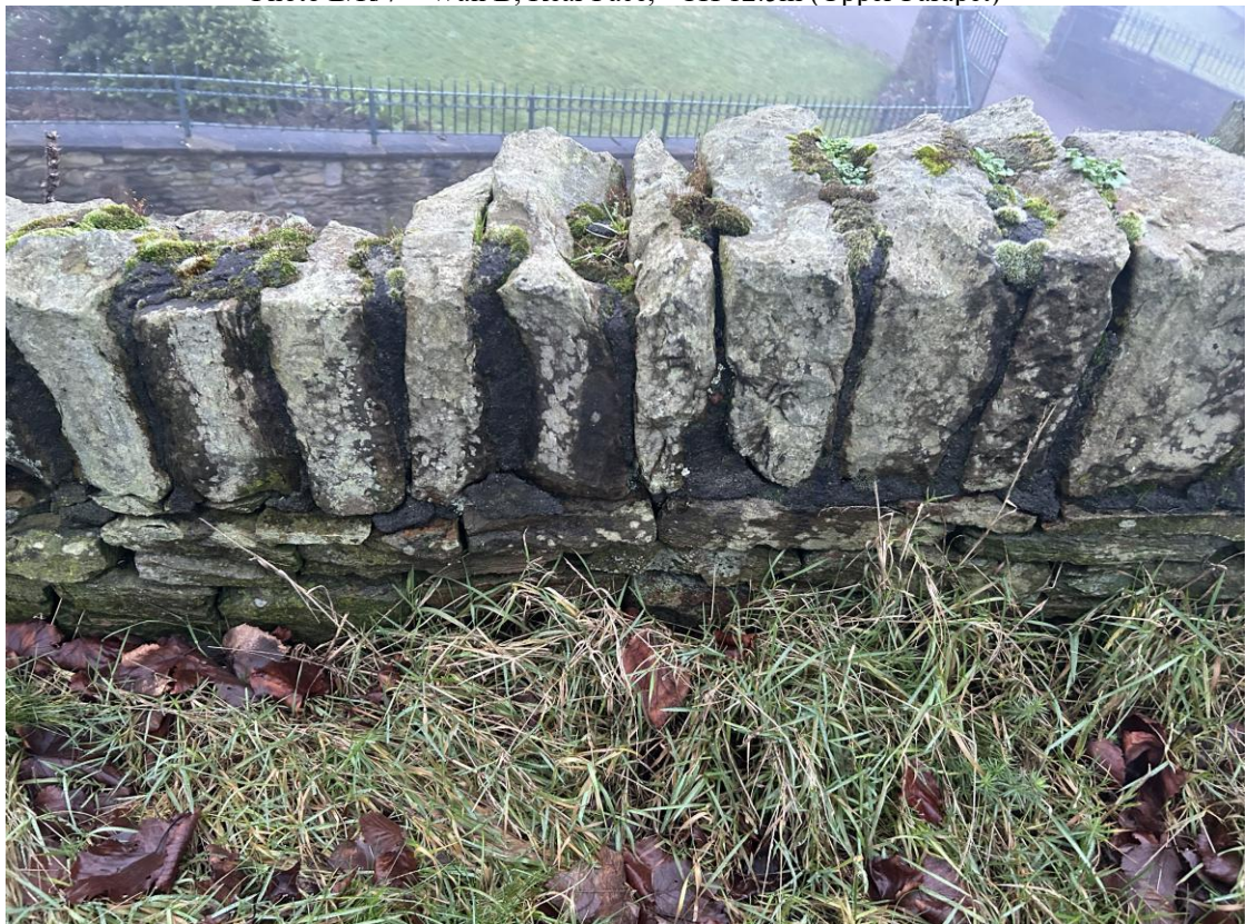
Photo B/R/8 – Wall B, Rear Face, ~CH 13.2m (Upper Parapet)
