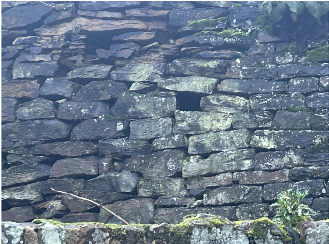
Photo B/F/10M – Wall B, Front Face, ~CH 19.0m (Middle Section)
