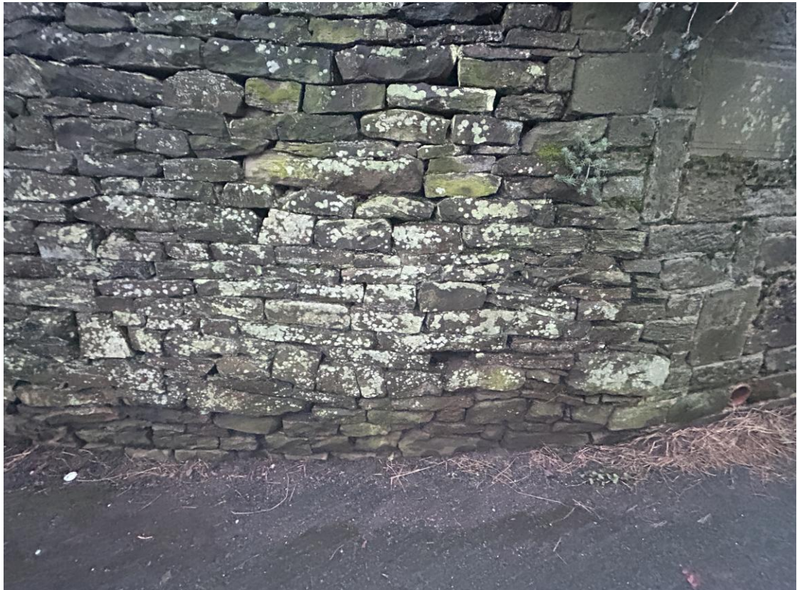
Photo B/F/3B – Wall B, Front Face, ~CH 7.5m (Lower Section)
