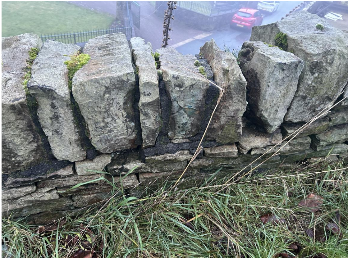
Photo B/R/11 – Wall B, Rear Face, ~CH 15.2m (Upper Parapet)
