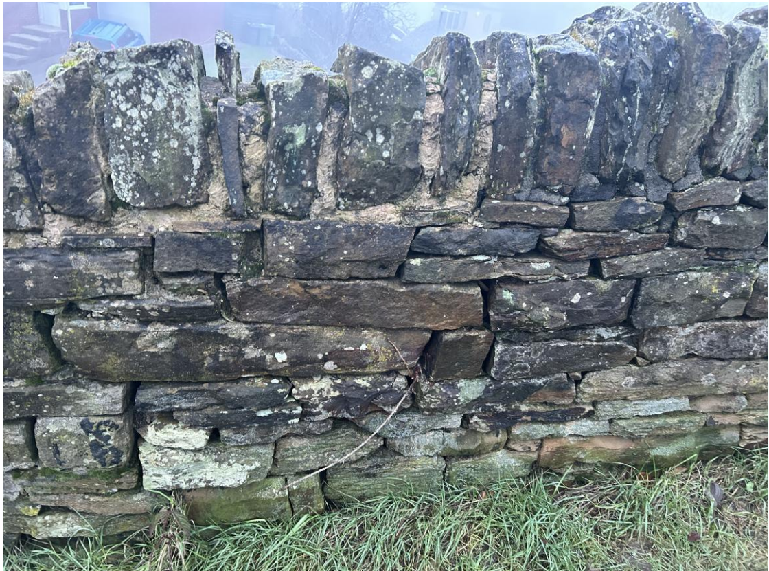
Photo B/R/23 – Wall B, Rear Face, ~CH 23.2m (Upper Parapet)
