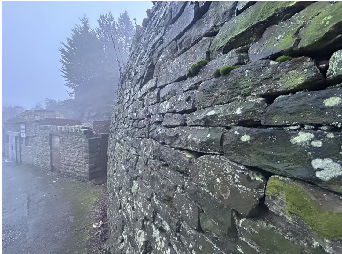
Photo B/F/2T – Wall B, Front Face, ~CH 7.0m (Upper Section)
