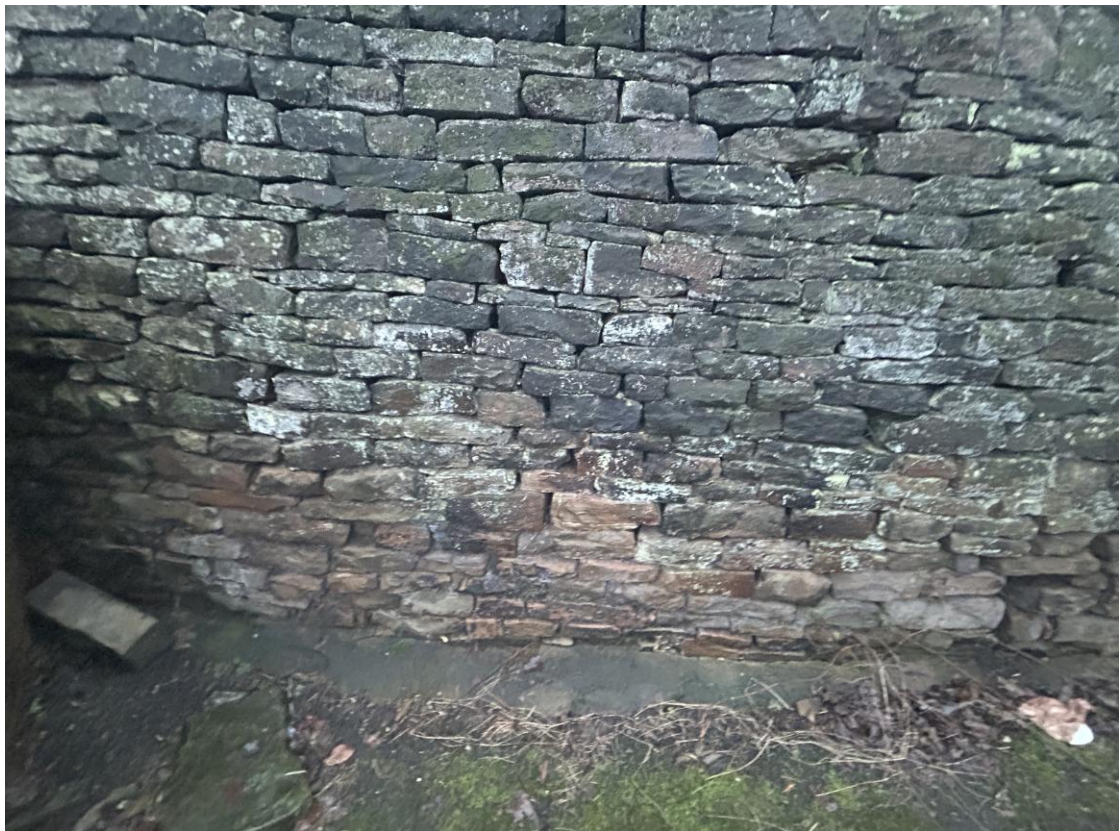
Photo B/F/8L – Wall B, Front Face, ~CH 13.2m (Lower Section)
