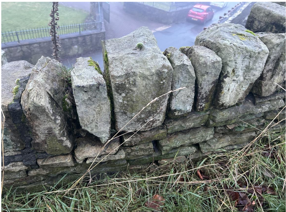
Photo B/R/12 – Wall B, Rear Face, ~CH 15.8m (Upper Parapet)
