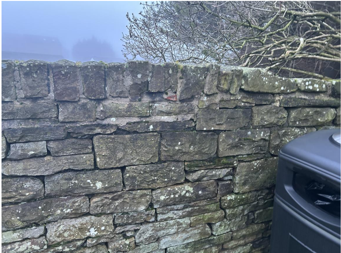
Photo B/R/26T – Wall B, Rear Face, ~CH 25.8m (Upper Parapet – Top Section)
