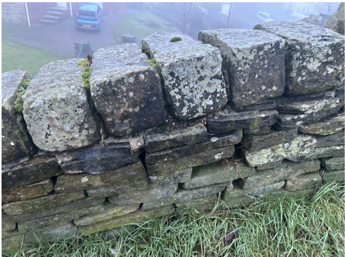
Photo B/R/18 – Wall B, Rear Face, ~CH 19.8m (Upper Parapet)
