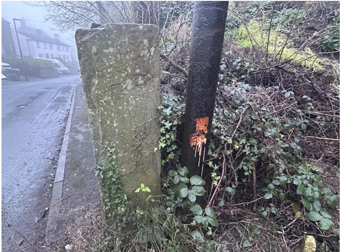
Photo A/F/1 – Wall A, Side Face, CH 0.0m (Whole Section)
