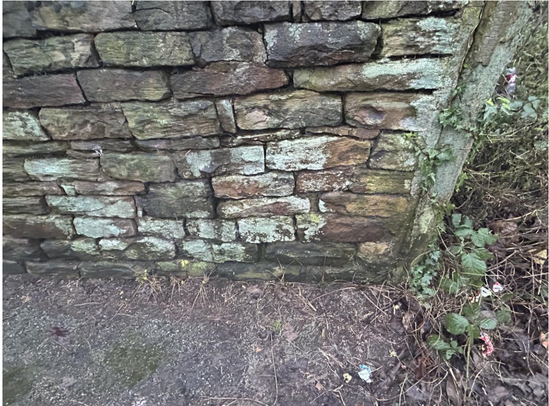
Photo C/F/2B – Wall A, Front Face, CH 0.0m (Lower Section)
