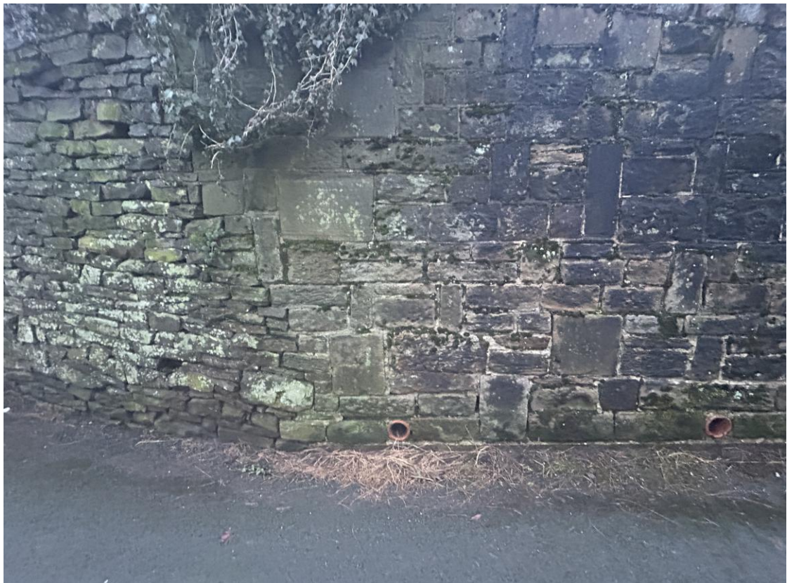
Photo B/F/1B – Wall B, Front Face, ~CH 5.5m (Lower Section)
