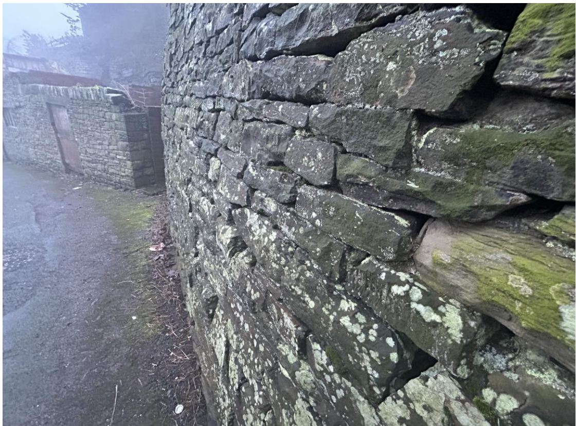
Photo B/F/2B – Wall B, Front Face, ~CH 7.0m (Lower Section)
