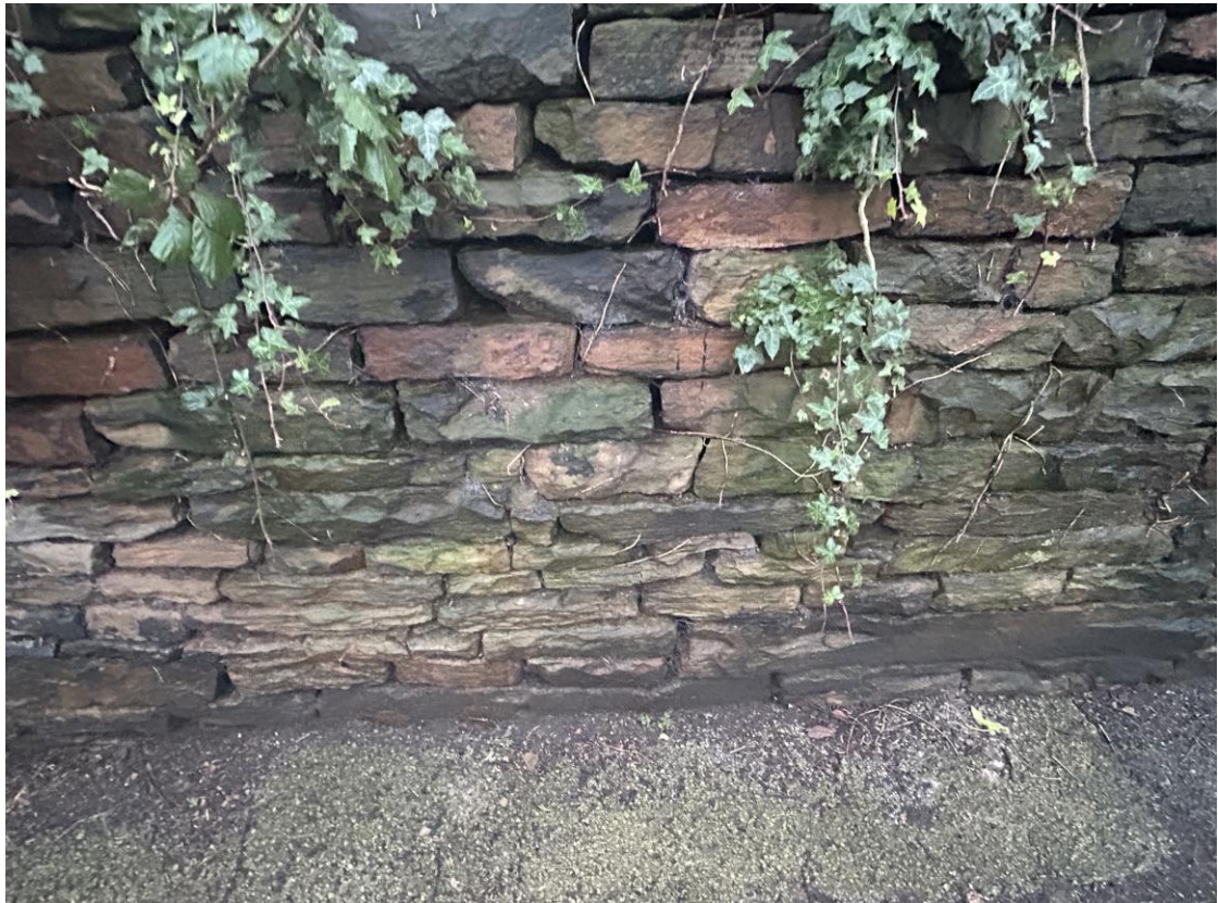
Photo K/F/6B – Wall A, Front Face, ~CH 4.0m (Lower Section)
