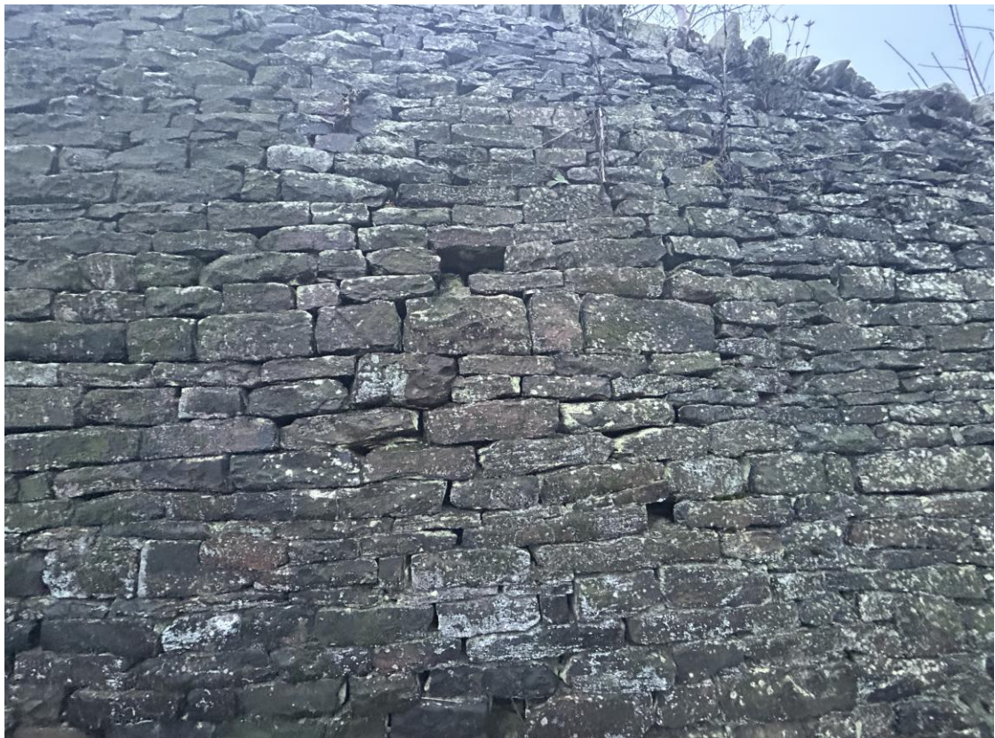
Photo B/F/7M – Wall B, Front Face, ~CH 12.5m (Middle Section)
