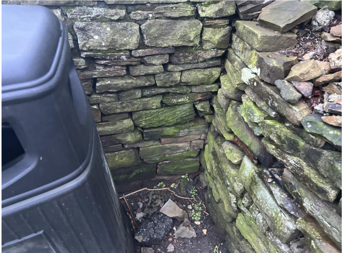
Photo B/R/27 – Wall B, Rear Face, ~CH 27.0m (Upper Parapet – Lower Section)
