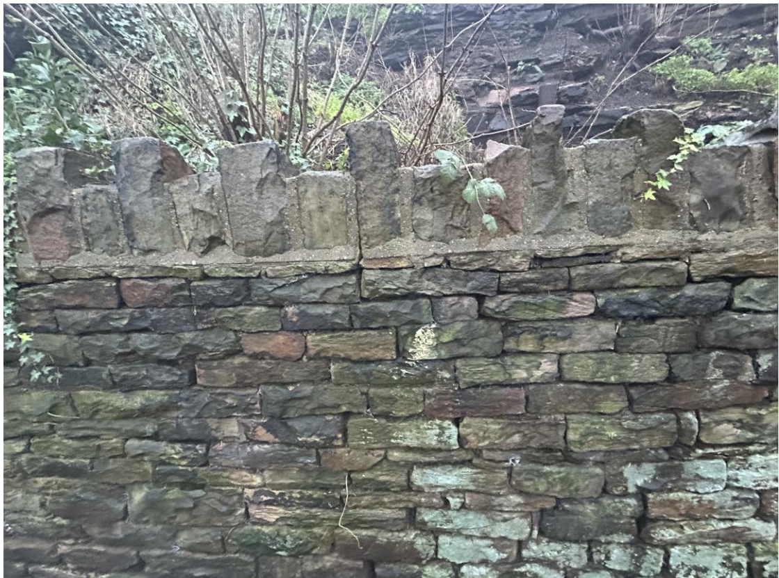
Photo D/F/3T – Wall A, Front Face, ~CH 1.0m (Upper Section)
