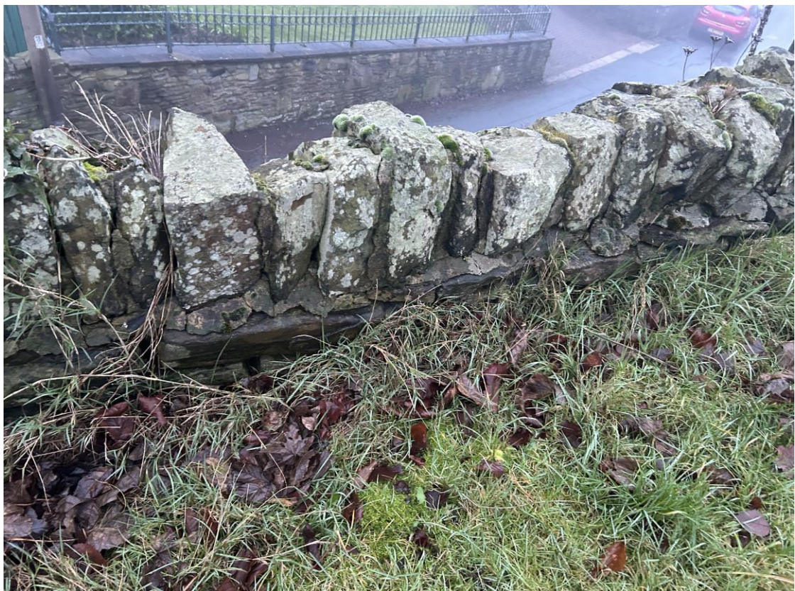
Photo B/R/2 – Wall B, Rear Face, ~CH 9.2m (Upper Parapet)
