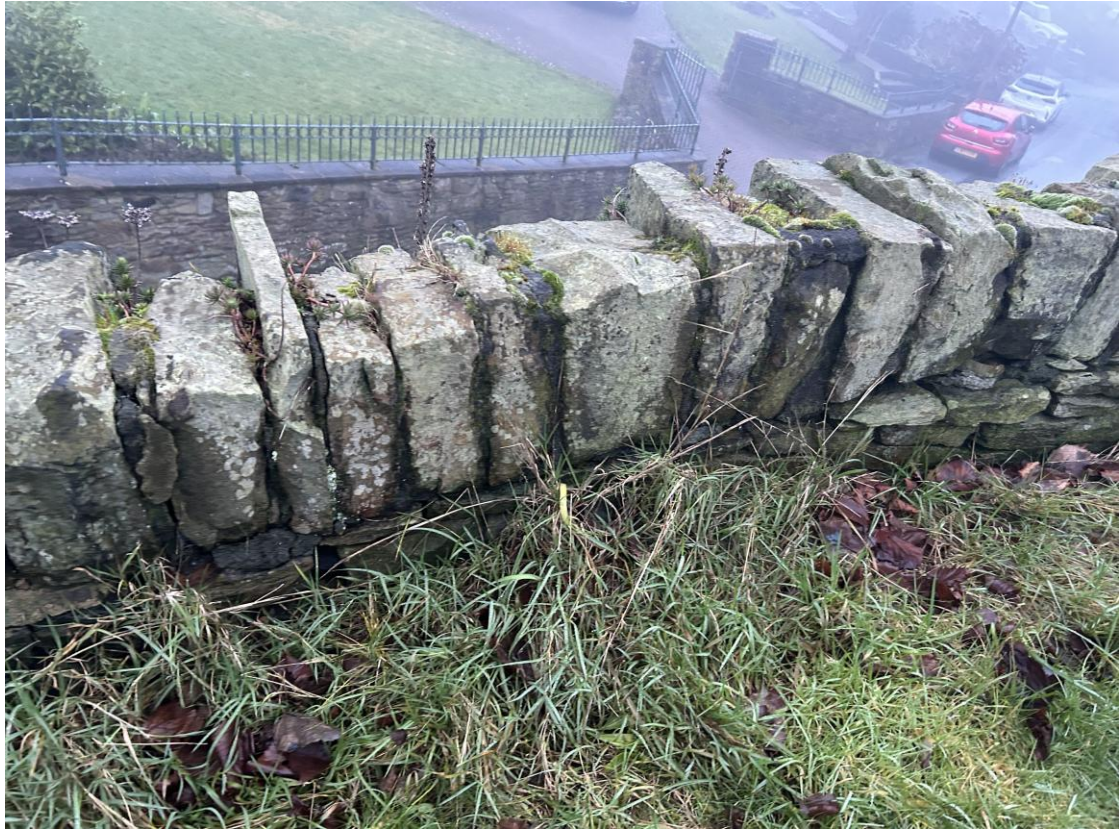
Photo B/R/5 – Wall B, Rear Face, ~CH 11.2m (Upper Parapet)
