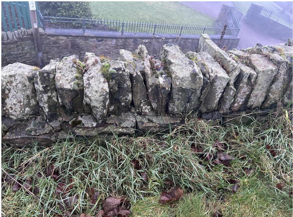
Photo B/R/4 – Wall B, Rear Face, ~CH 10.5m (Upper Parapet)
