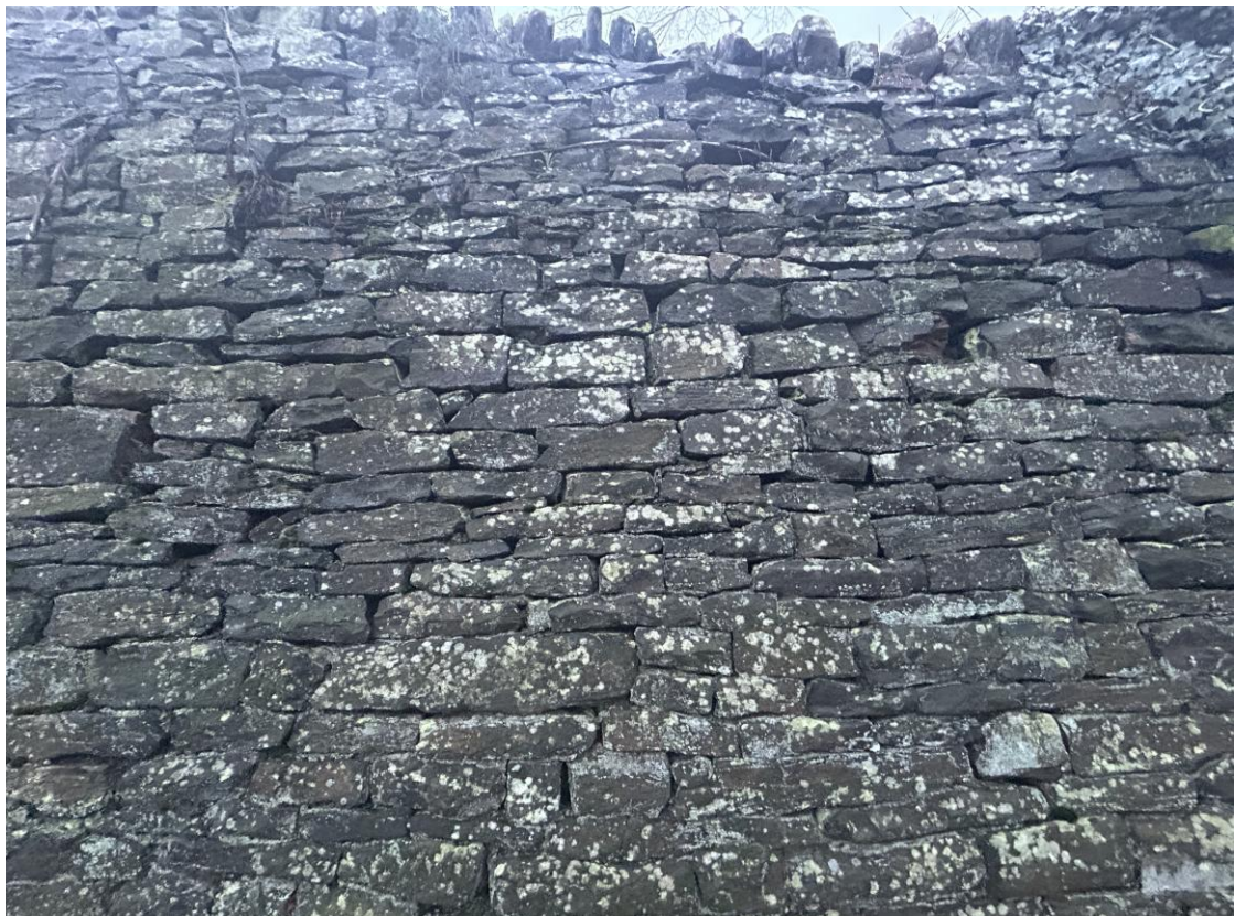
Photo B/F/5M – Wall B, Front Face, ~CH 10.2m (Middle Section)
