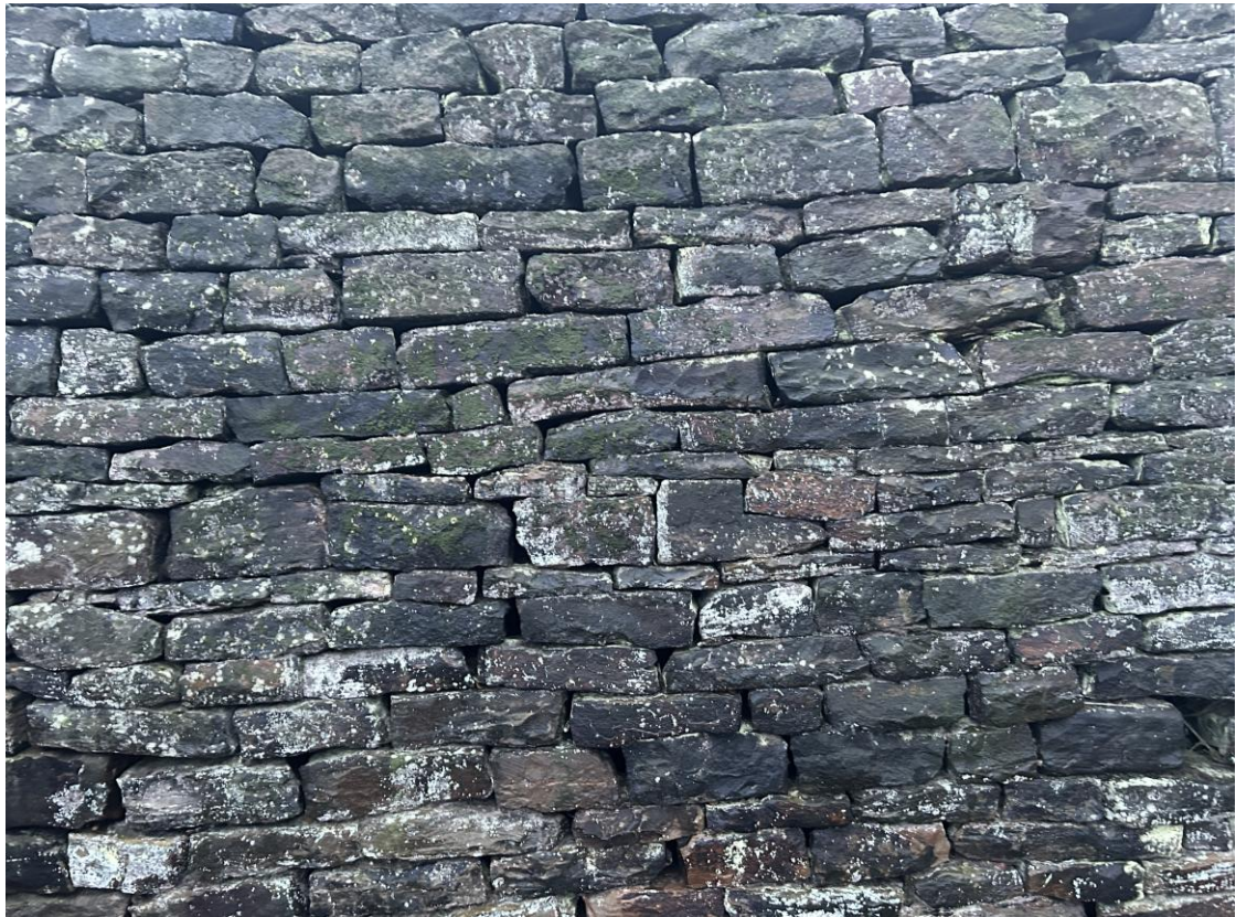
Photo B/F/8M – Wall B, Front Face, ~CH 13.2m (Middle Section)
