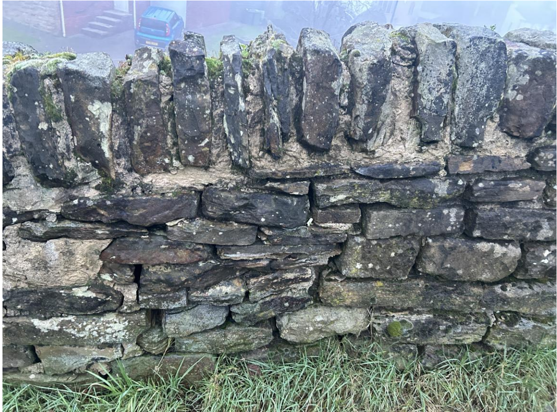
Photo B/R/21 – Wall B, Rear Face, ~CH 21.8m (Upper Parapet)
