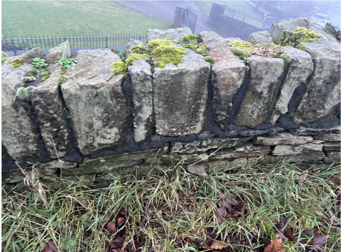
Photo B/R/9 – Wall B, Rear Face, ~CH 13.8m (Upper Parapet)
