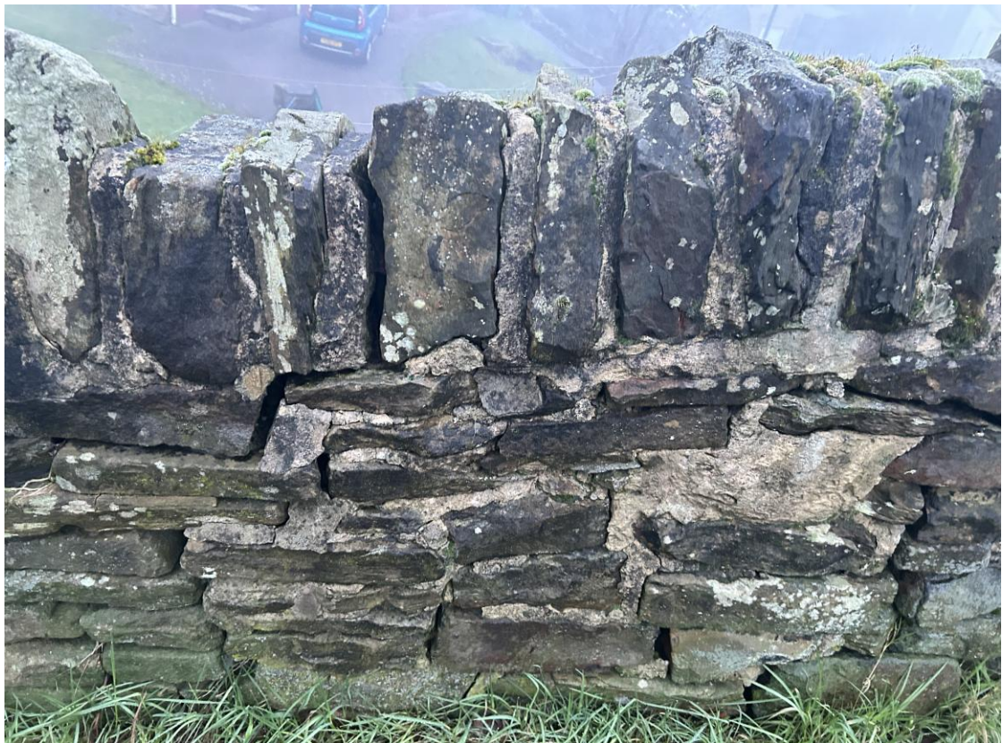
Photo B/R/20 – Wall B, Rear Face, ~CH 21.2m (Upper Parapet)
