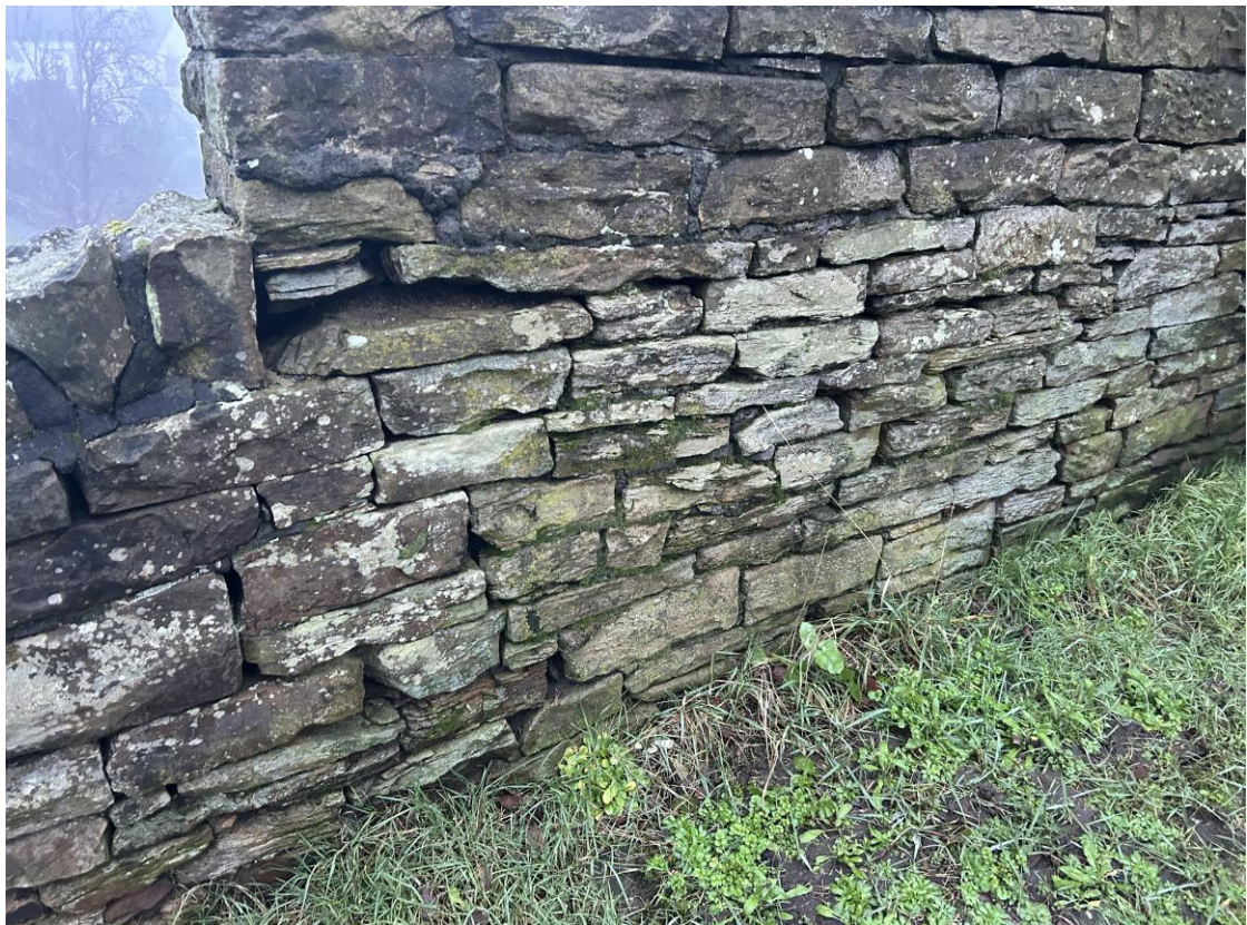
Photo B/R/25B – Wall B, Rear Face, ~CH 24.5m (Upper Parapet – Lower Section)
