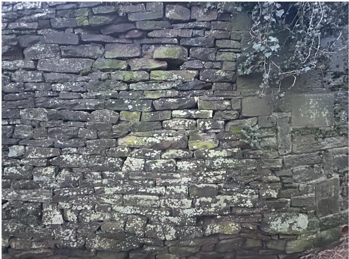
Photo B/F/3M – Wall B, Front Face, ~CH 7.5m (Middle Section)
