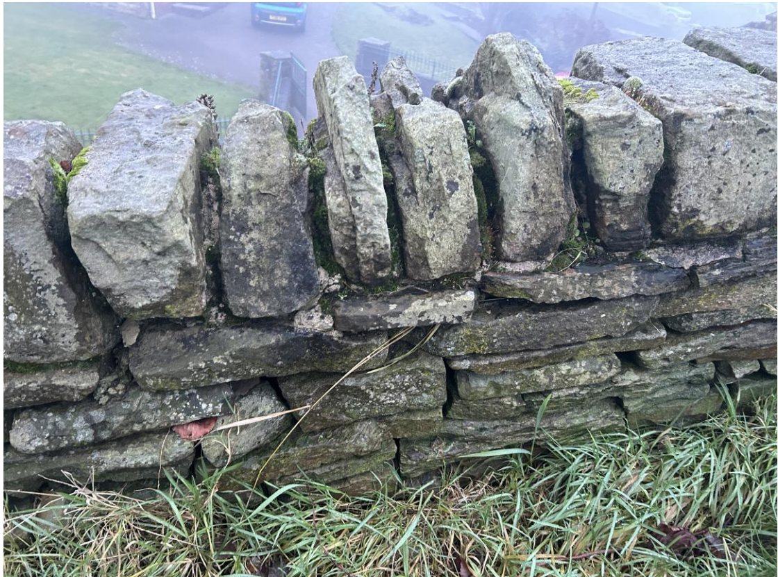
Photo B/R/15 – Wall B, Rear Face, ~CH 17.8m (Upper Parapet)
