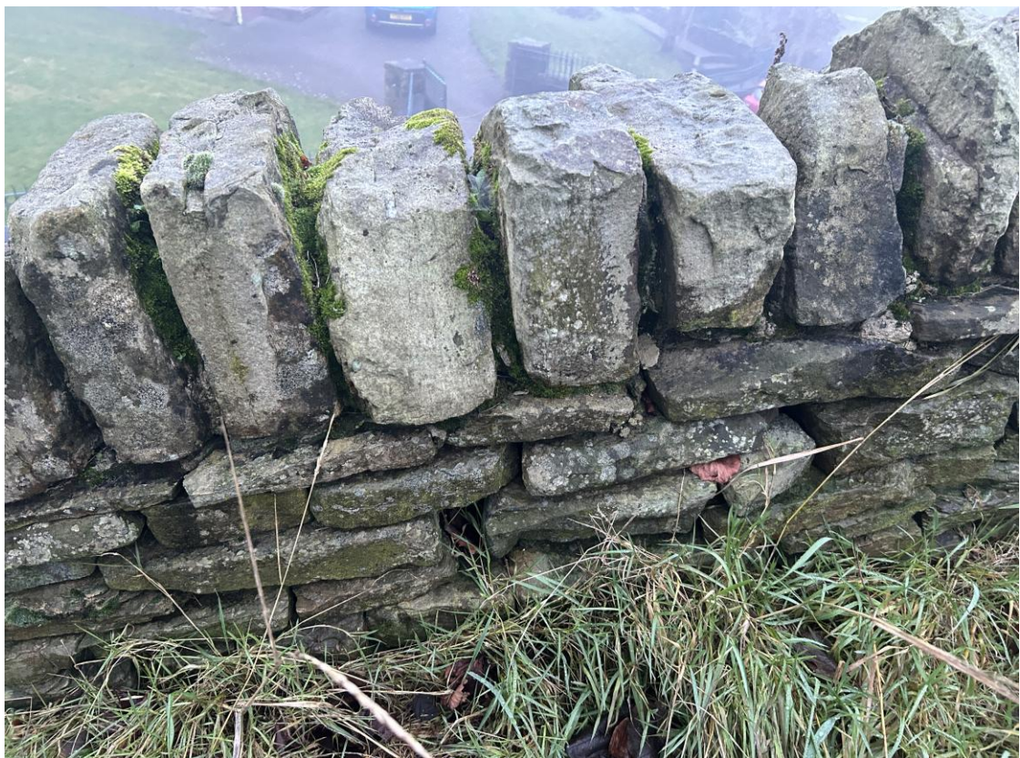
Photo B/R/14 – Wall B, Rear Face, ~CH 17.2m (Upper Parapet)
