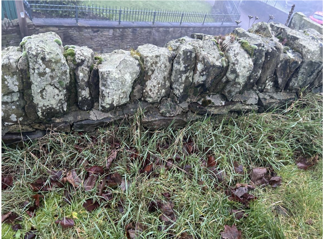
Photo B/R/3 – Wall B, Rear Face, ~CH 9.8m (Upper Parapet)
