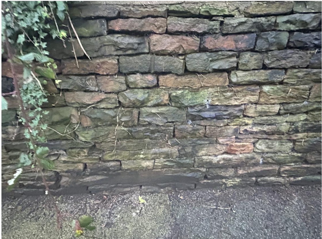
Photo I/F/5B – Wall A, Front Face, ~CH 3.0m (Lower Section)
