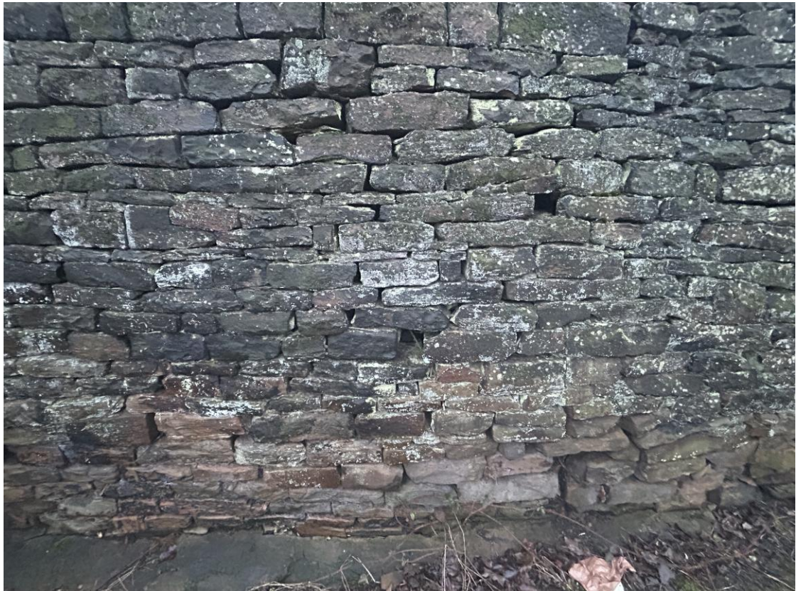
Photo B/F/7L – Wall B, Front Face, ~CH 12.5m (Lower Section)
