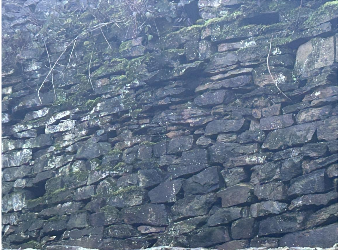
Photo B/F/11M – Wall B, Front Face, ~CH 21.5m (Middle Section)
