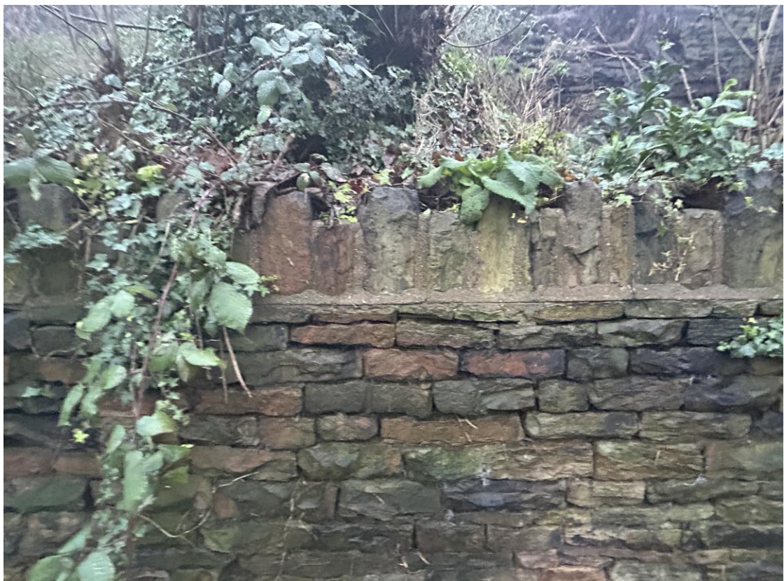
Photo H/F/5T – Wall A, Front Face, ~CH 3.0m (Upper Section)
