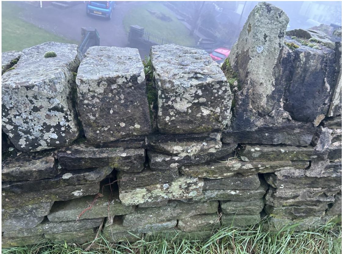
Photo B/R/19 – Wall B, Rear Face, ~CH 20.5m (Upper Parapet)
