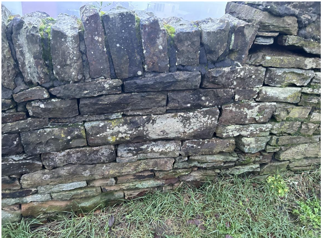
Photo B/R/24 – Wall B, Rear Face, ~CH 23.8m (Upper Parapet)
