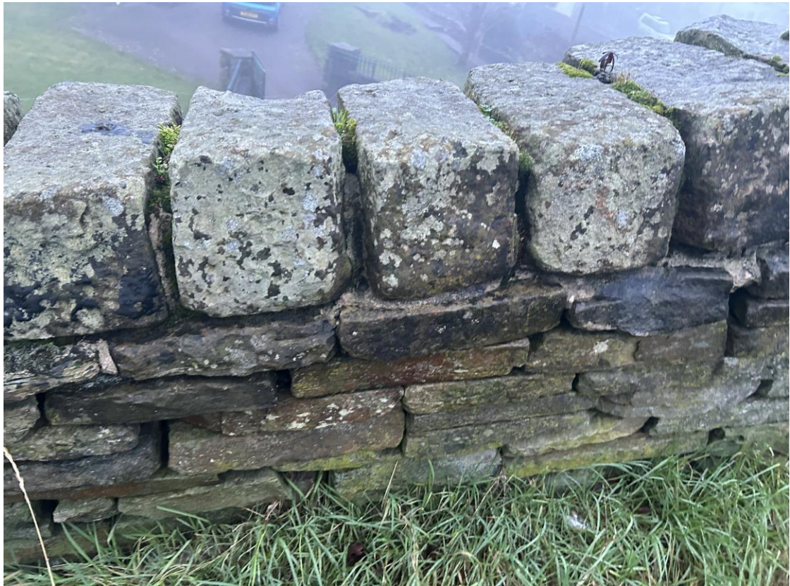
Photo B/R/17 – Wall B, Rear Face, ~CH 19.2m (Upper Parapet)
