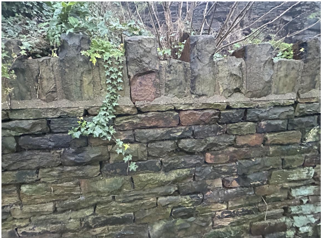
Photo F/F/4T – Wall A, Front Face, ~CH 2.0m (Upper Section)
