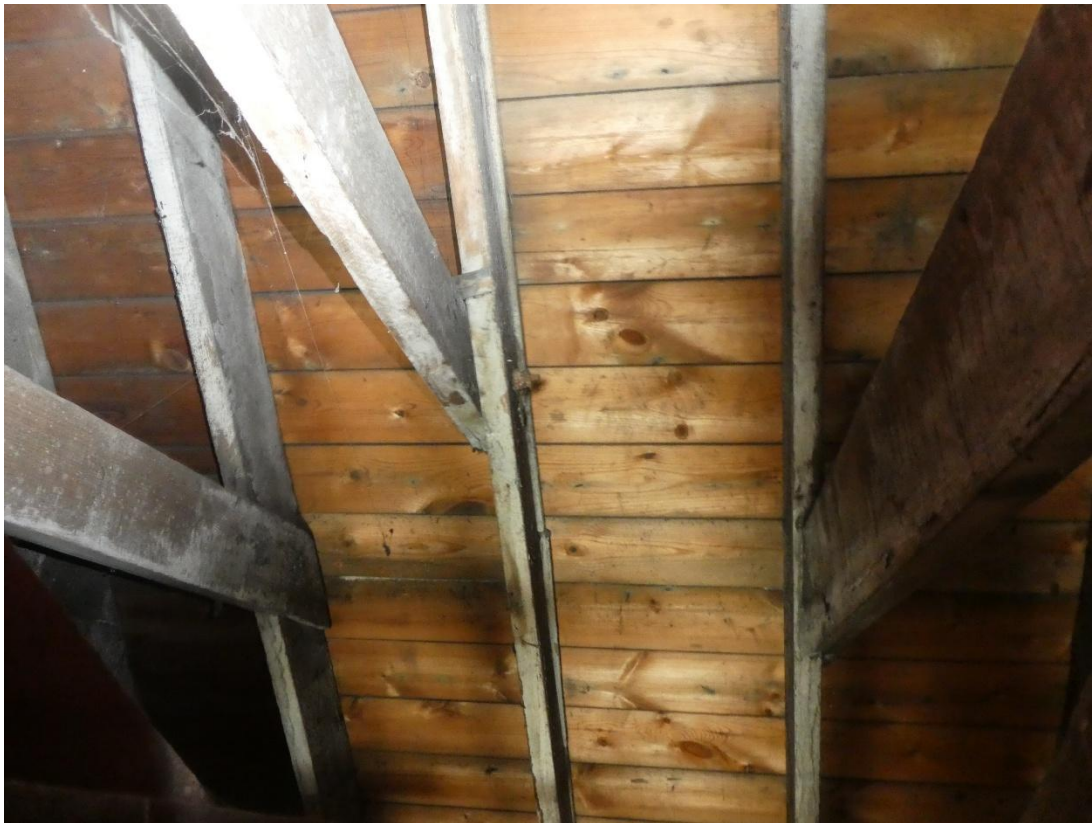
Scissor trusses with horizontal boarding 1890's front section.
