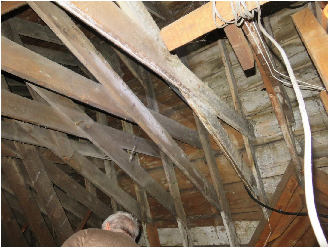
Scissor trusses (1890's).
