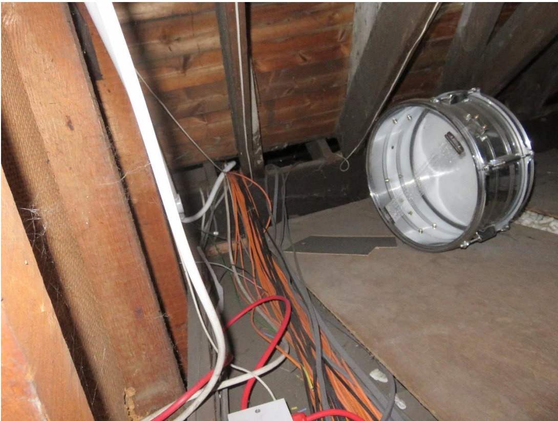
Scissor trusses (1890's).
