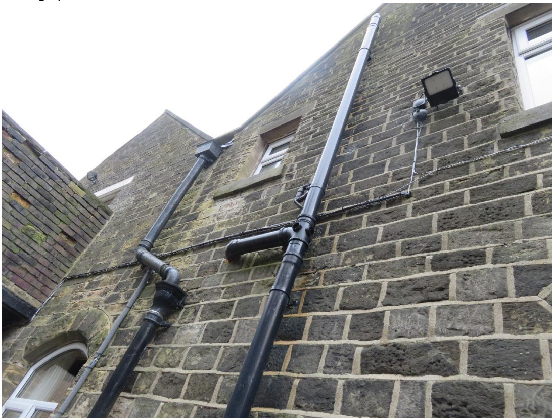
Vertical joint to right hand side elevation indicating the rear section was built at an earlier period in the first front section possibly around 1890's.
