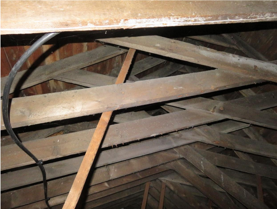
Scissor trusses (1890's).
