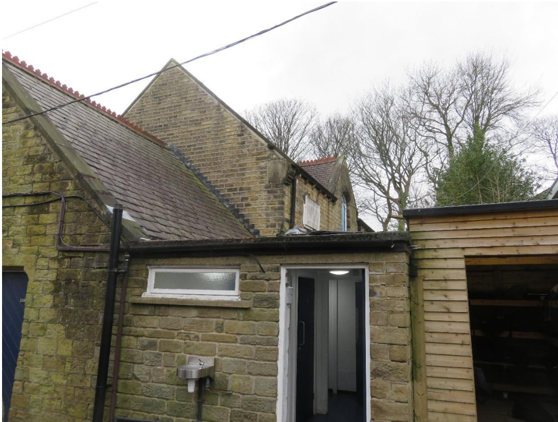
Single storey toilet block circa 1960's.
