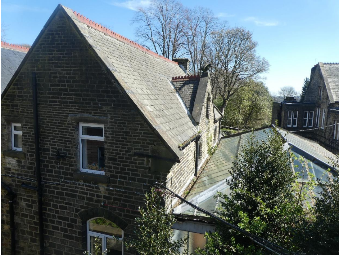
First floor window to left hand side later position, probably inserted between 1930's and 1950's.
