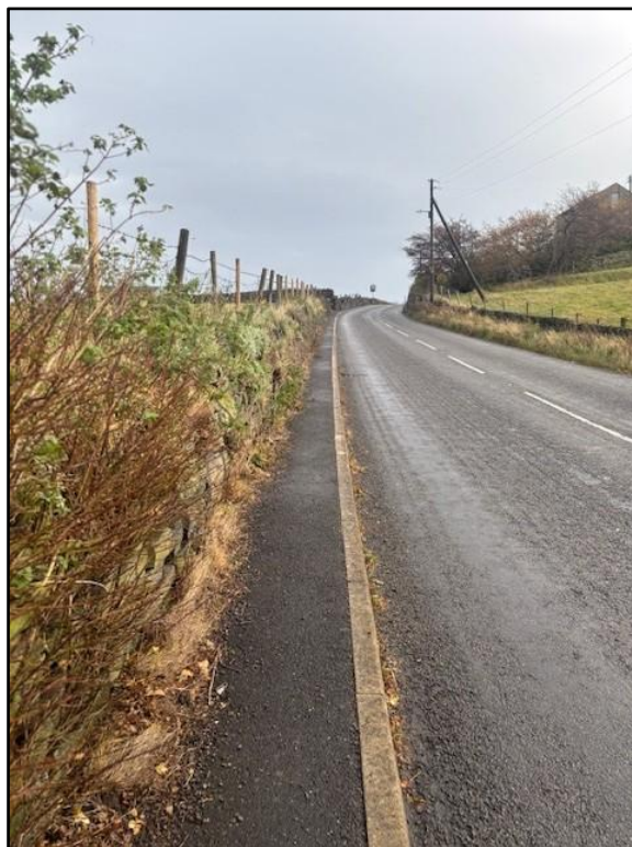
Image 1.3 Meltham Road Adjacent Site frontage
