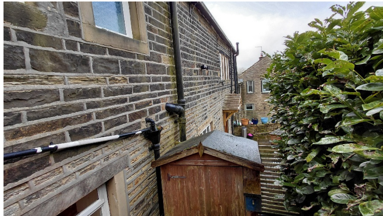
6,7 Barnside - Rear Elevation
