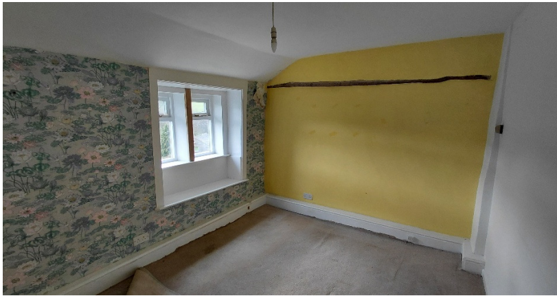
Front bedroom, sings of old beams built into the wall
