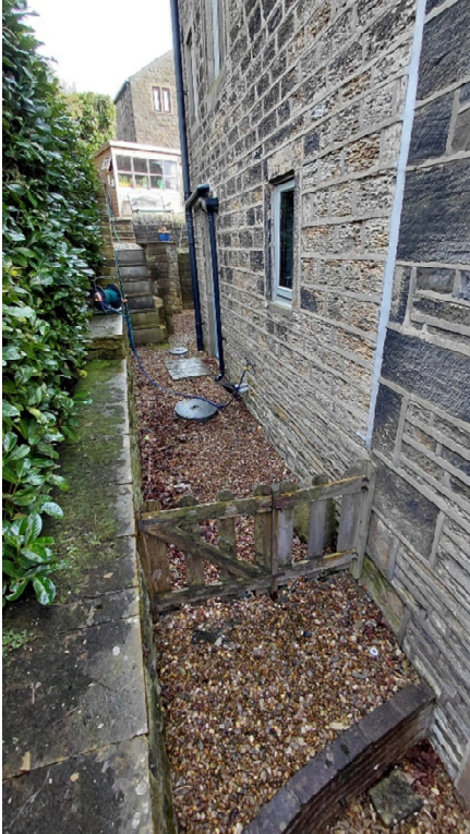
9 Barnside - Rear Elevation
